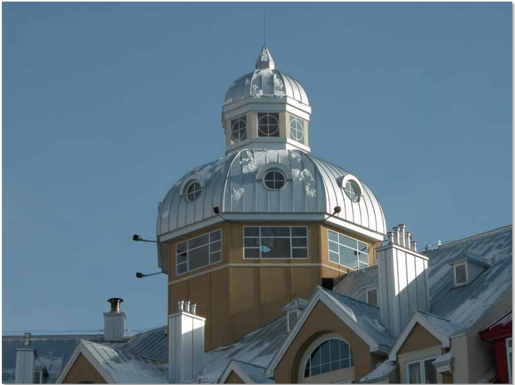
Contemporary terne-look roof in standing seam
