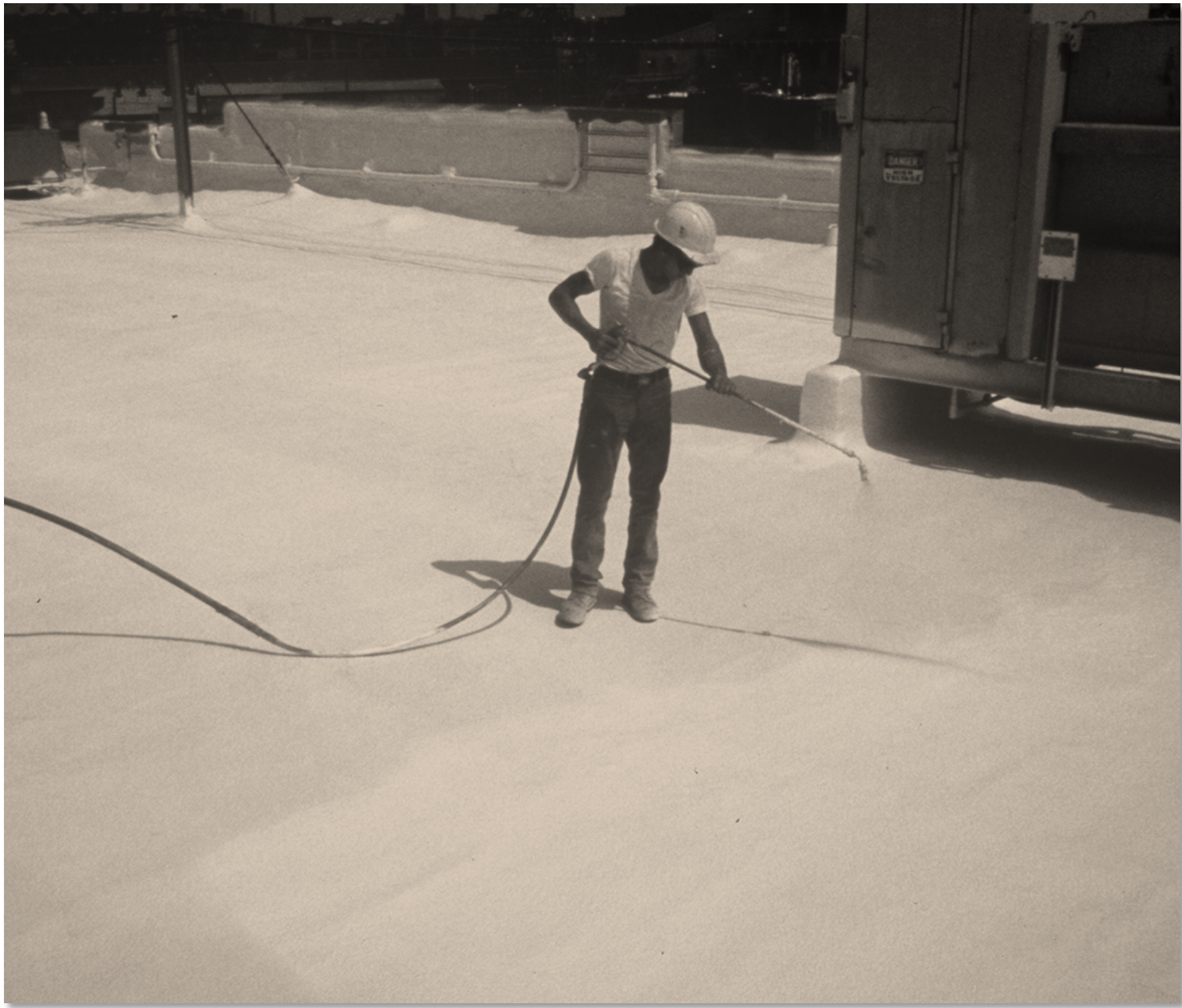
Spray applied elastomeric membrane roofing
