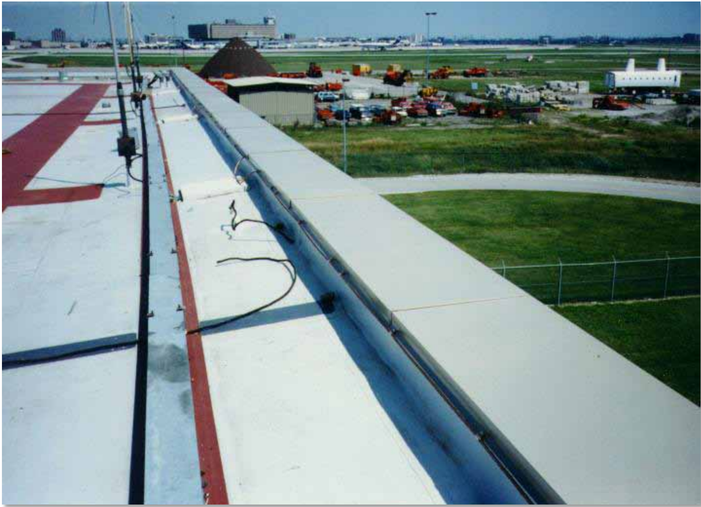
PVC Roof at Pearson International Airport
