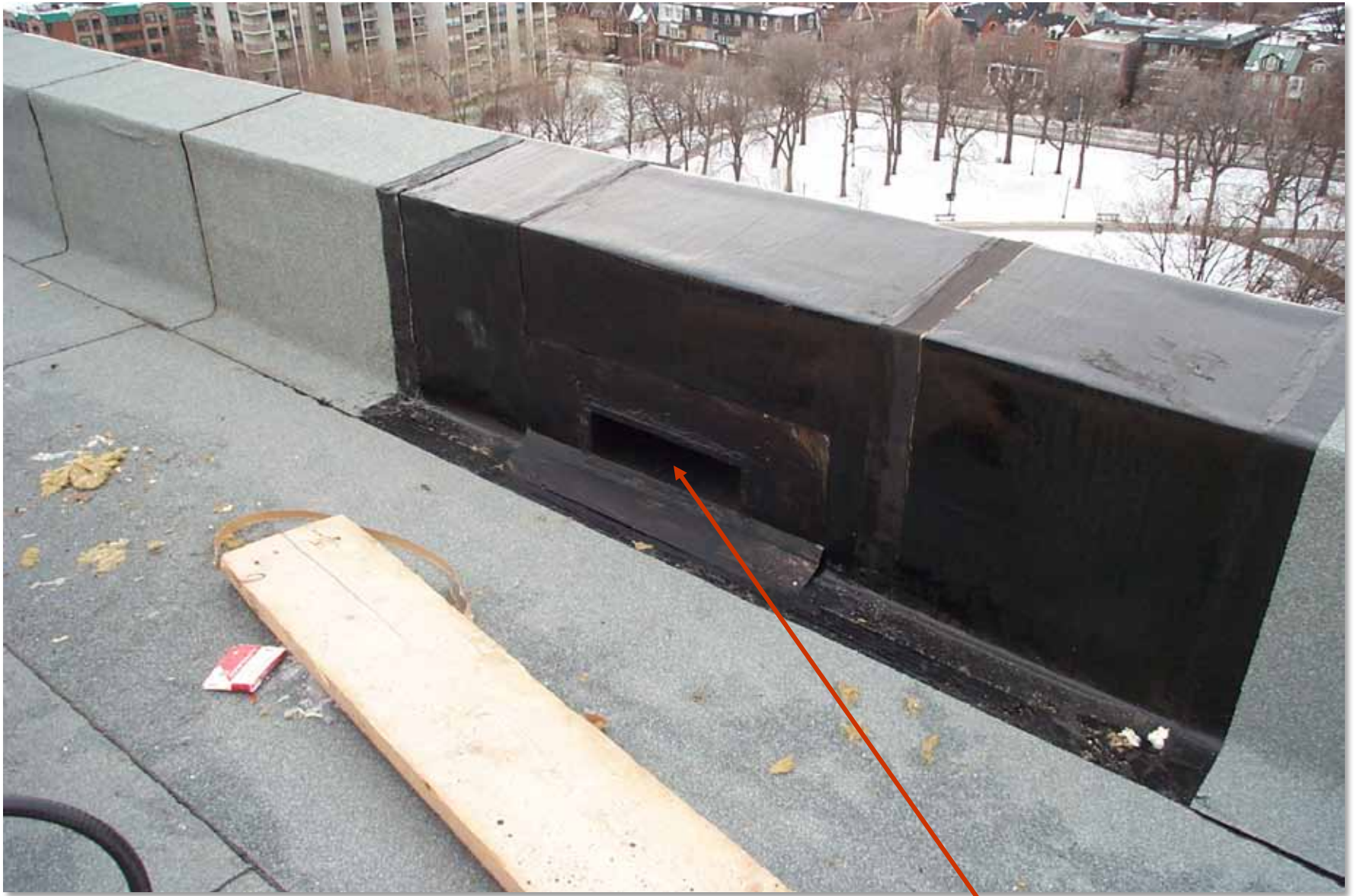
Detail at parapet. Note water overflow opening.
