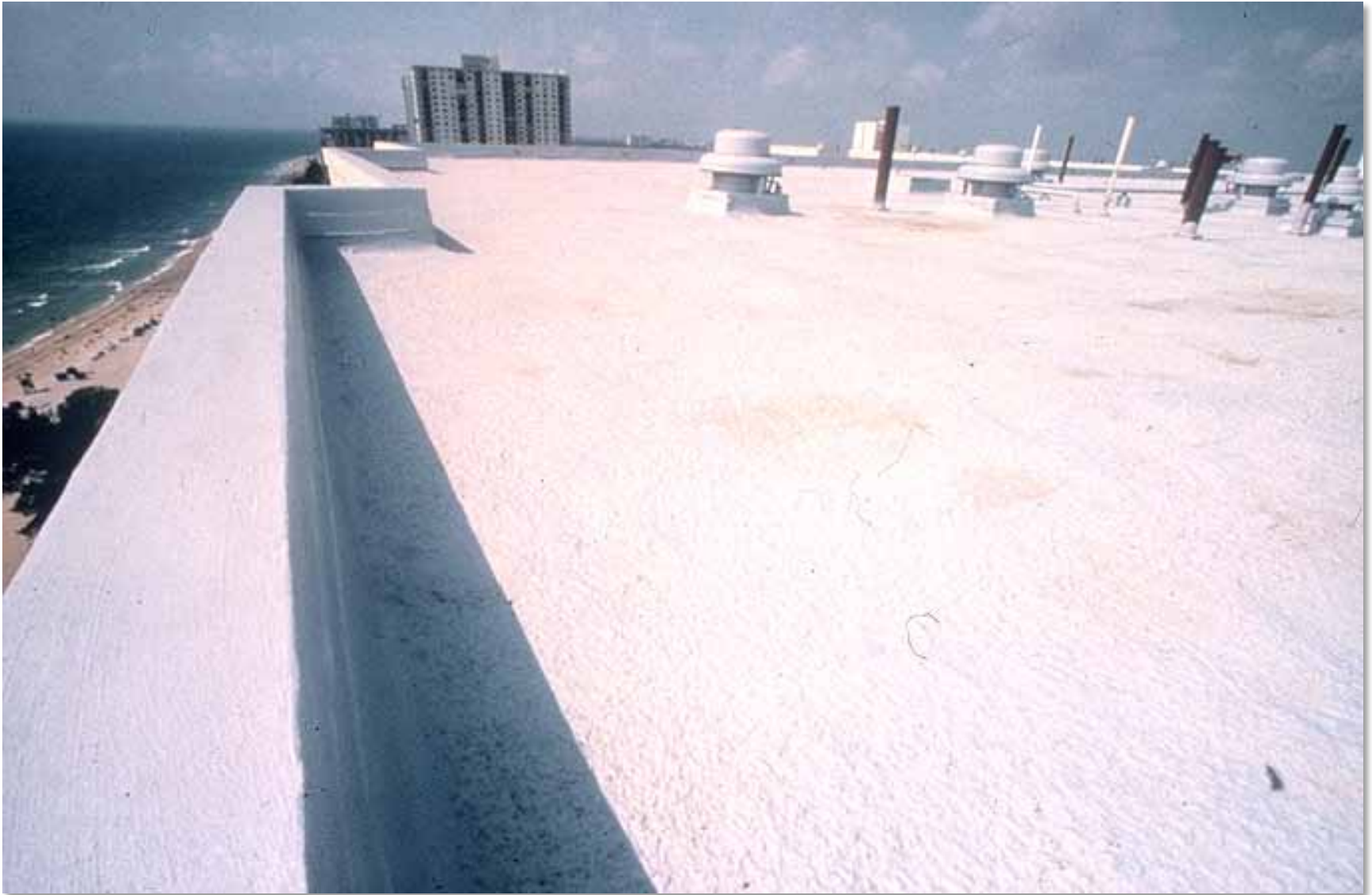
Spray applied elastomeric membrane roofing
