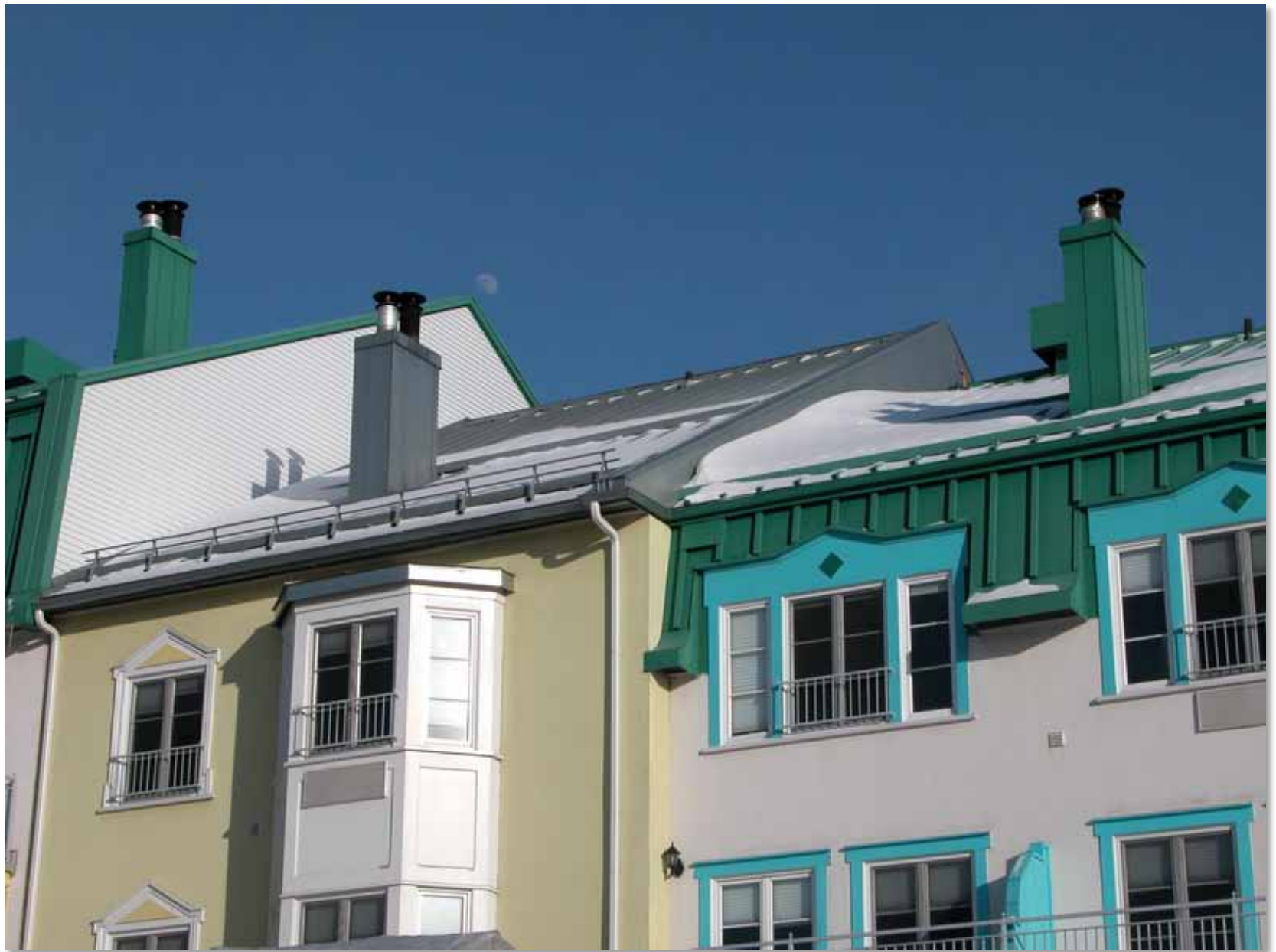
Snow guards at the edge of roofs
