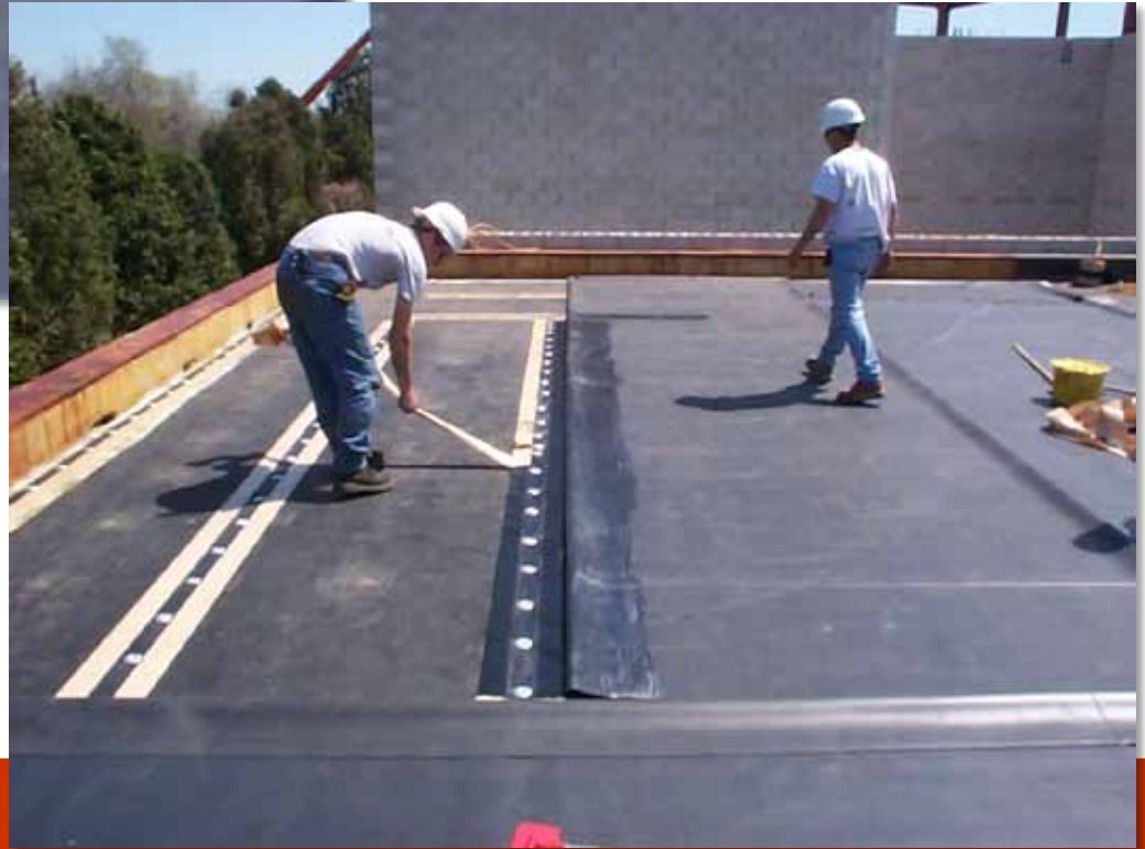
Mechanical fastening strips and an EPDM roof
