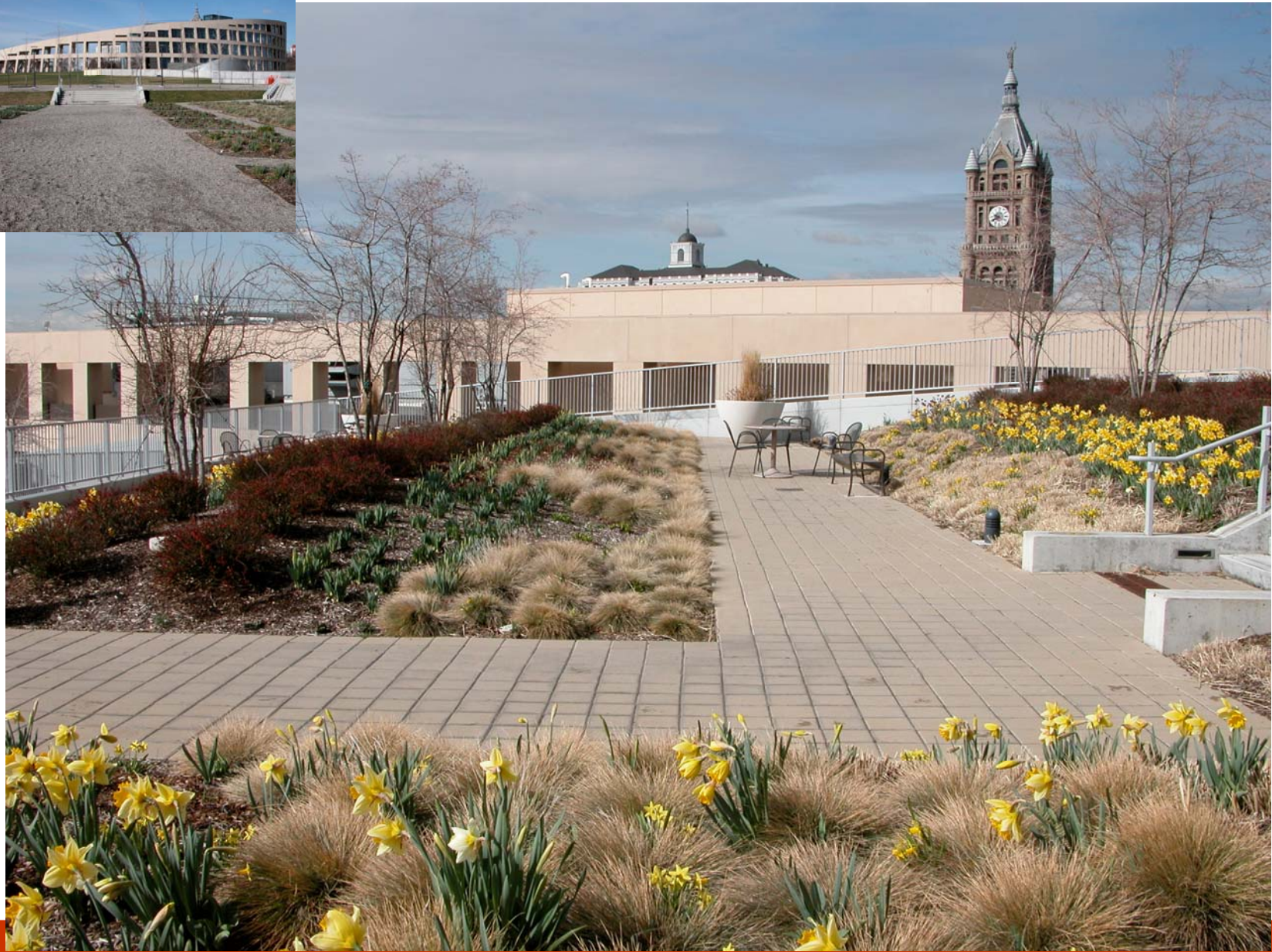
Partial green roof on the Salt Lake City Library by Moshe Safdie
