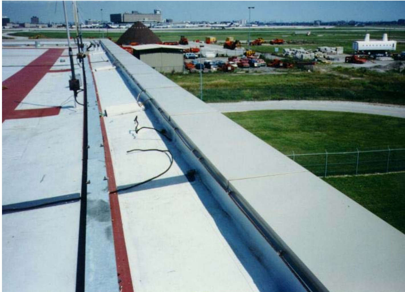
PVC Roof at Pearson International Airport
