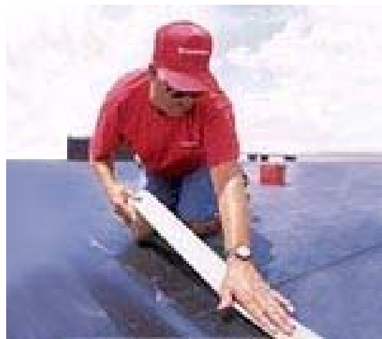
EPDM Roofing installation
