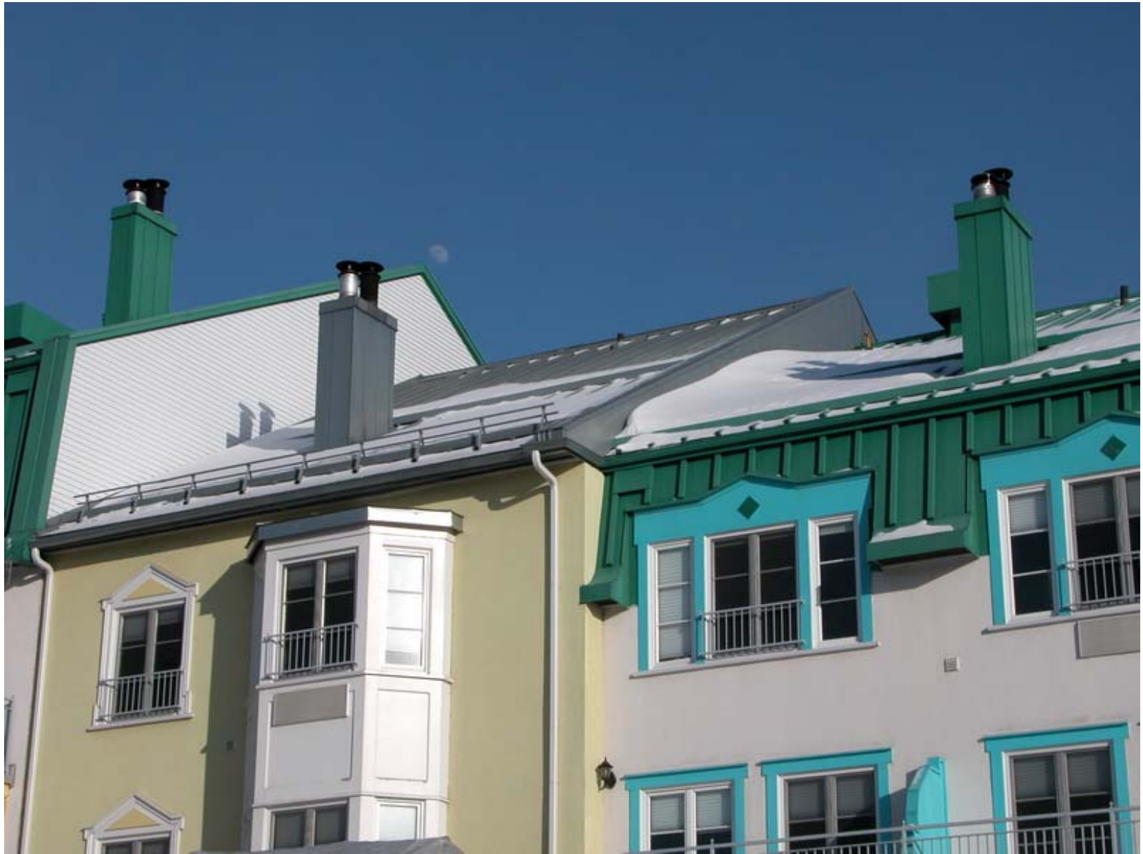
Snow guards at the edge of roofs
