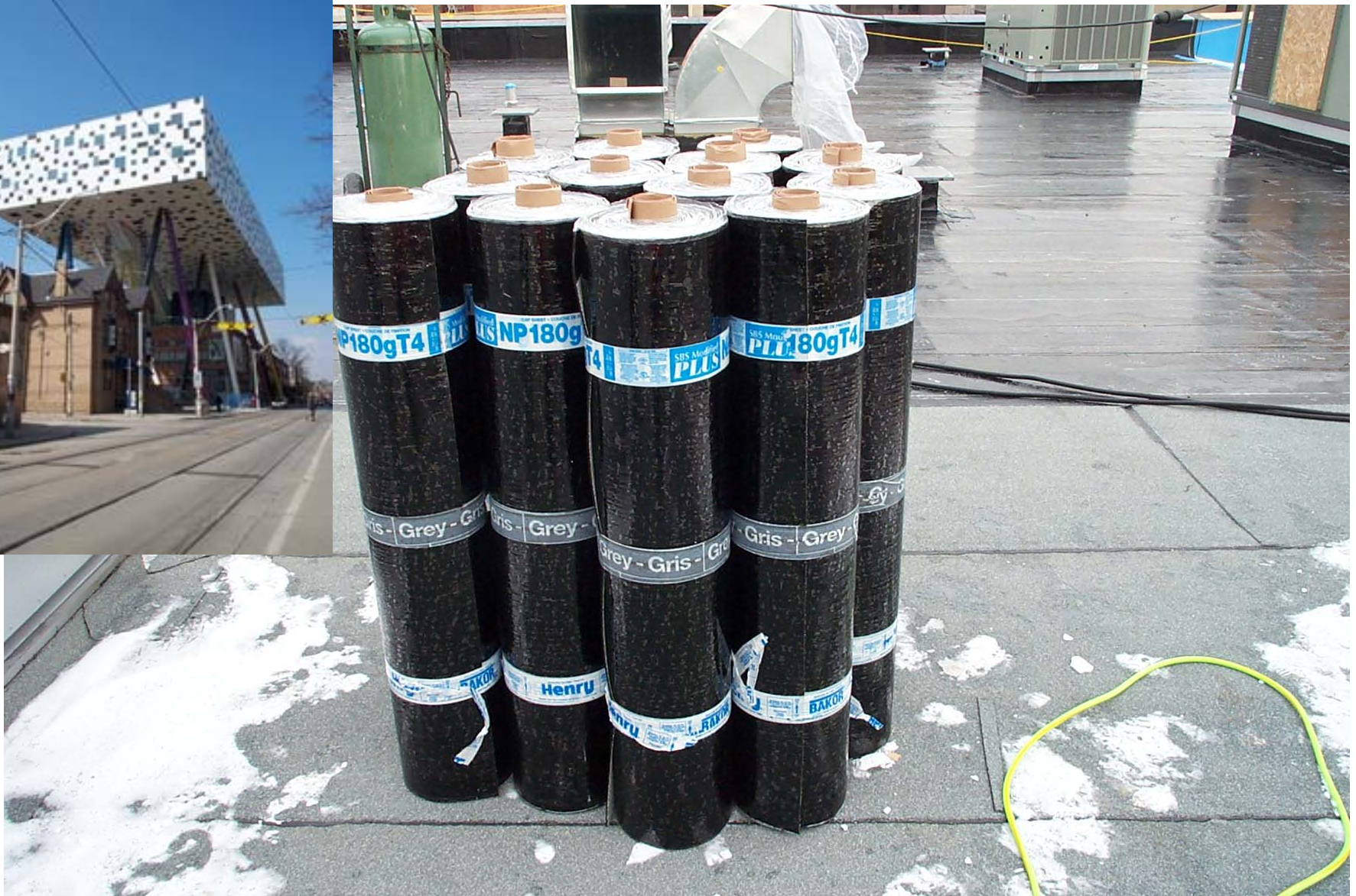
OCAD modified bitumenous membrane roofing ready for installation
