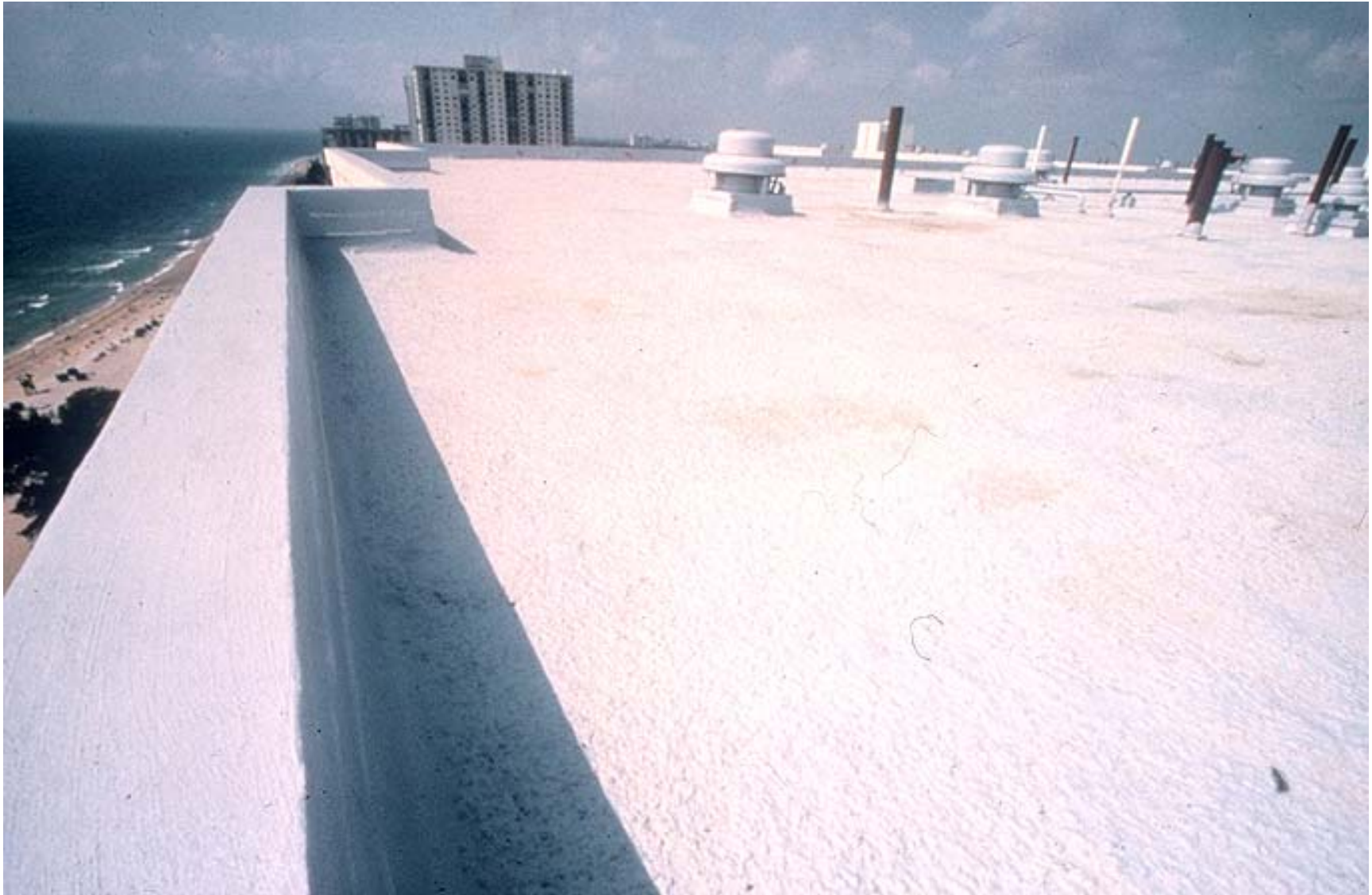
Spray applied elastomeric membrane roofing
