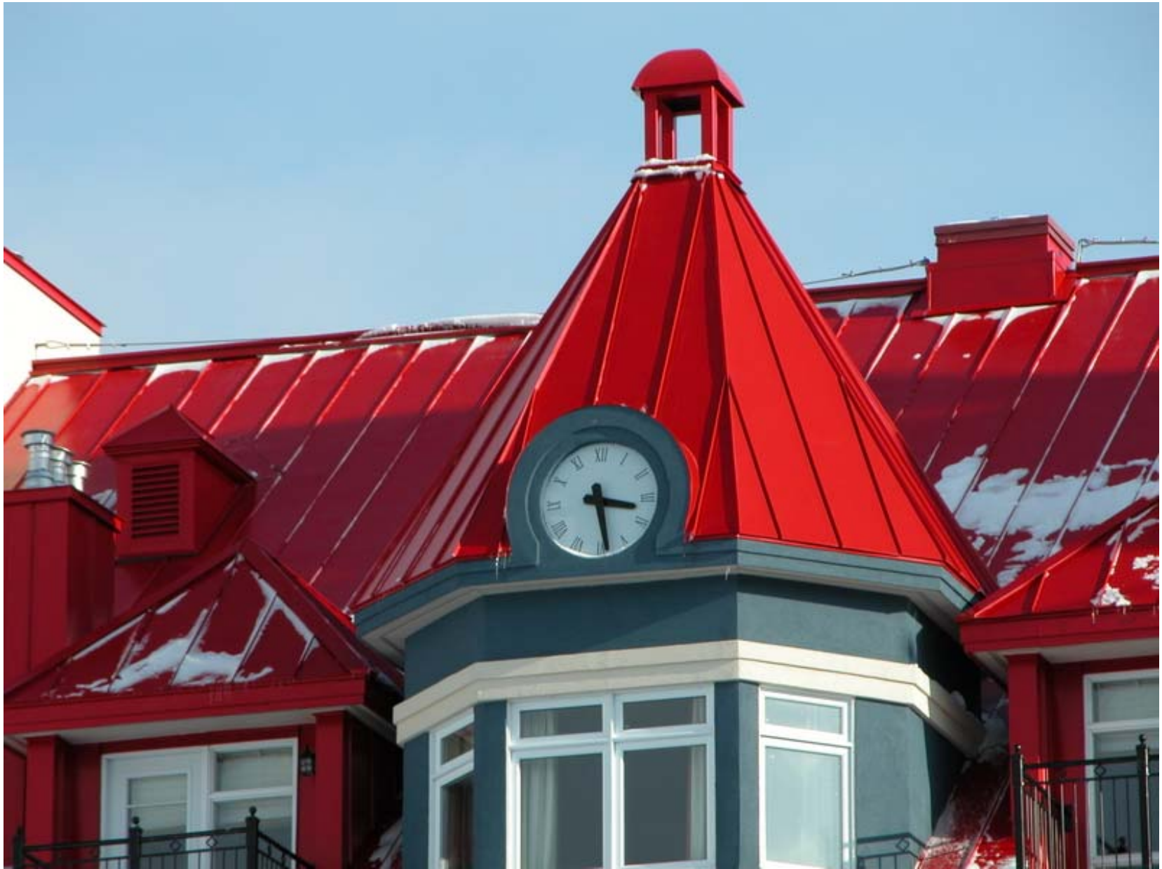
Standing seam metal roof
