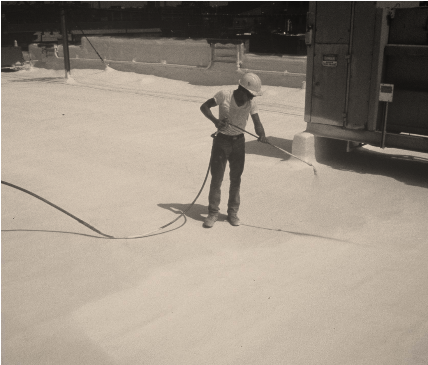
Spray applied elastomeric membrane roofing
