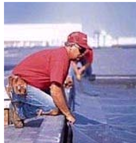
EPDM Roofing installation
