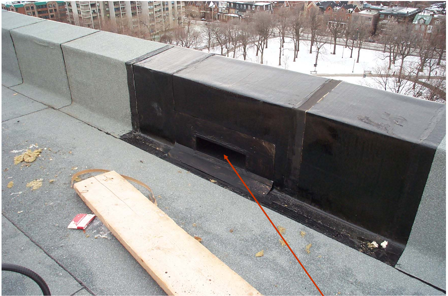
Detail at parapet. Note water overflow opening.
