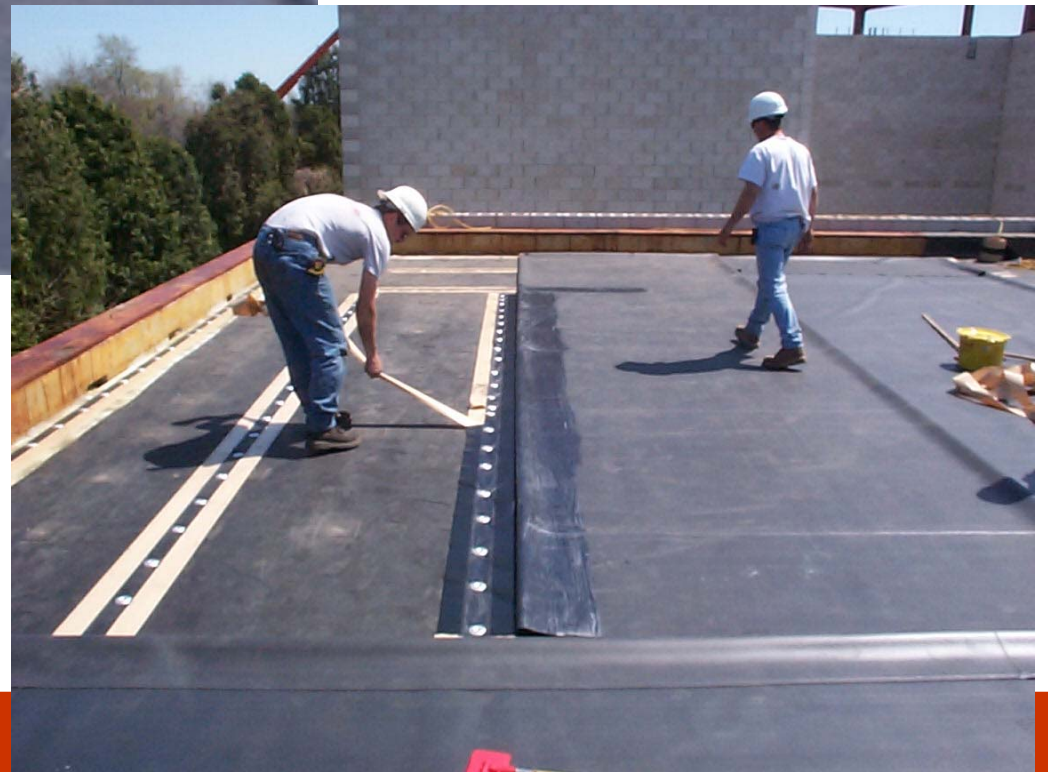
Mechanical fastening strips and an EPDM roof
