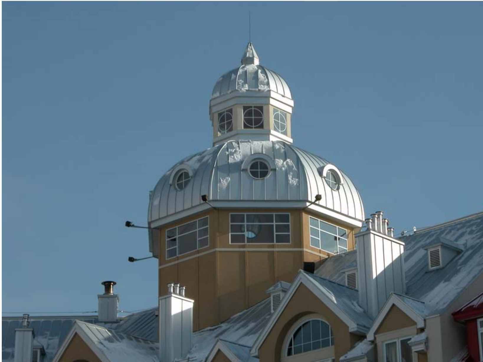
Contemporary terne-look roof in standing seam
