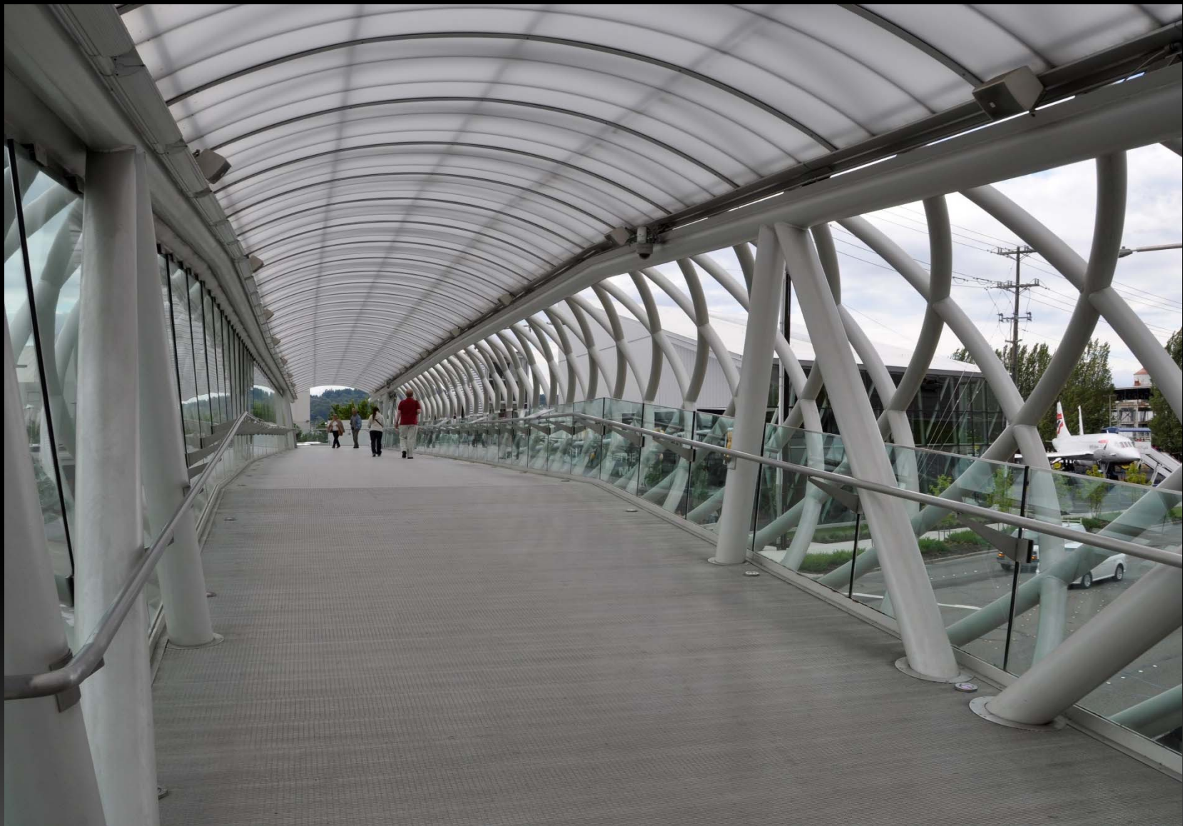
Interior view down the bridge. Slight arch as it passes over the roadway.
