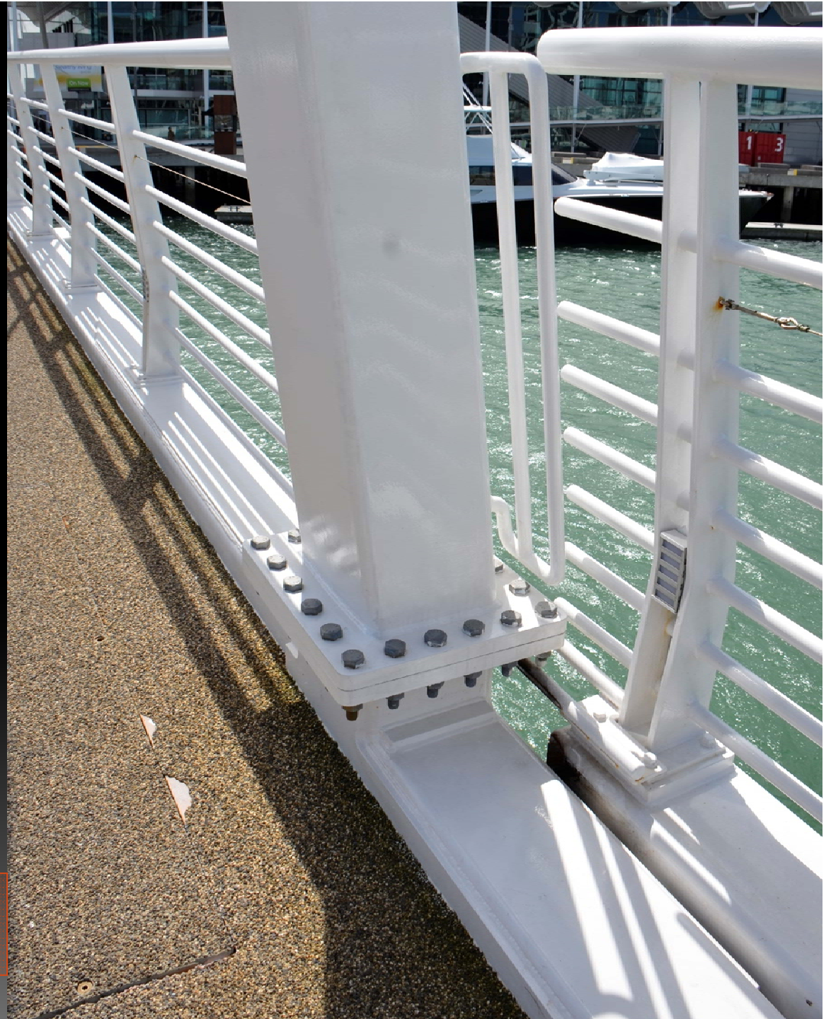
Base connection of the mast to the bridge platform.
