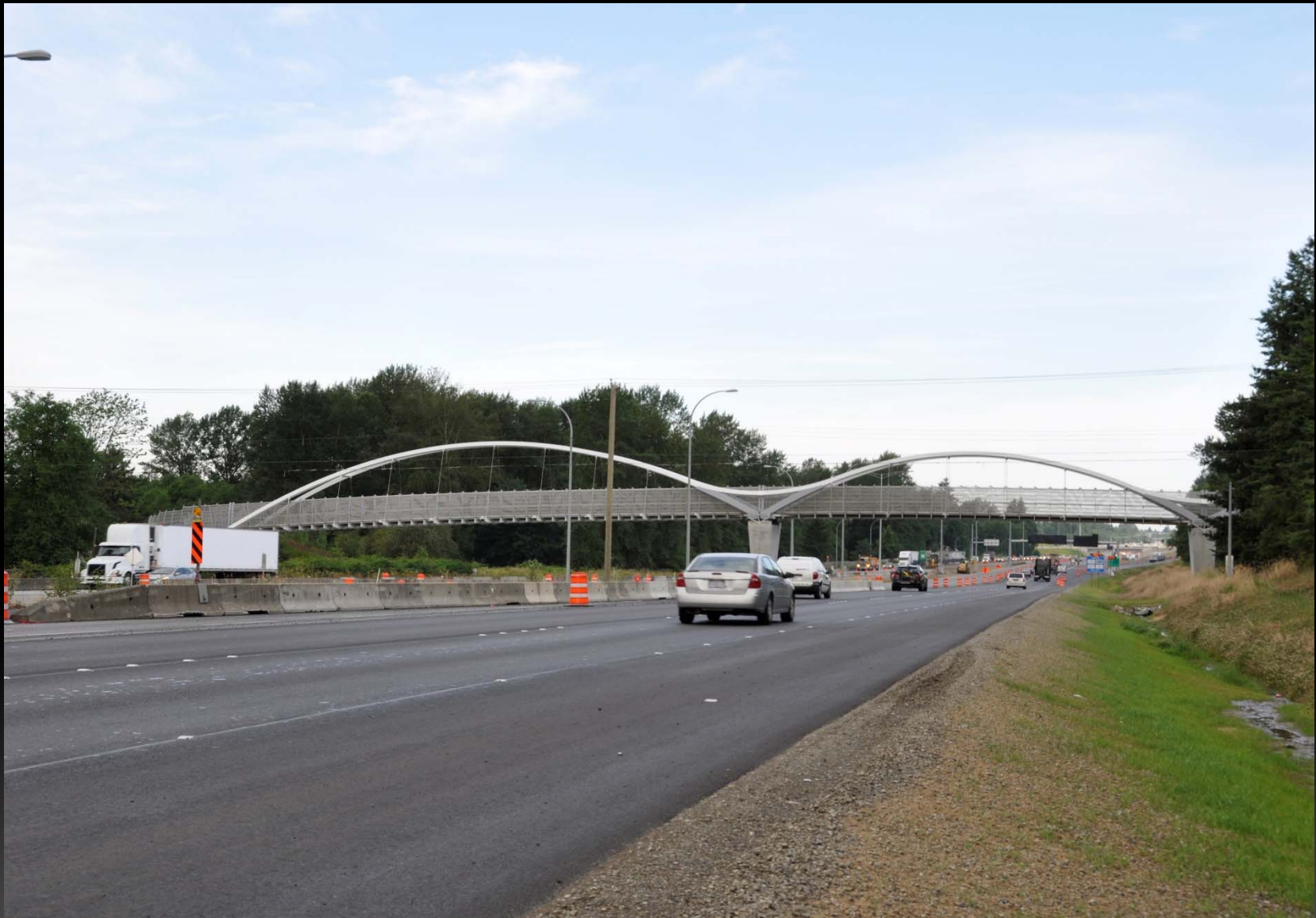
Pedestrian bridge over the Trans Canada Highway outside Vancouver. Two arches, supported at the median, pedestrian deck hung on cables.
