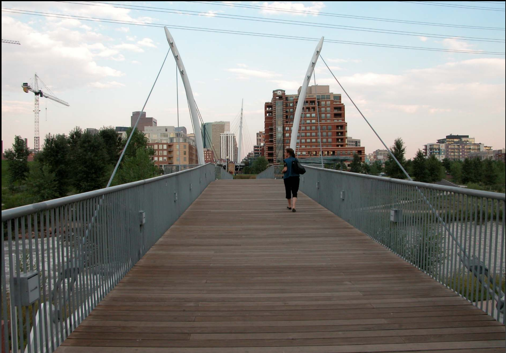
Pedestrian Bridge, Denver, Colorado – a pair of mast supports is used to suspend the bridge deck symmetrically from both sides.
