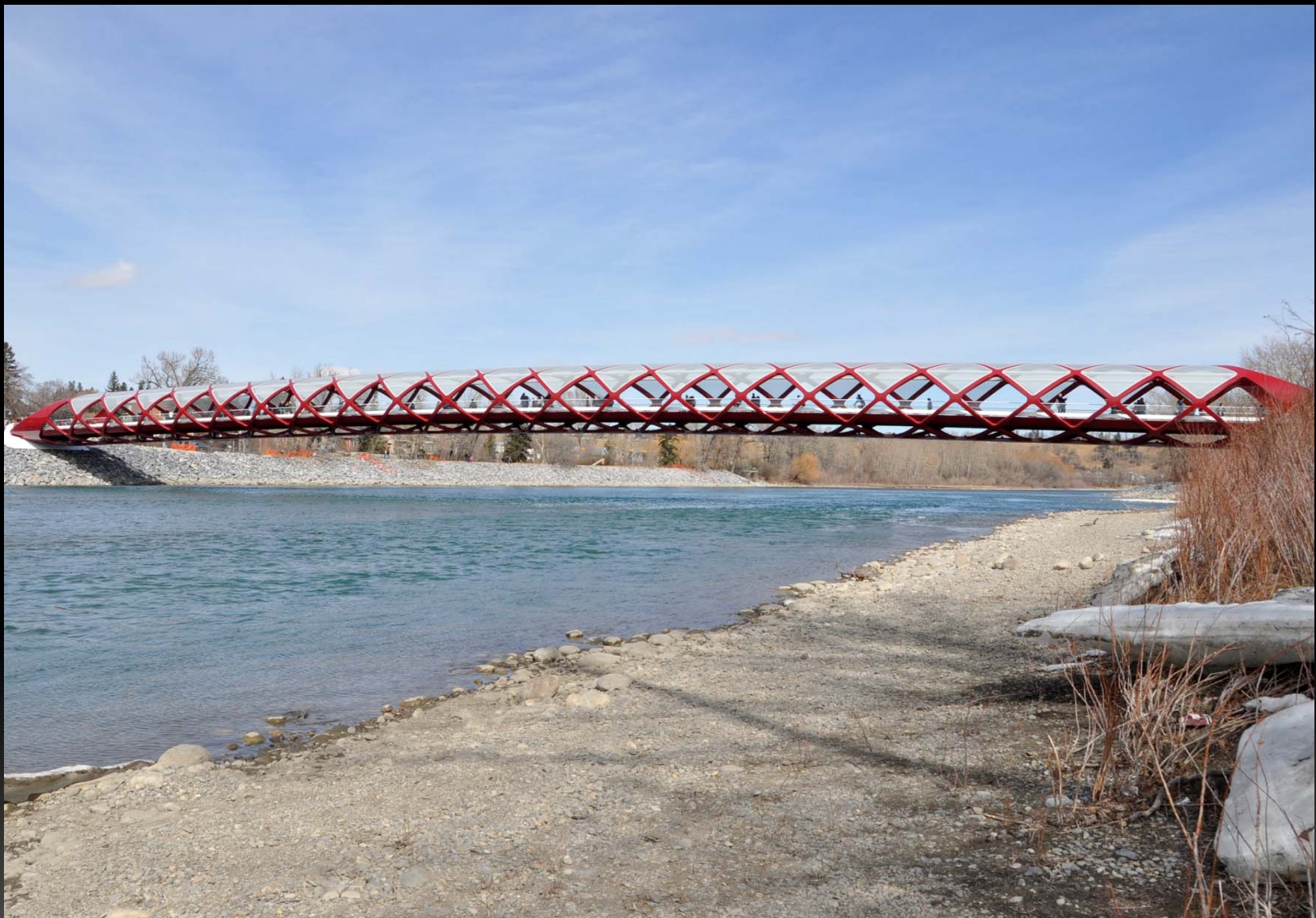
The new Peace Bridge in Calgary, designed by Santiago Calatrava, uses a diagrid type of "Chinese Finger Tube", in a fully welded scenario, to create a very slender span across the Bow River. Span 130 m.
