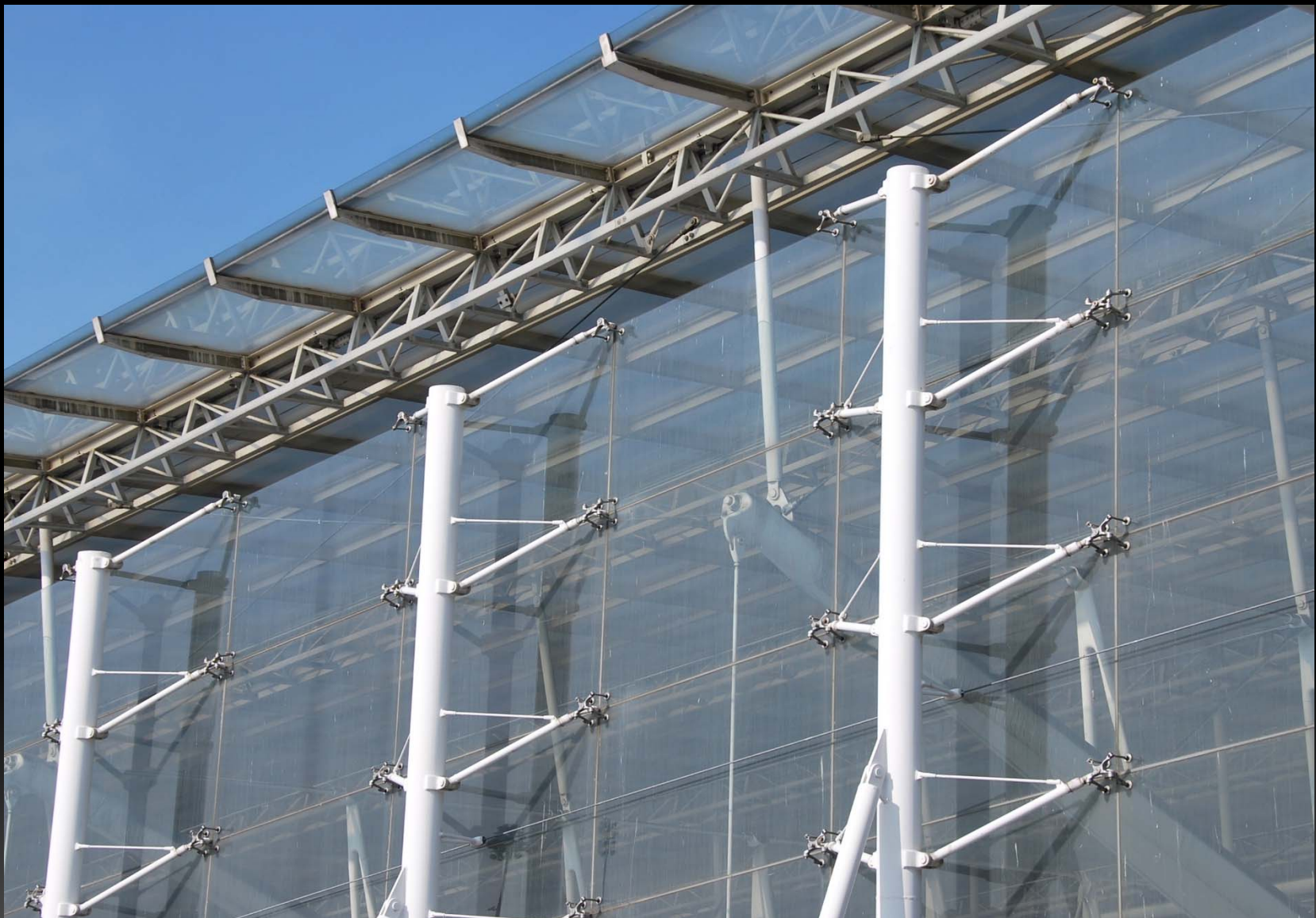
Exterior glazed wall support structure. Also using a smaller box truss along the edge of the upper roof to span between the bowstring trusses.
