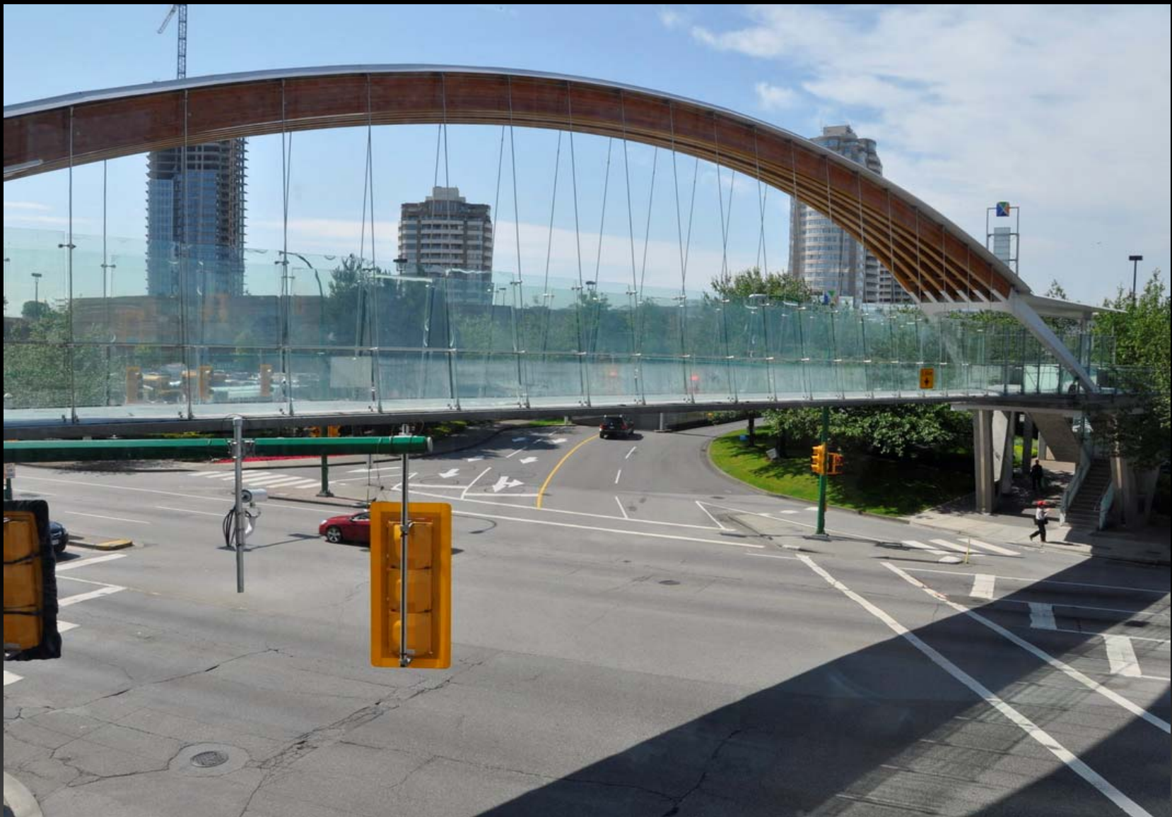
Pedestrian Bridge outside of Vancouver that uses steel and glulam to create an arched structure that supports a platform from cables.
