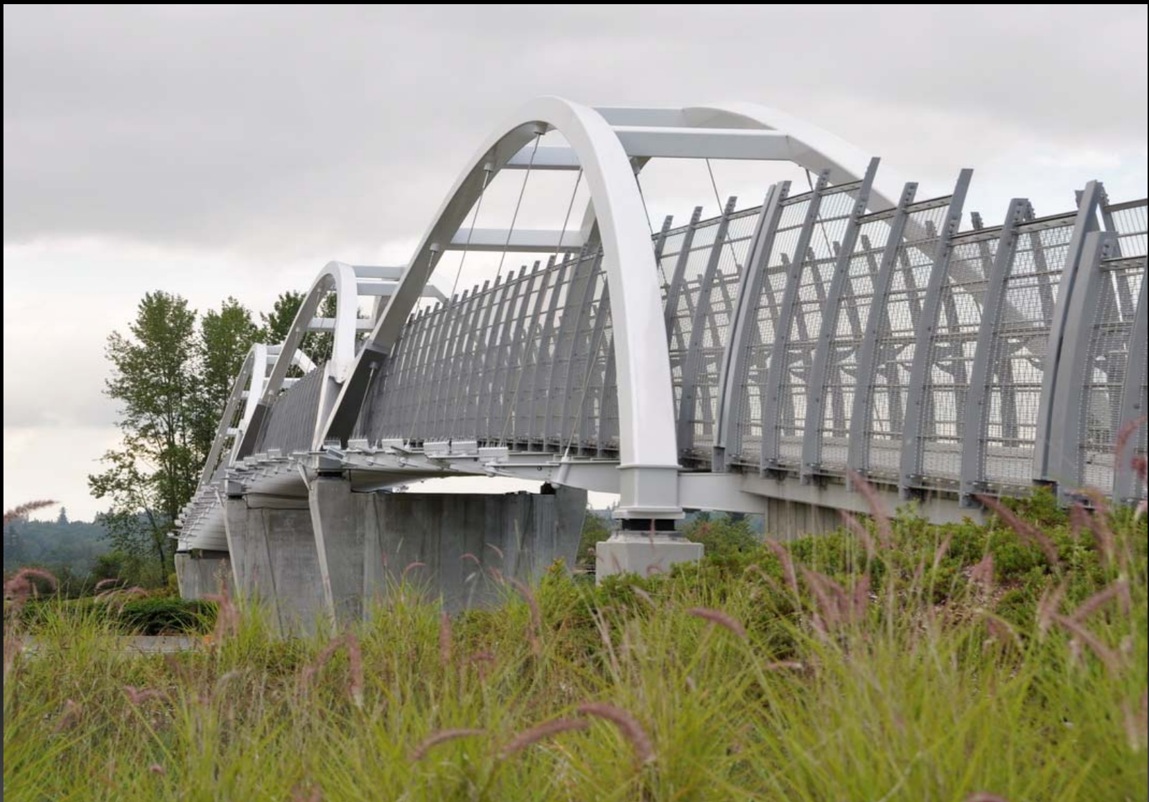
View across the bridge. The arch sections are all custom fabricated from plate steel.
