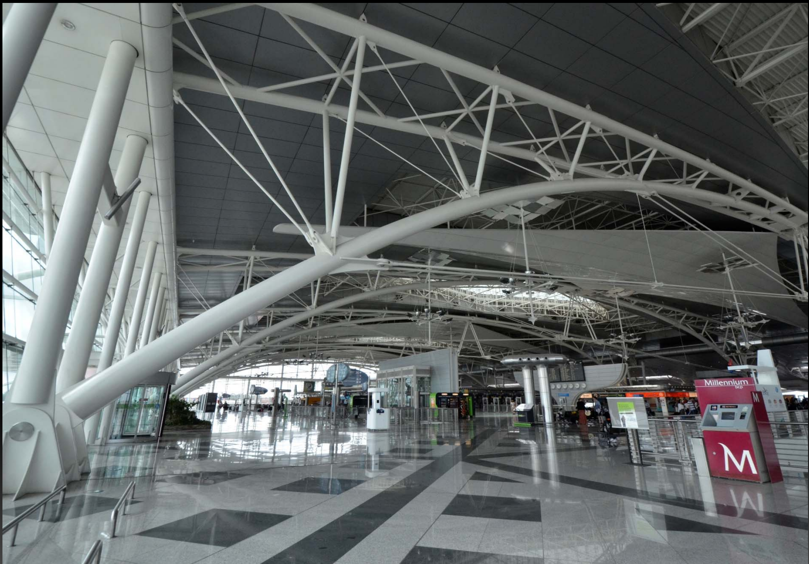
Very large complex triangulated arched trusses clear span across the departures hall.
