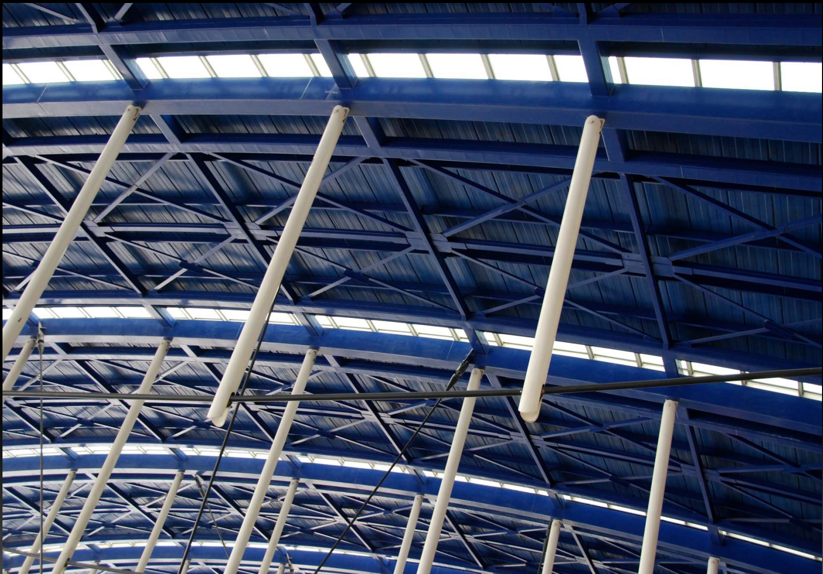
Roof over passenger drop off zone exposes the nature of the structure that is concealed on the interior.
