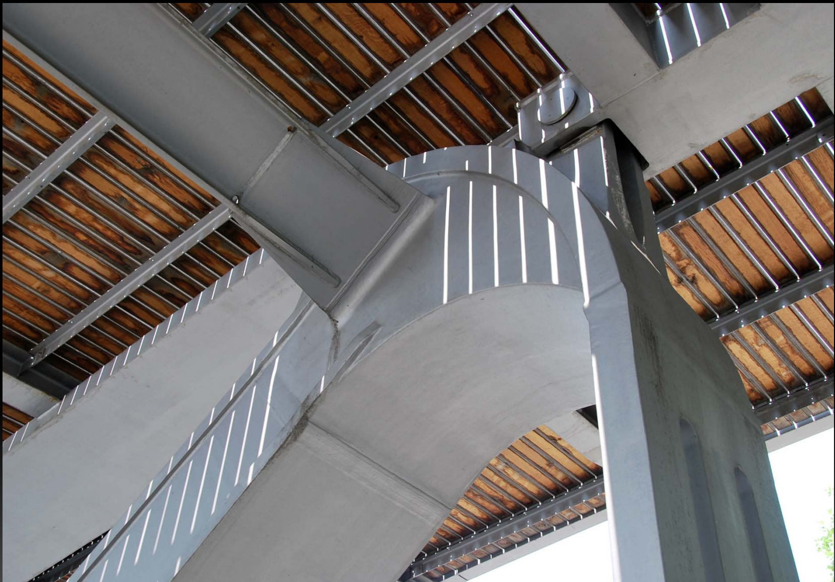
Main connection at the river side to the support system.
