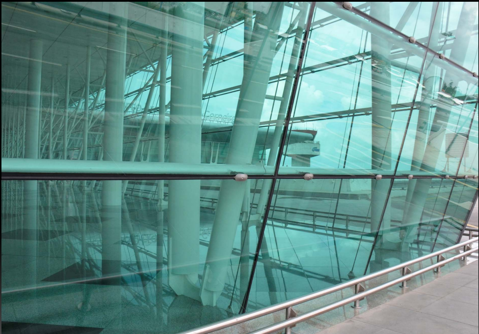
Glass at front wall clips to slender steel members behind.
