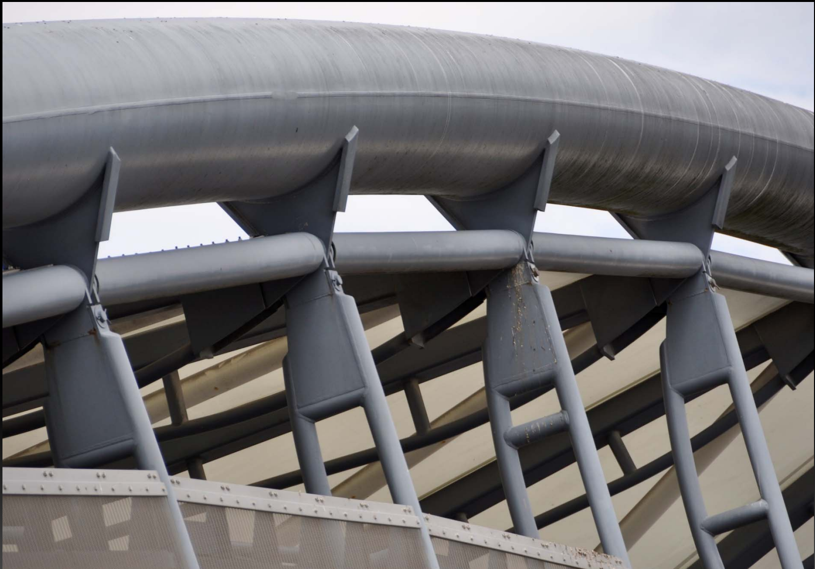
Detail of the connection of the "wall" support system to the upper tube.
