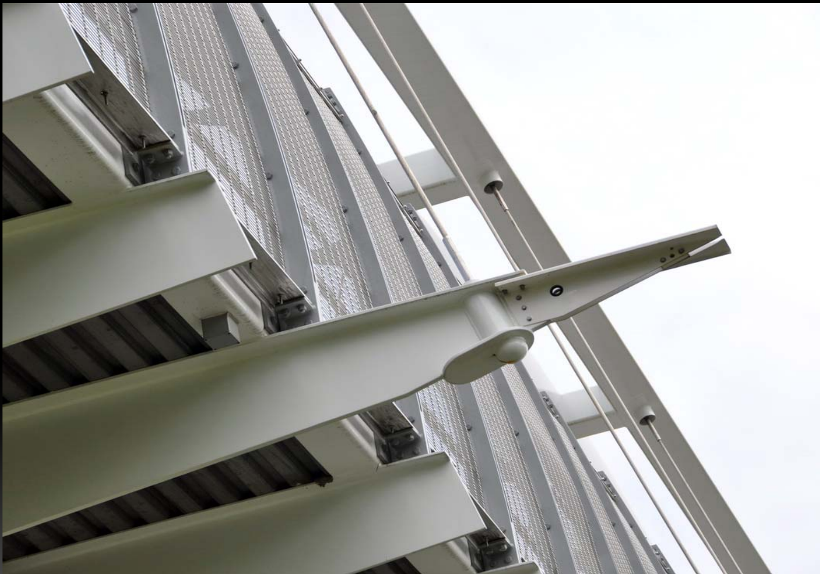
Edge detail from below. See the galvanized decking that spans between the white T beams.
