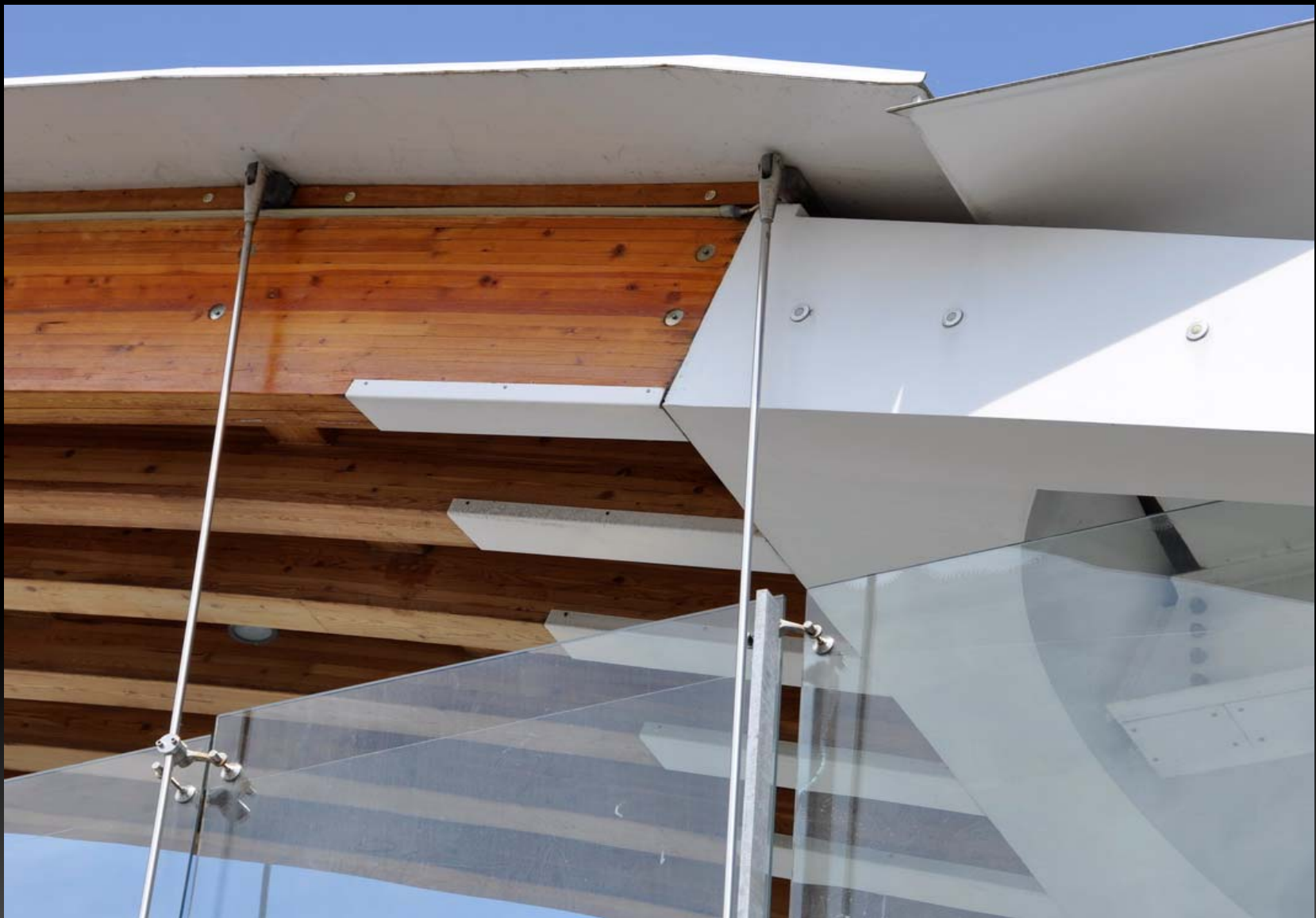
Detail where wood and steel meet.
