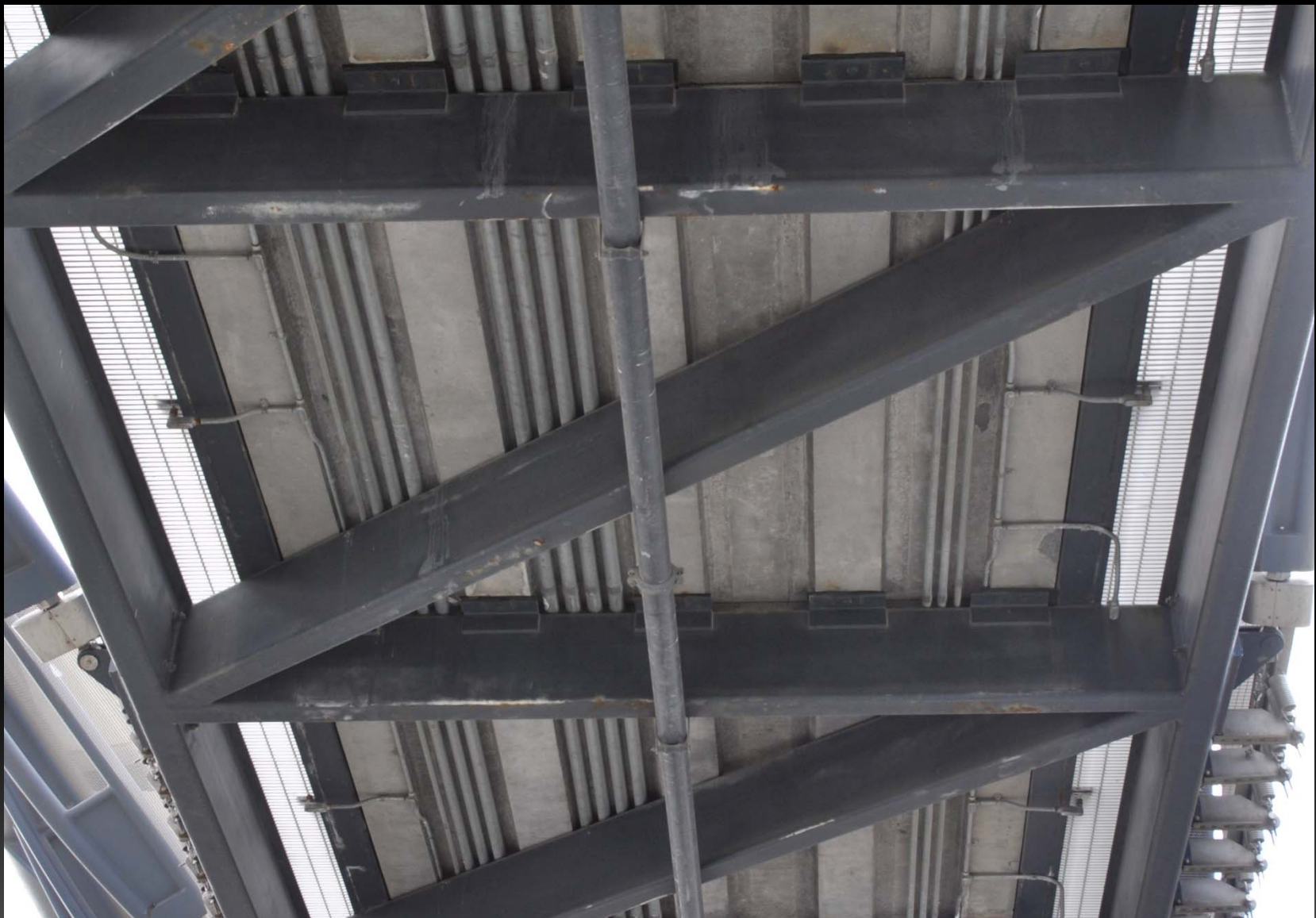
View of underside of bridge showing fairly standard truss arrangement to support walkway.
