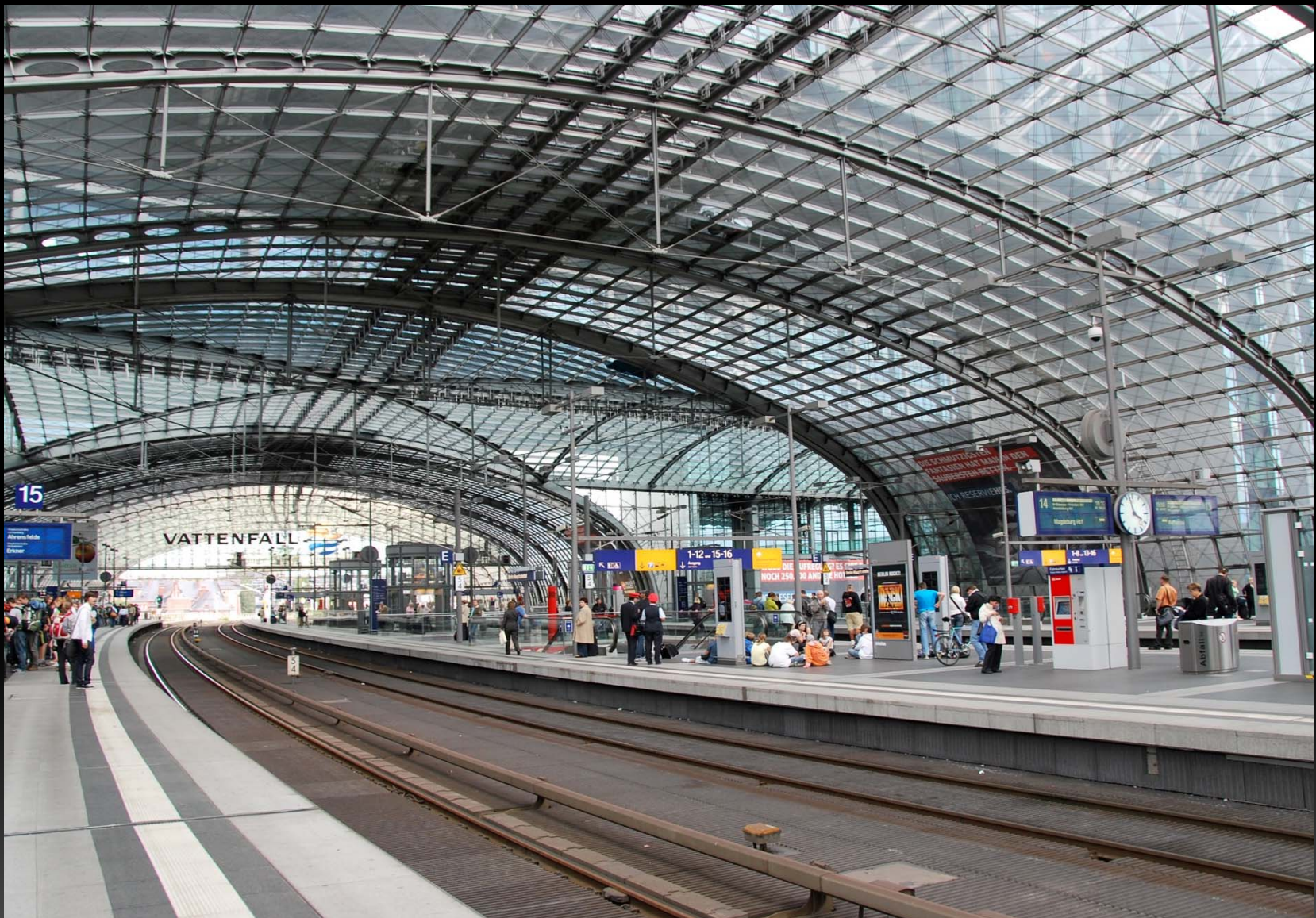
Curved, castellated beams with tension support.
