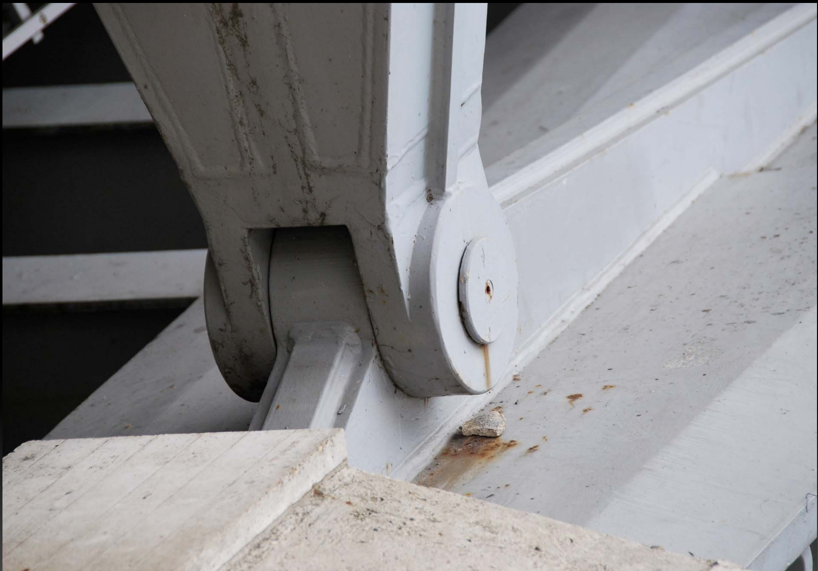
Custom hinge connection at one of the abutments to connect the upper level to the lower level.
