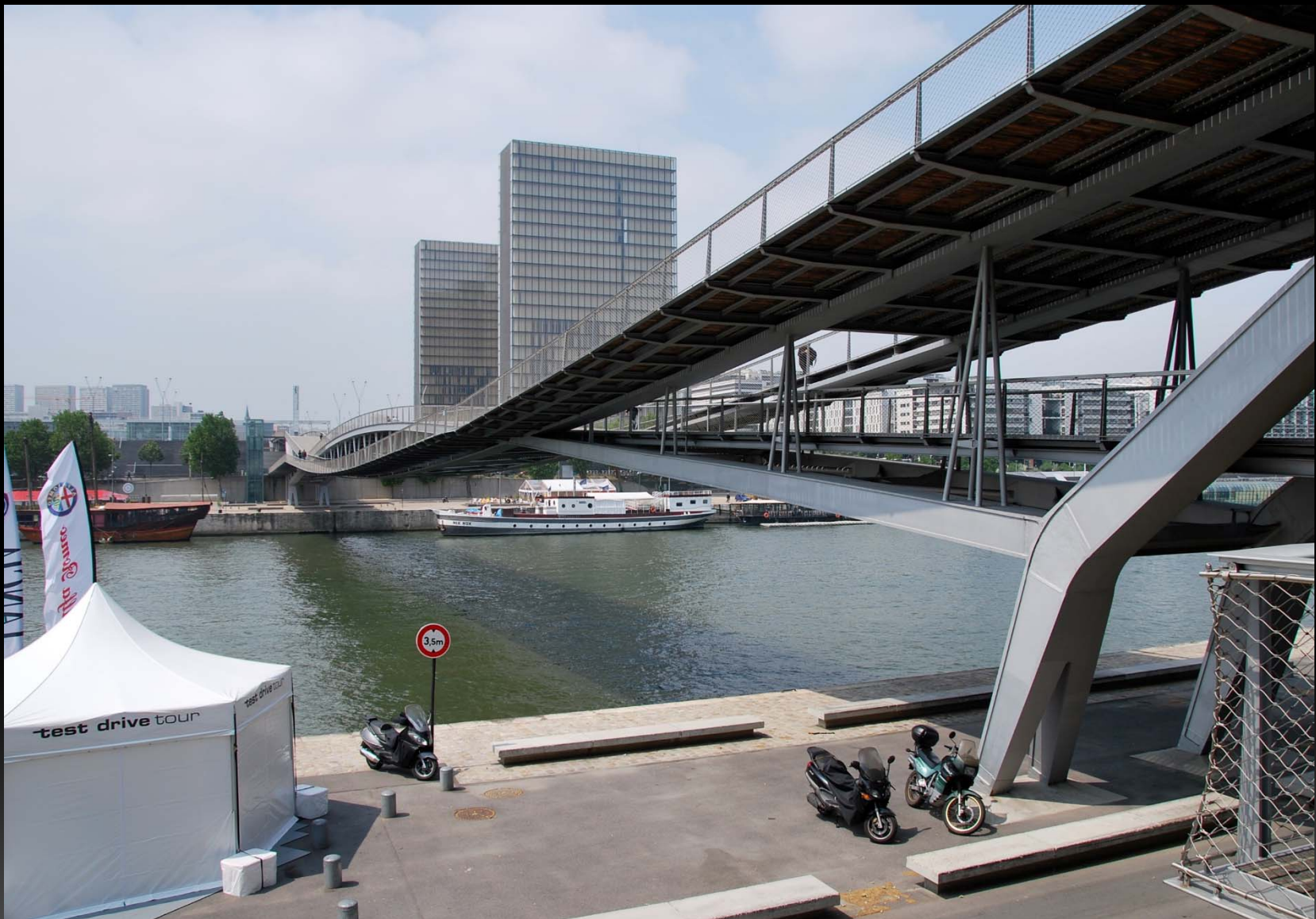
Simone Beauvoir Footbridge by RFR, Paris, France
