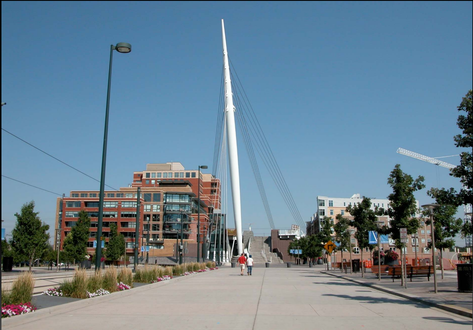
Millennium Bridge Denver, Colorado – single large mast to suspend walkway.
