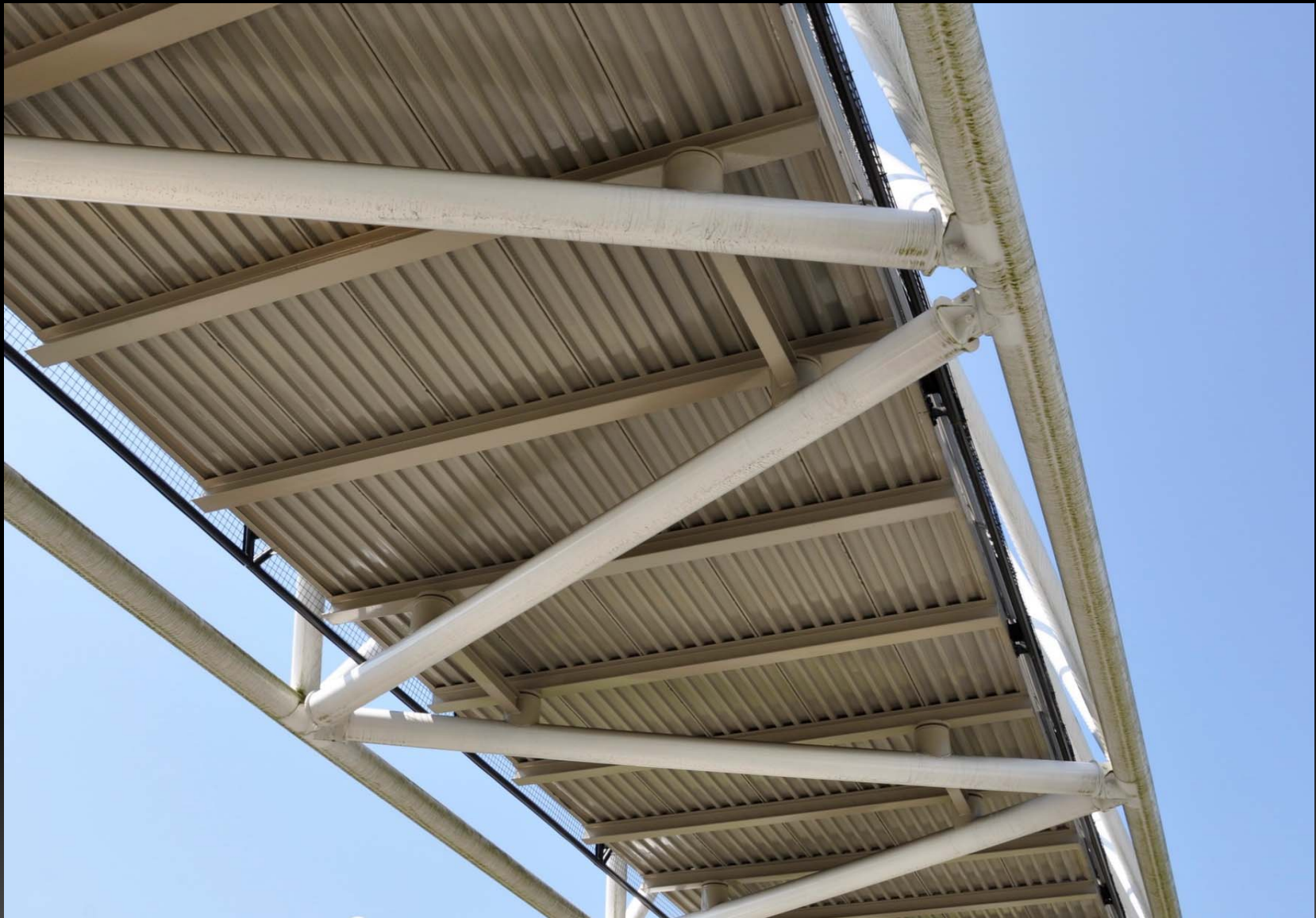
View of secondary spanning systems. Note bolted connections at connection to top part of bridge truss.
