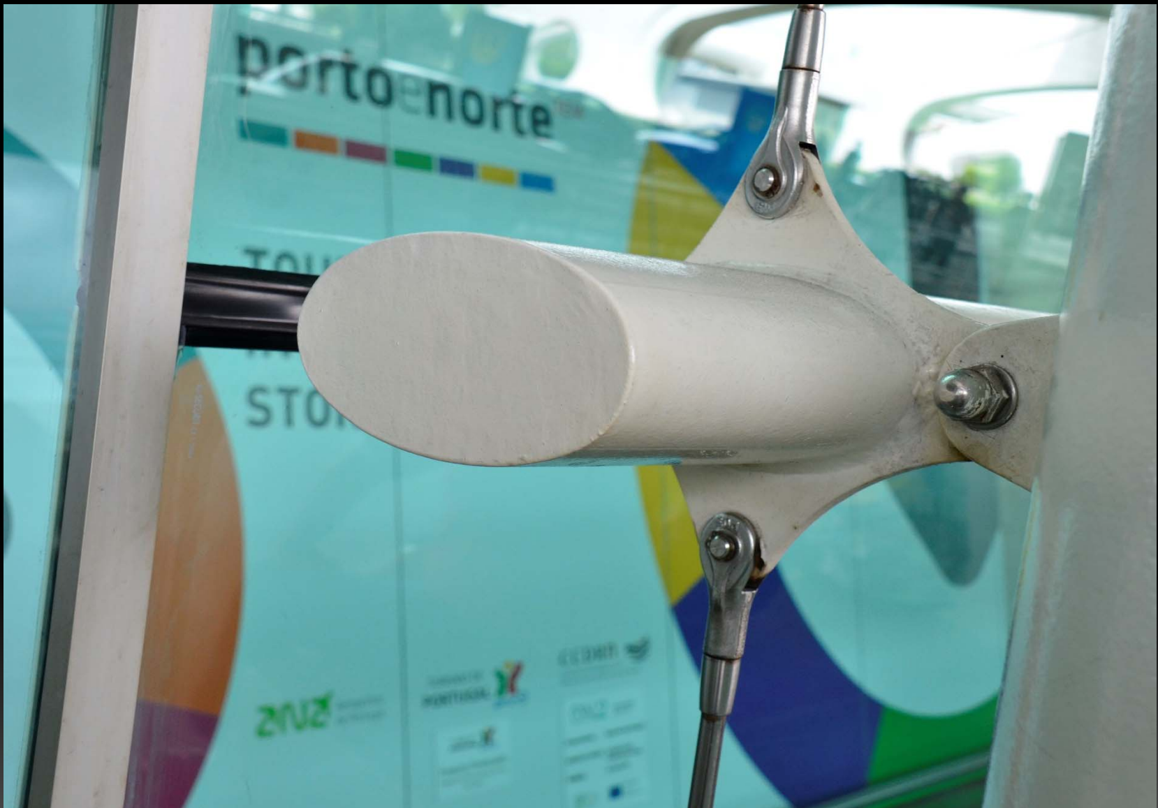
Glazing supported by elliptical tubes that are bolted to the trusses via small plates. Hung from above with stainless rods.
