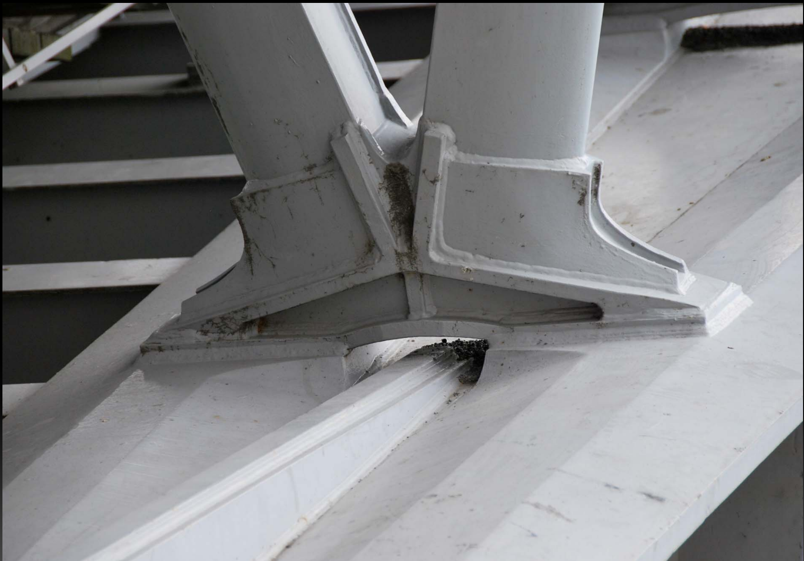
Special "feet" to connect the elliptical tubes to the base of the support system.
