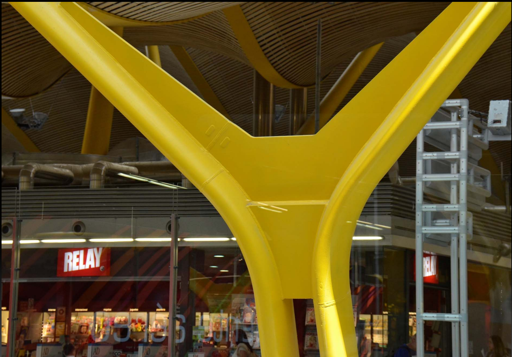
Alternate support system on the interior. Use of elliptical tubes. Exposed welds.
