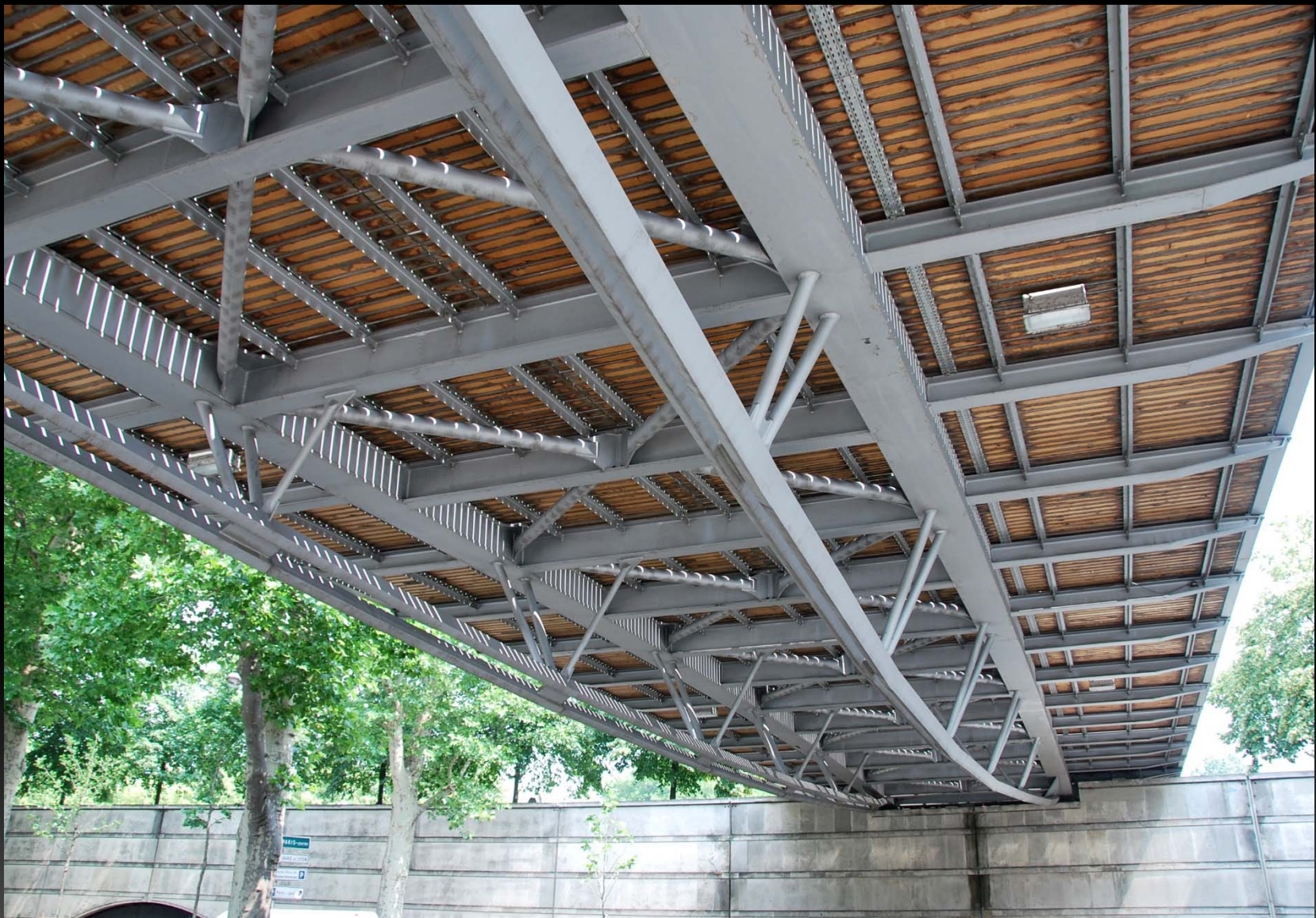
Support system where bridge crosses over road at side of span. Note the multiple layering of span conditions.
