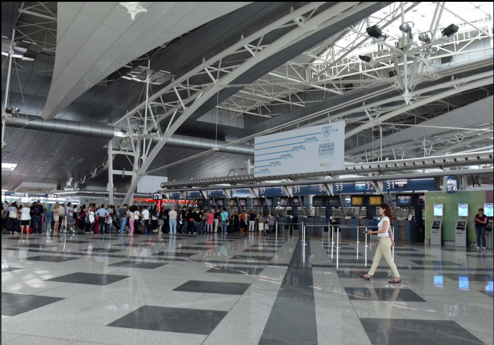
Very light tension below visible truss.
