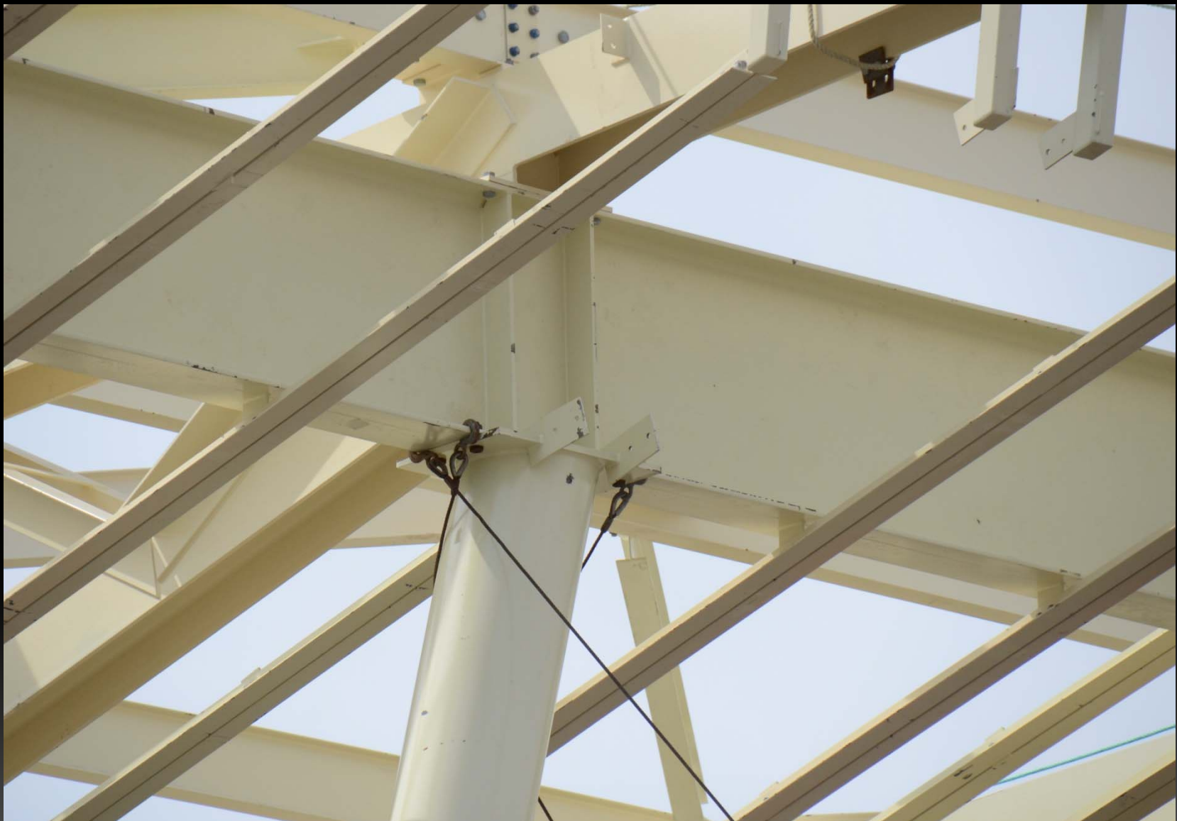
Column to beam connection
