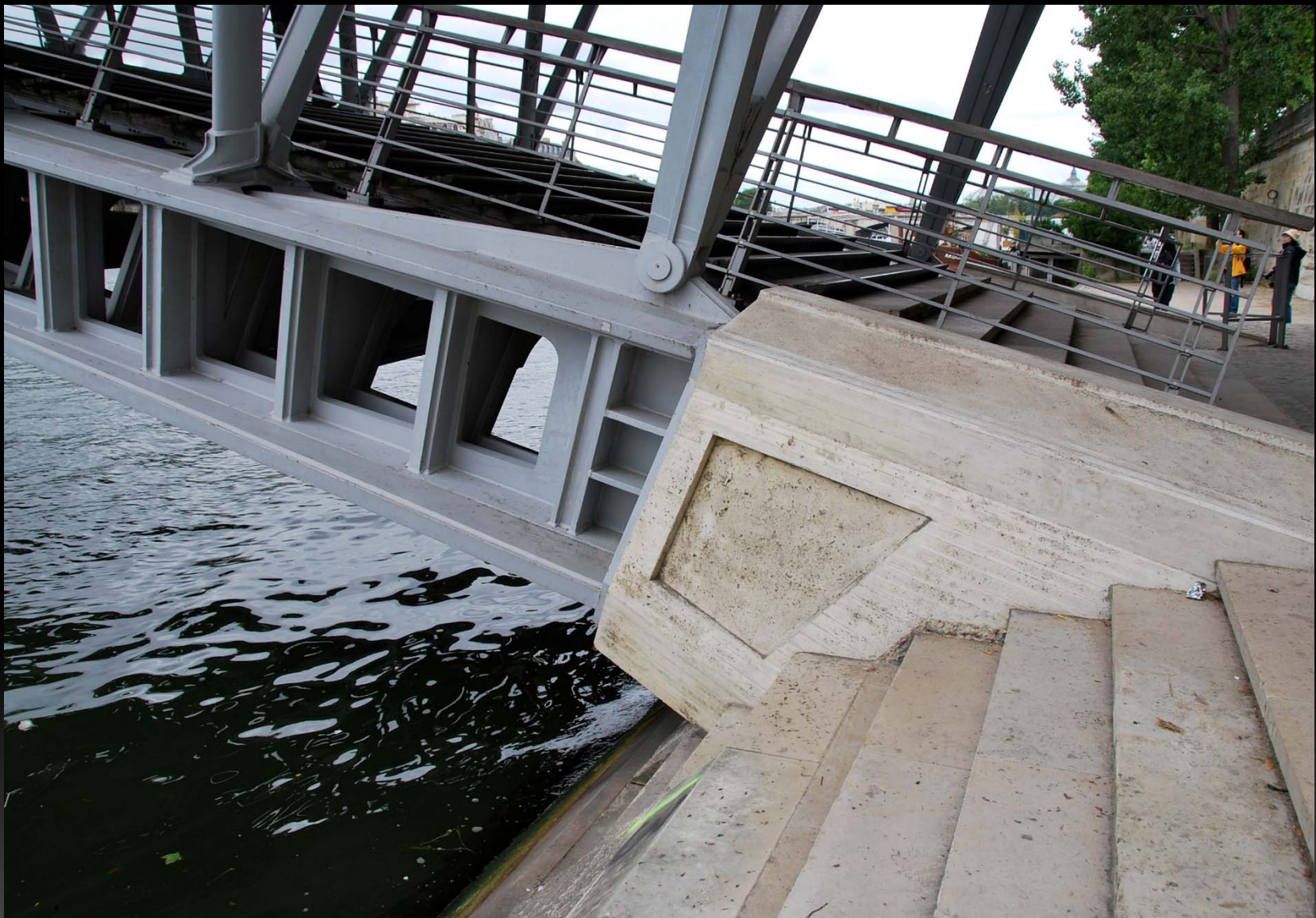
Concrete abutments absorb the thrust of the lower section.
