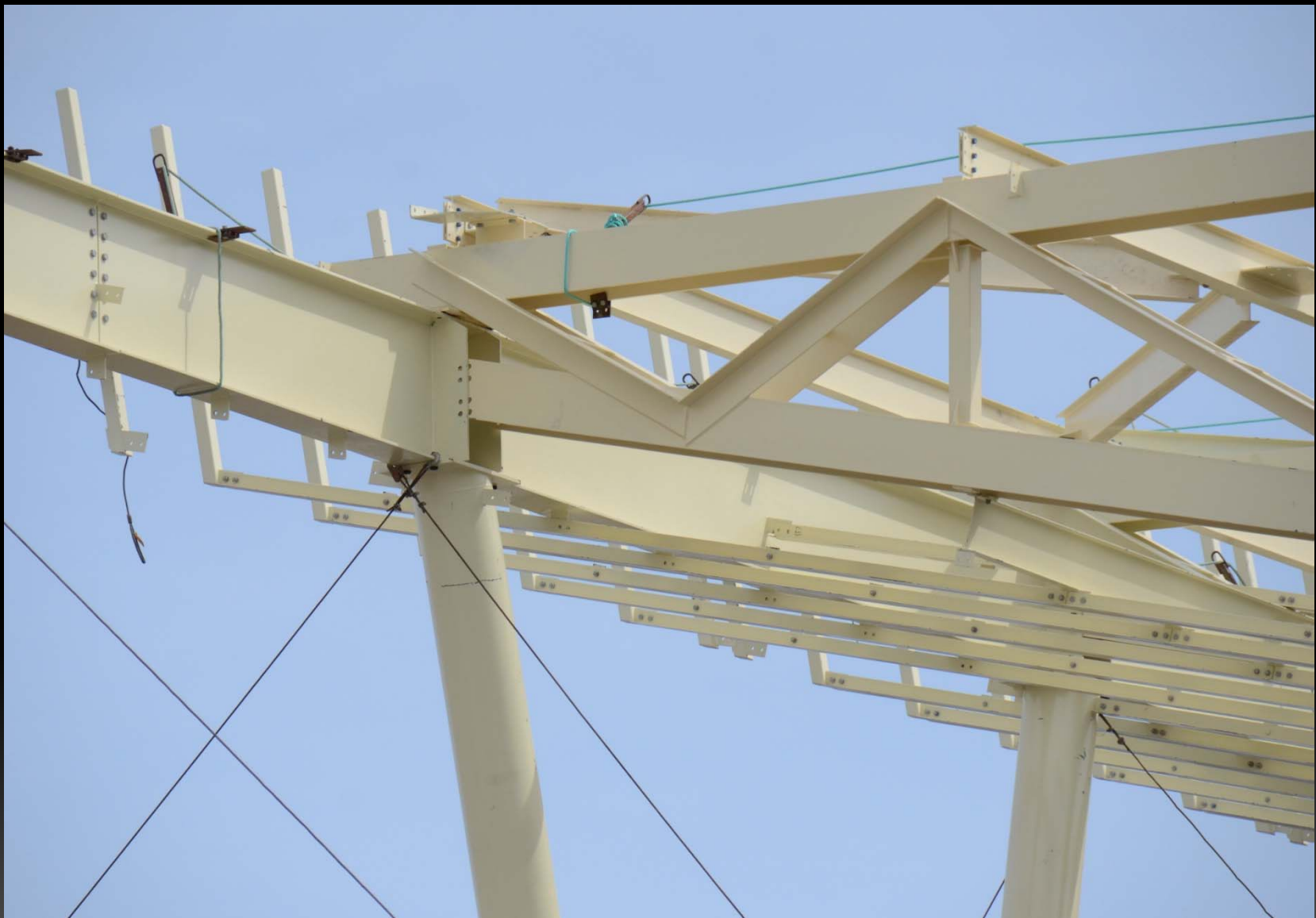
Bolted vs welded connections
