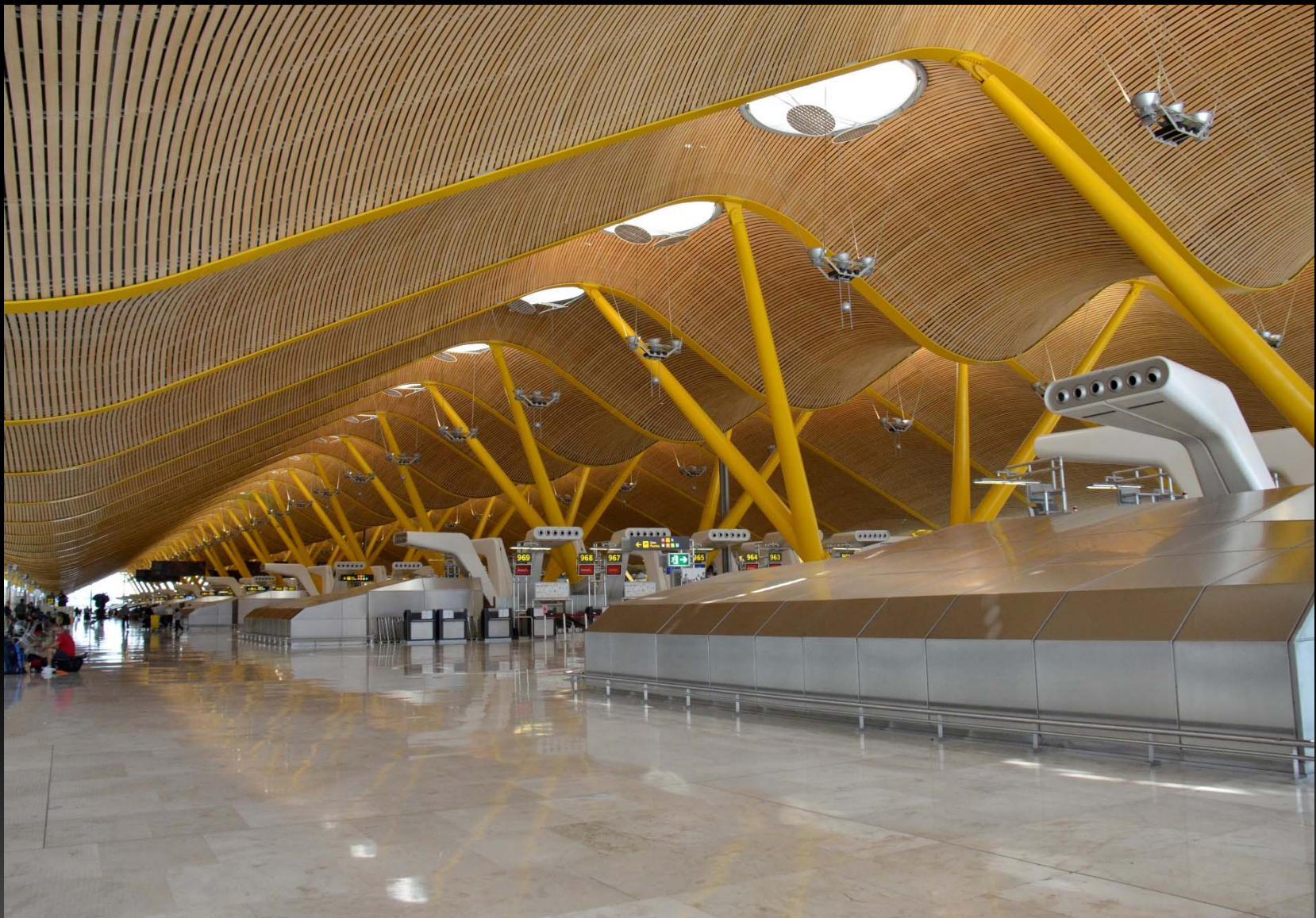
Madrid Barajas Airport, Terminal 4 by Richard Rogers. The use of the long tapered tubular supports helps to decrease the span of the curved members.
