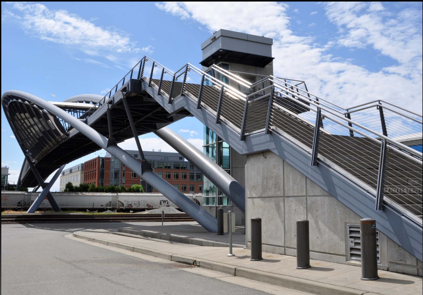
Large round HSS tubes create a criss-crossed support system for the walking platform and the partial canopy covering.
