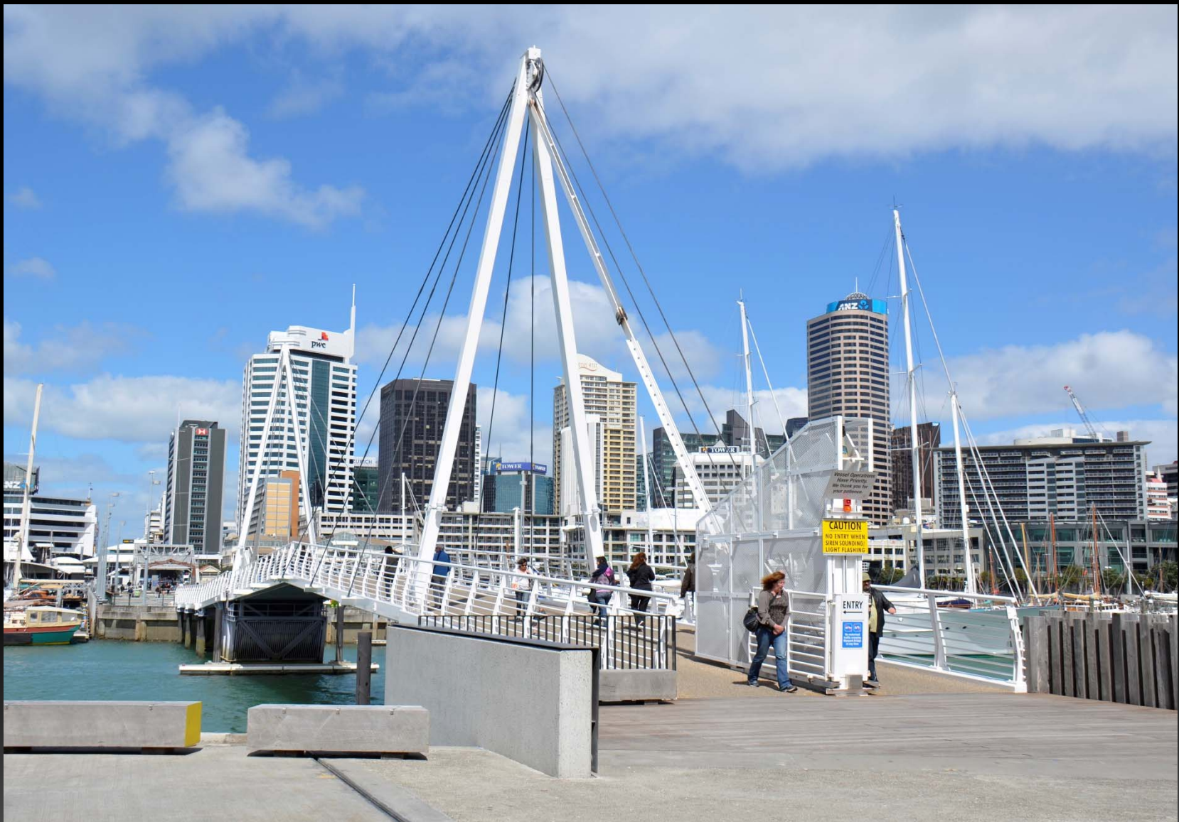
A lift bridge in Auckland, New Zealand.
