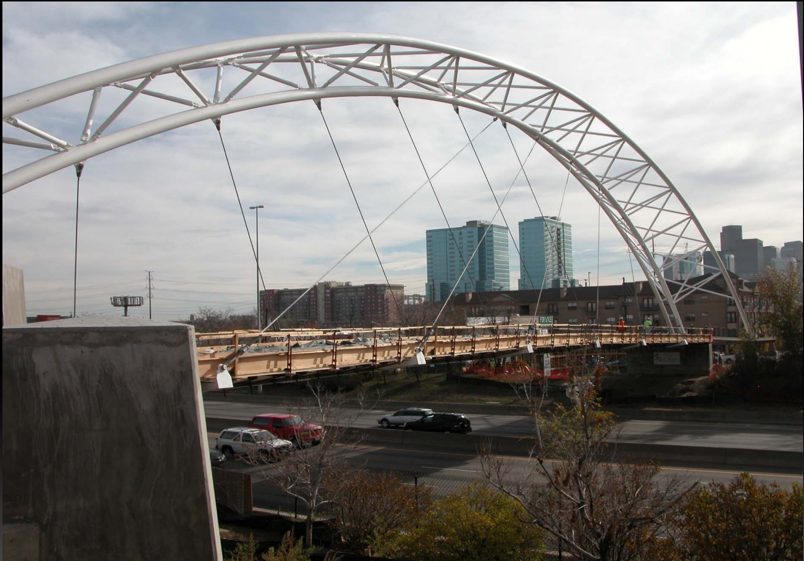
Triangulated truss with suspension system for the bridge platform. Note the asymmetry of the cables.
