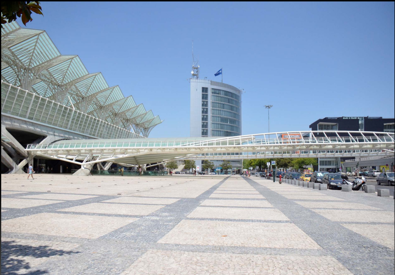
Side view of bridge as it spans across the plaza and multi lane street.
