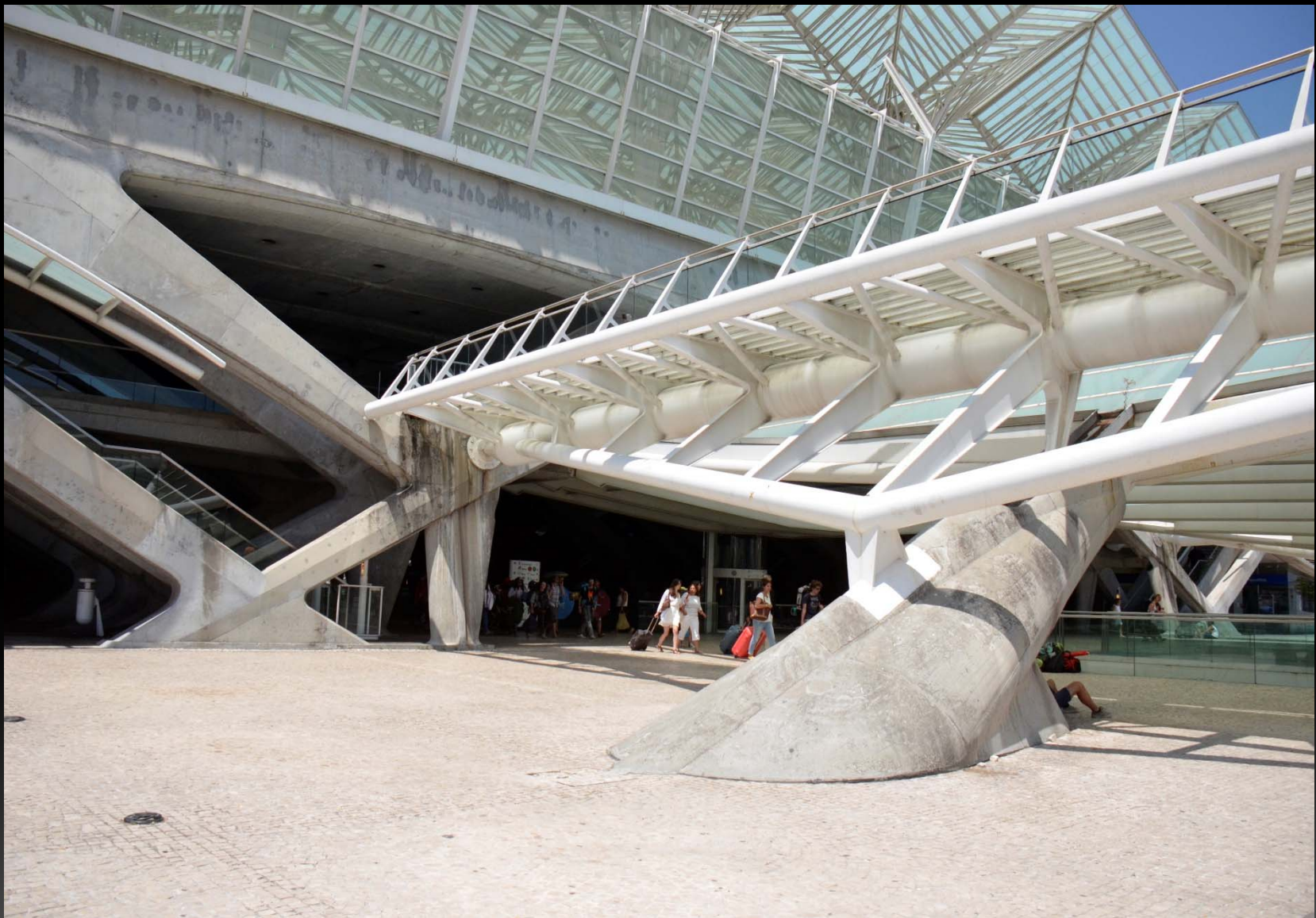
Concrete support for the bridge. Bridge structure uses round tubes and tapered wide flange type members.
