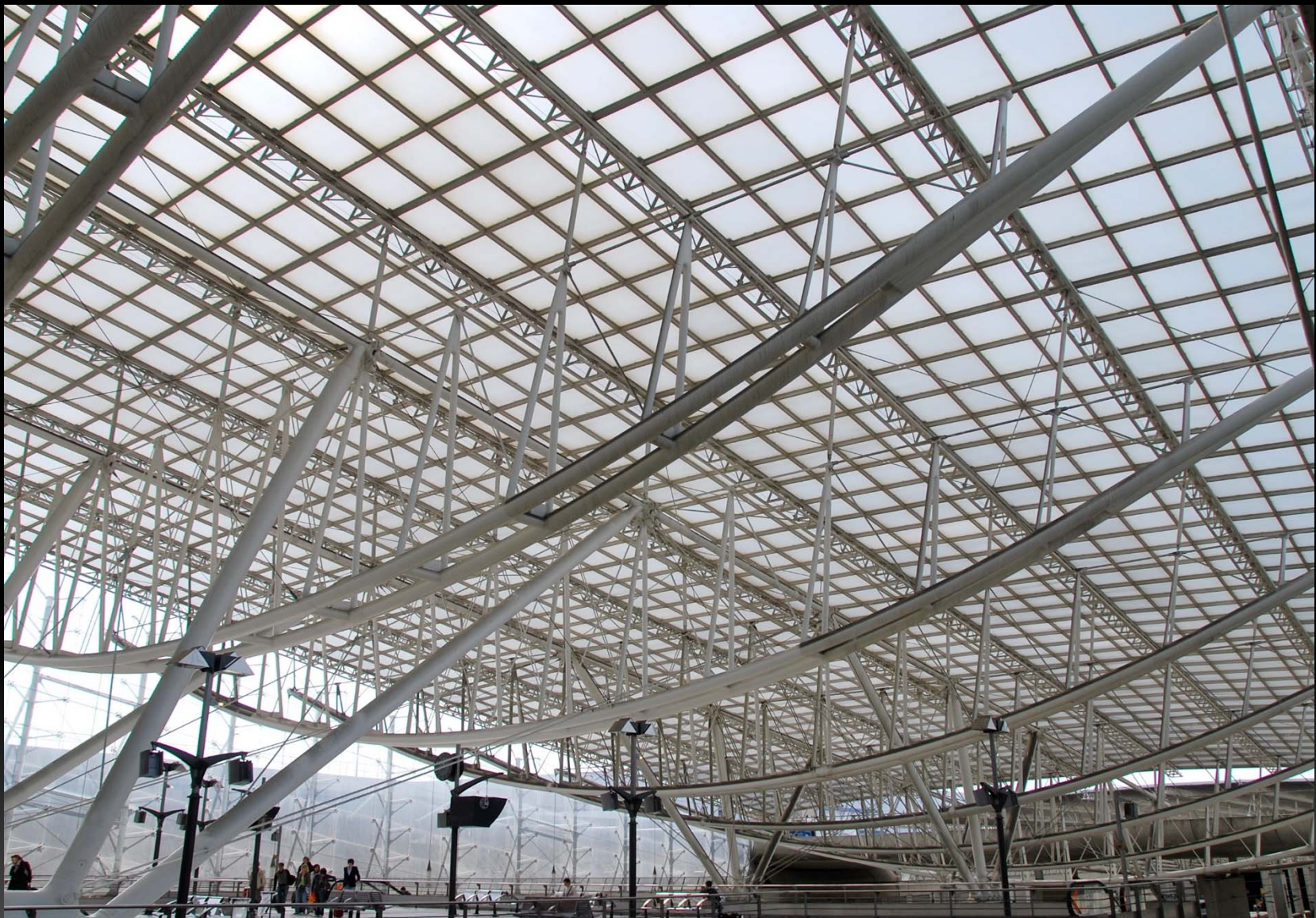
Peter Rice, TGV Station at Charles deGaulle Airport in Paris. Inverted bowstring truss.
