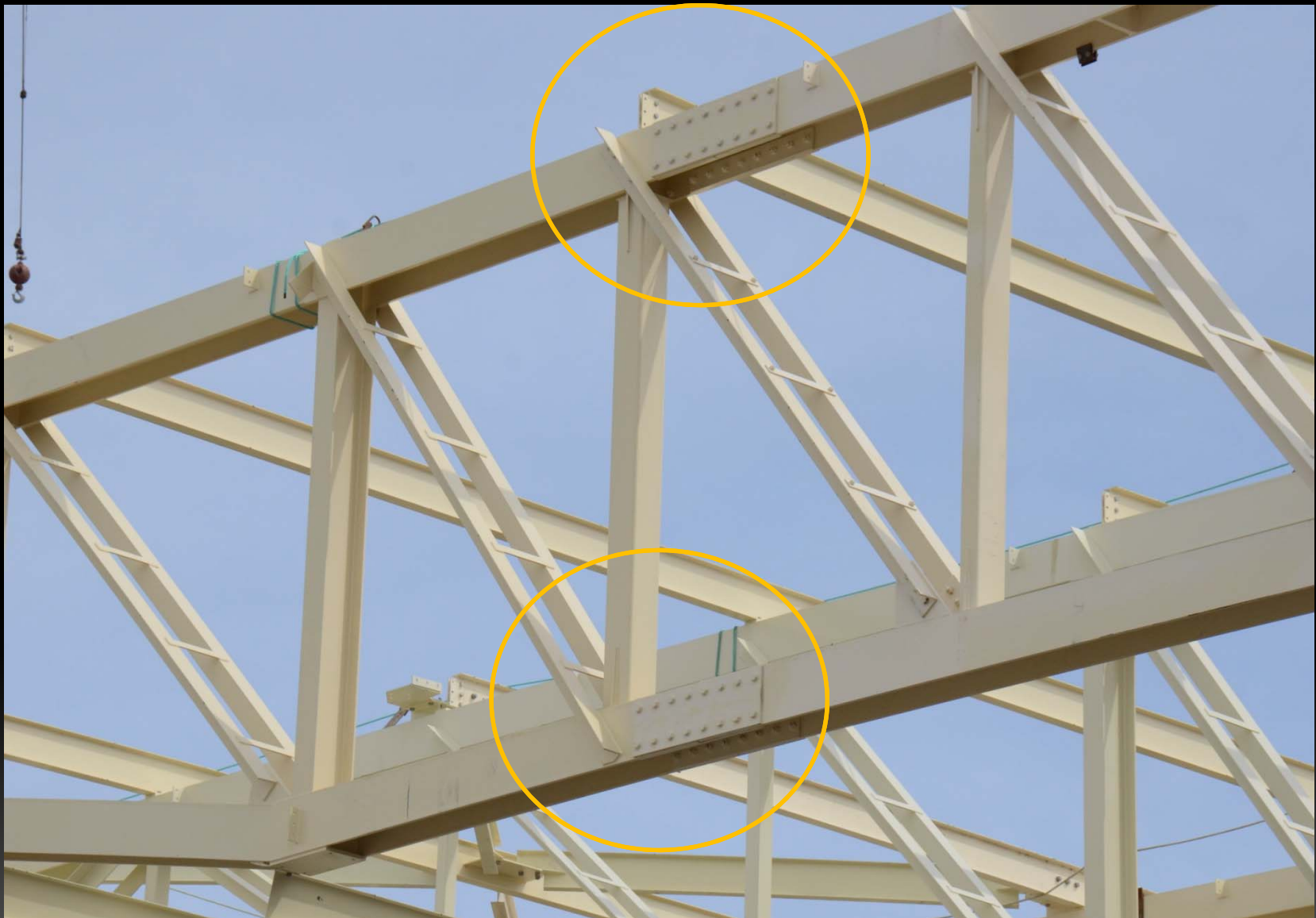
Splicing the trusses
