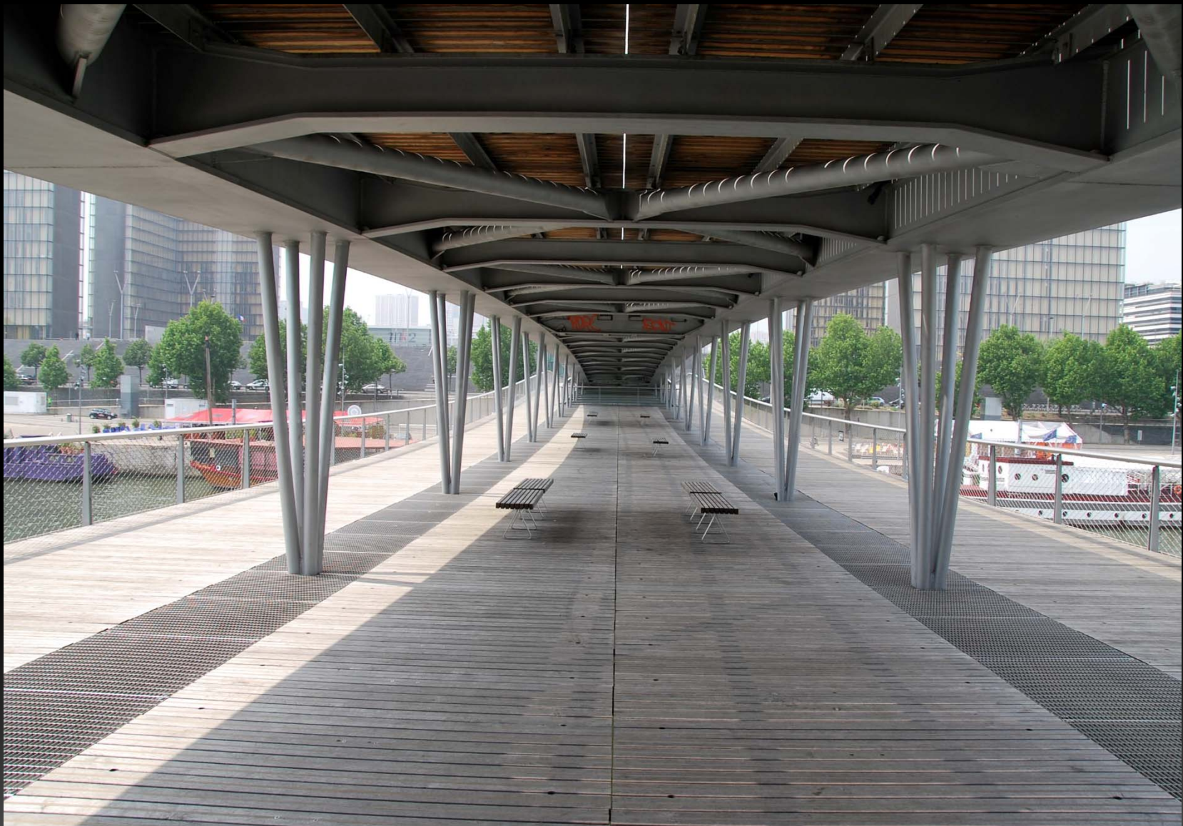
A resting space inside the bridge showing the construction of the top platform.
