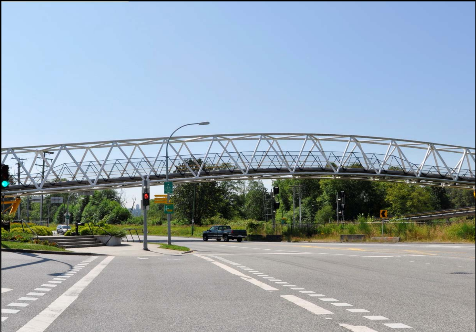
Pedestrian bridge outside of Vancouver. Box truss gently arched as it passes over the street.
