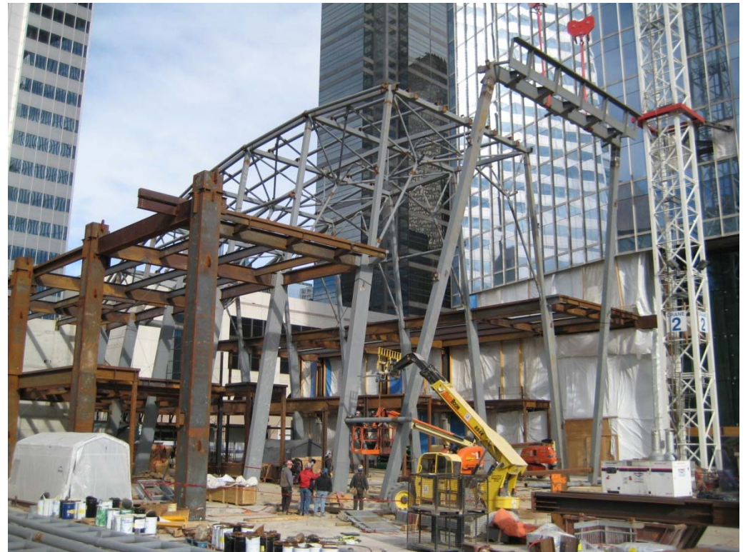
Last Arch erection
