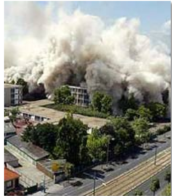
Pruitt Igoe Housing development.
