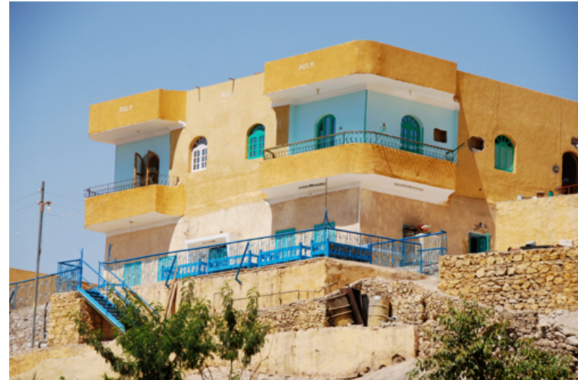
Traditional House in Egypt
