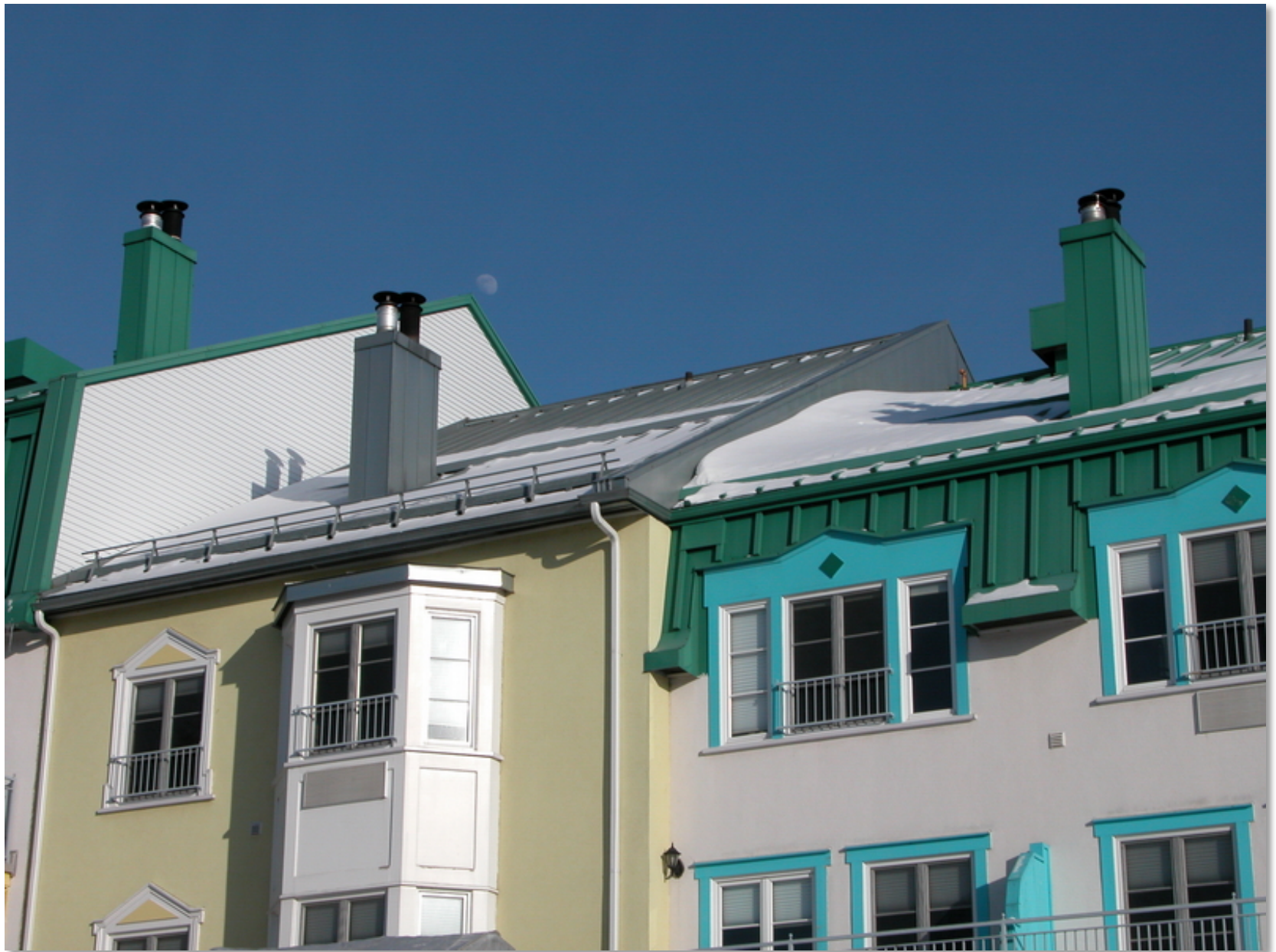
Snow guards at the edge of roofs
