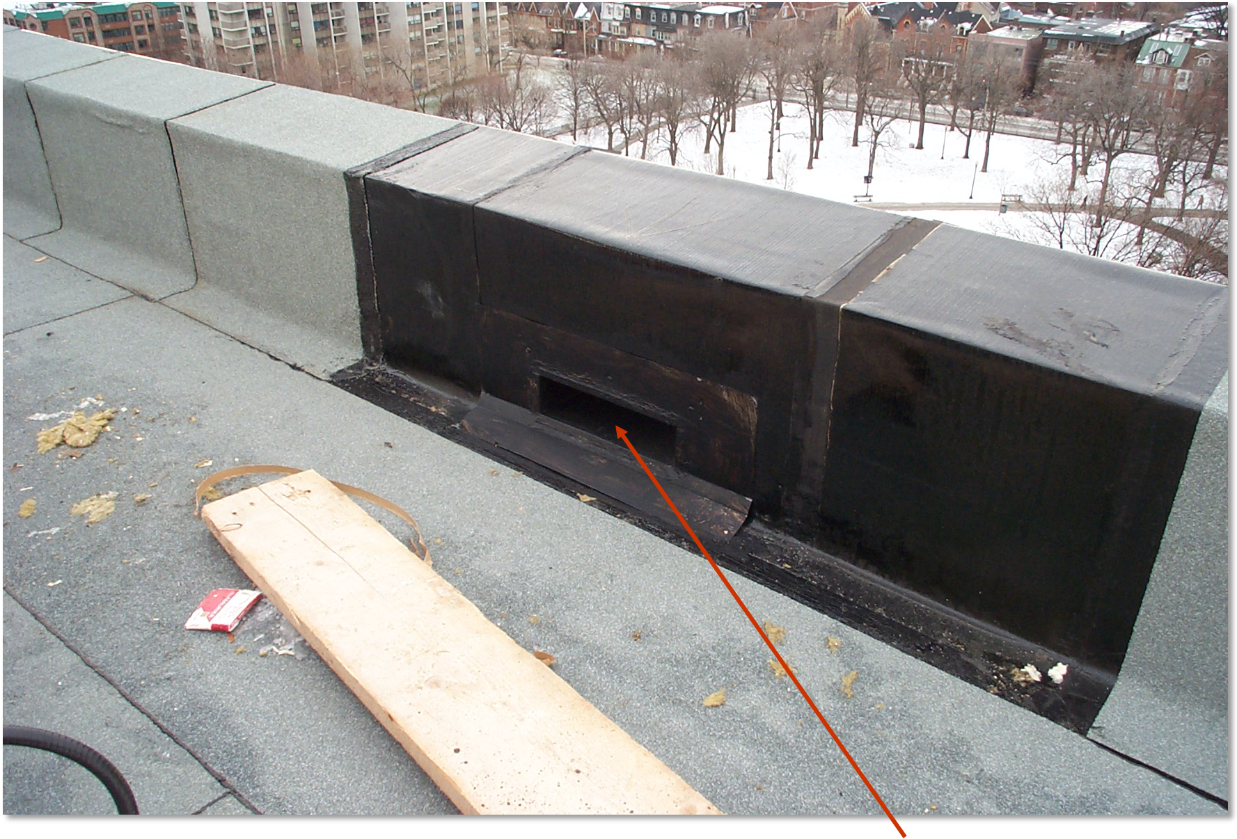
Detail at parapet. Note water overflow opening.
