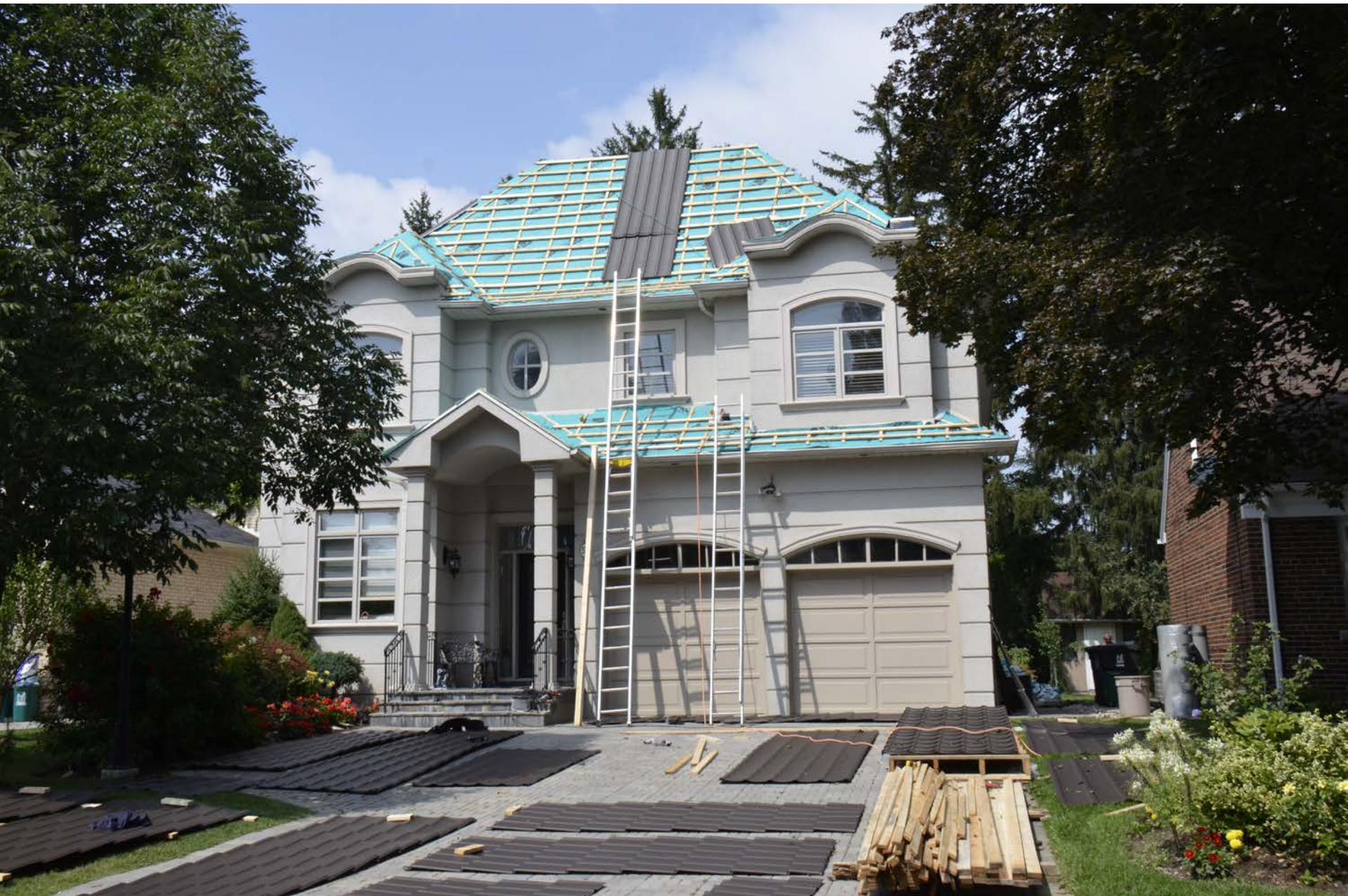
Contemporary tile look roof with underlayment
