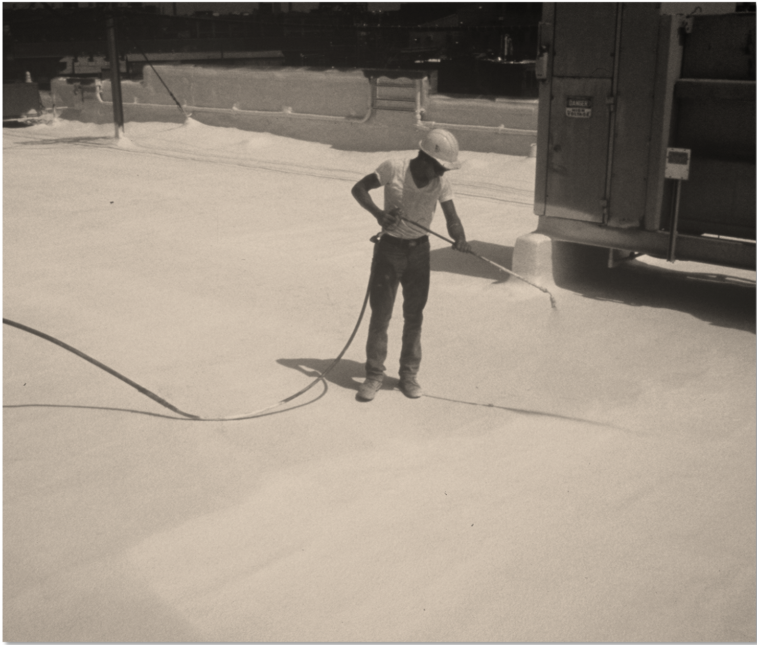
Spray applied elastomeric membrane roofing
