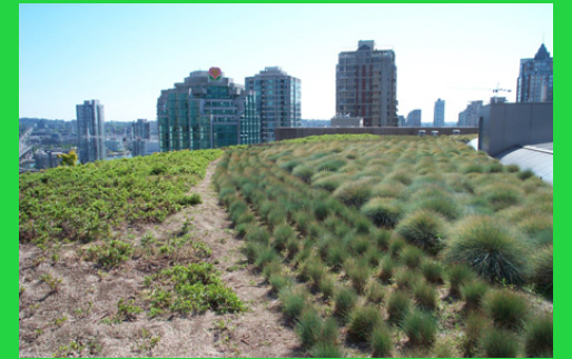
Green roof at Vancouver Public Library
