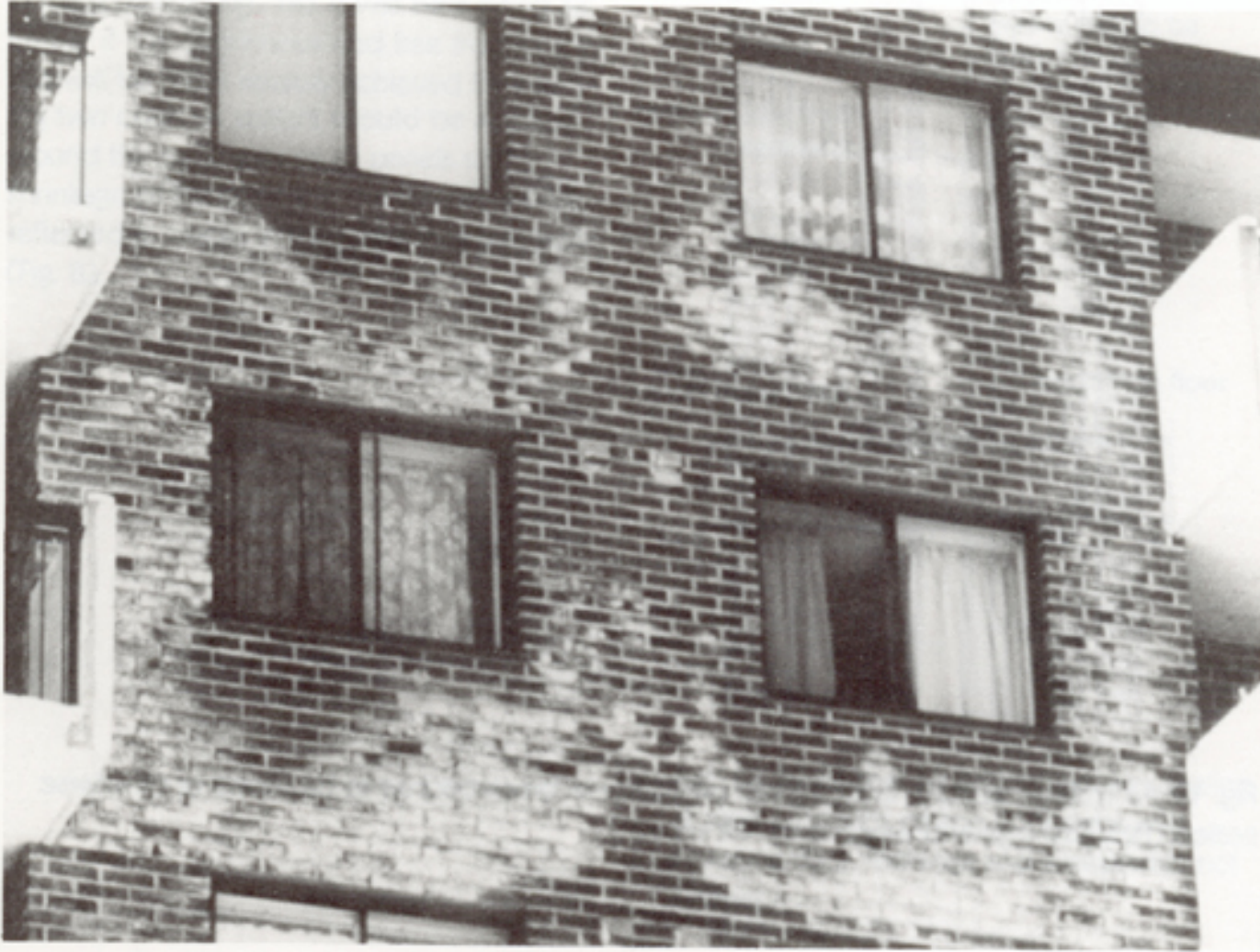
Fig. 16 An example of extensive wetness and efflorescence
