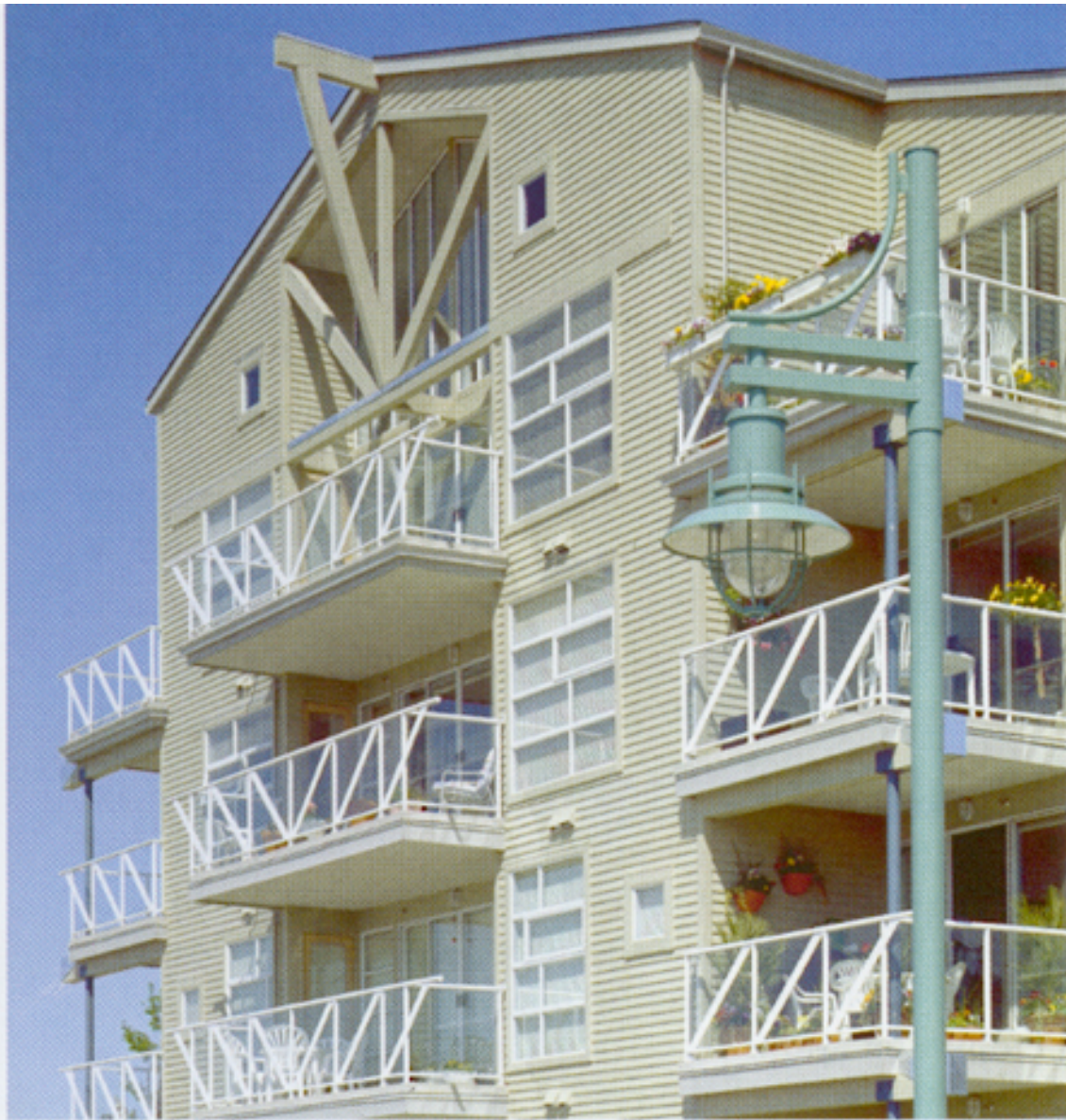
Figure 2 Four Storey Wood Frame Residential Construction
