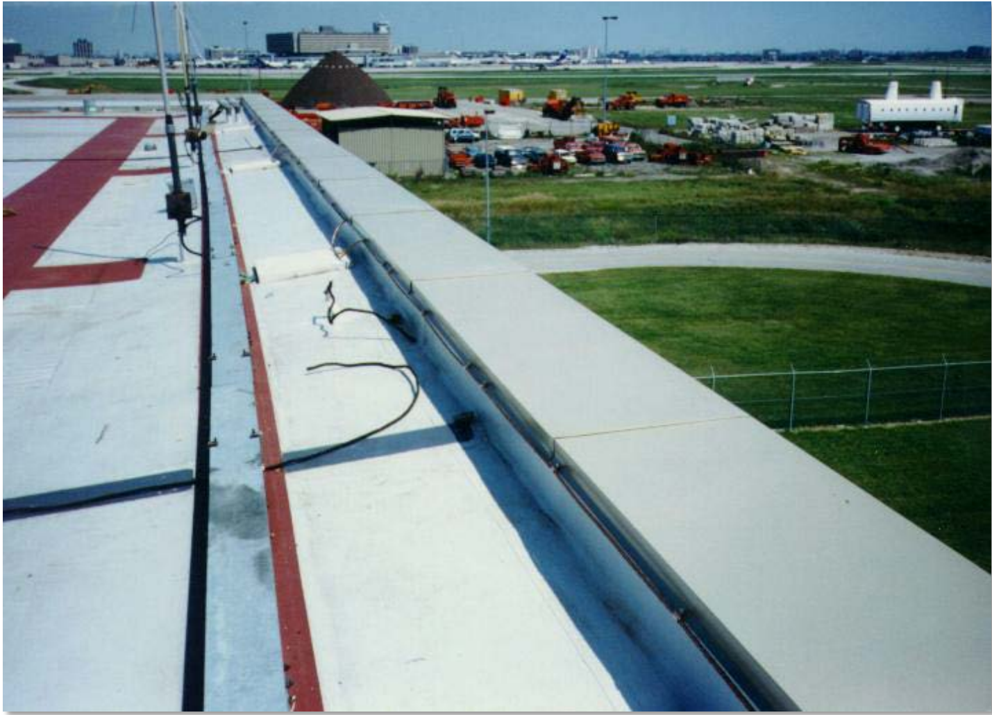
PVC Roof at Pearson International Airport
