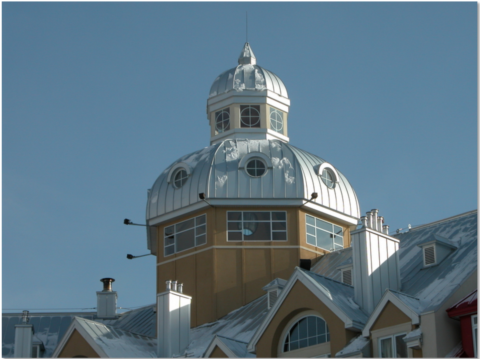
Contemporary terne-look roof in standing seam
