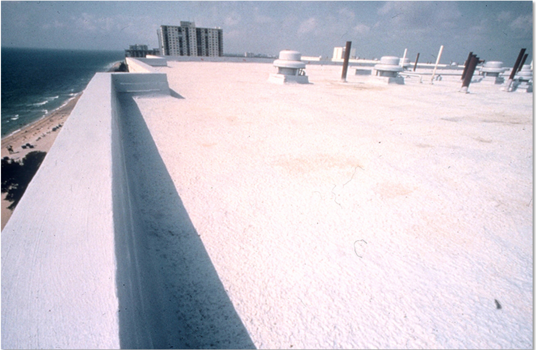
Spray applied elastomeric membrane roofing
