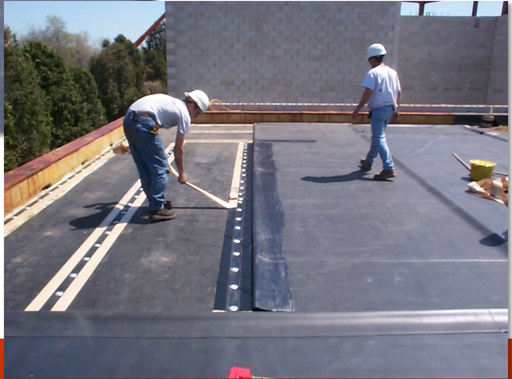
Mechanical fastening strips and an EPDM roof
