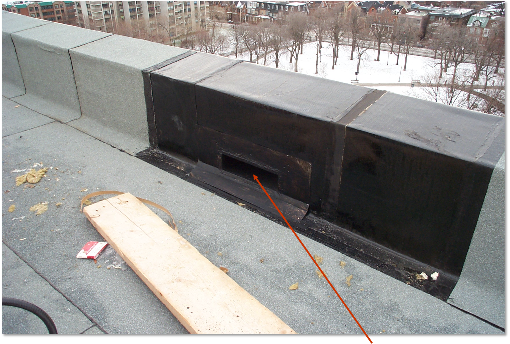
Detail at parapet. Note water overflow opening.
