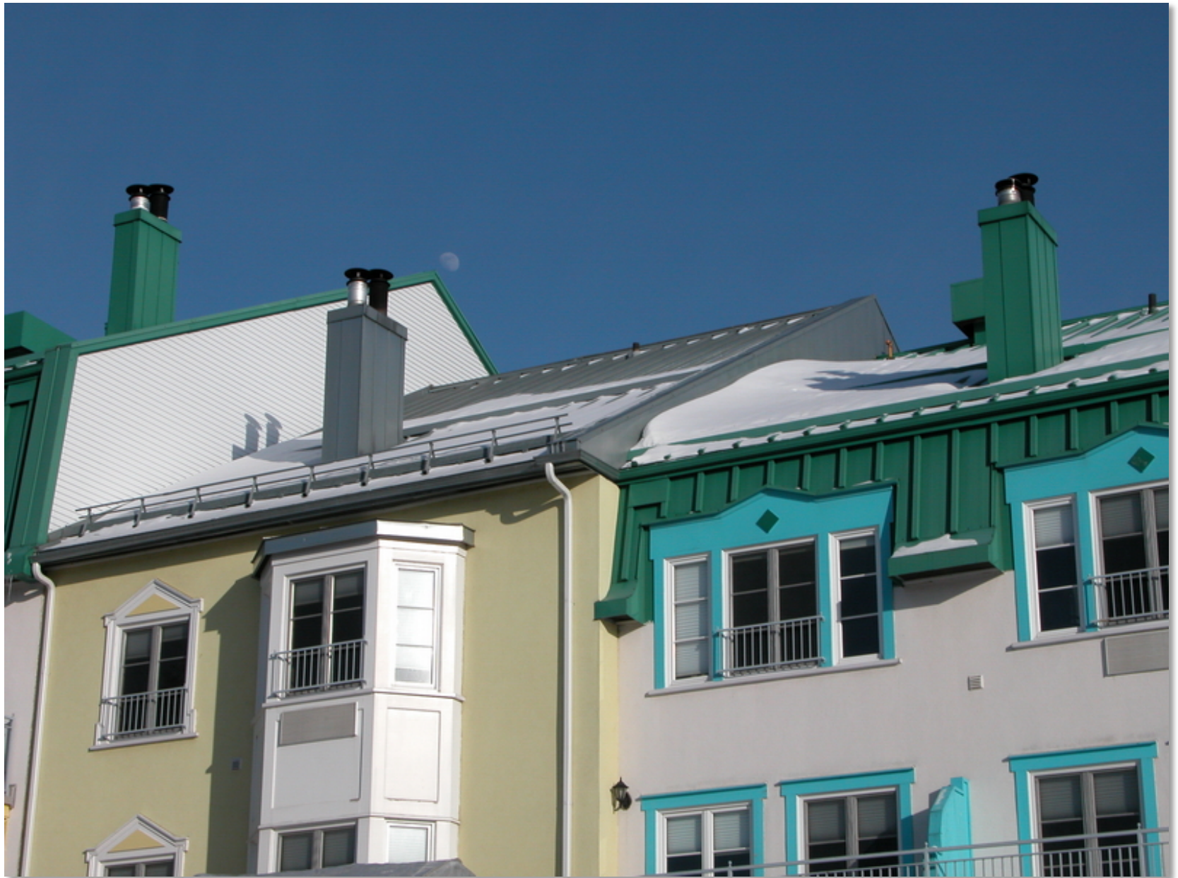
Snow guards at the edge of roofs
