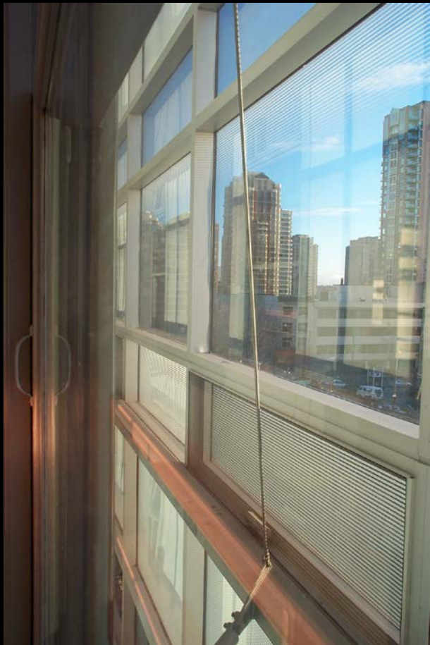
Views inside cavity
