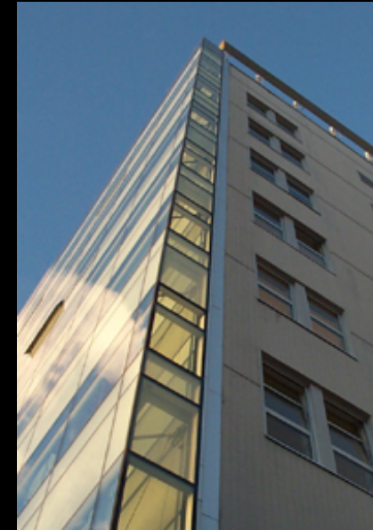
View of side of added skin
