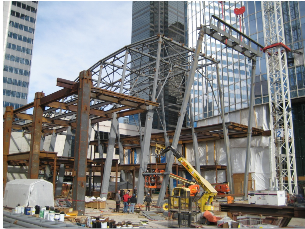
Last Arch erection
