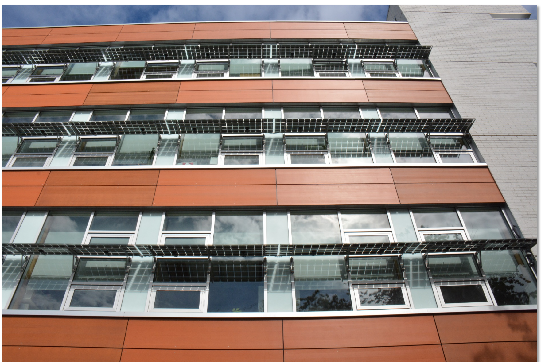
CIRS Centre, UBC – PV doubles as south facing shading device
