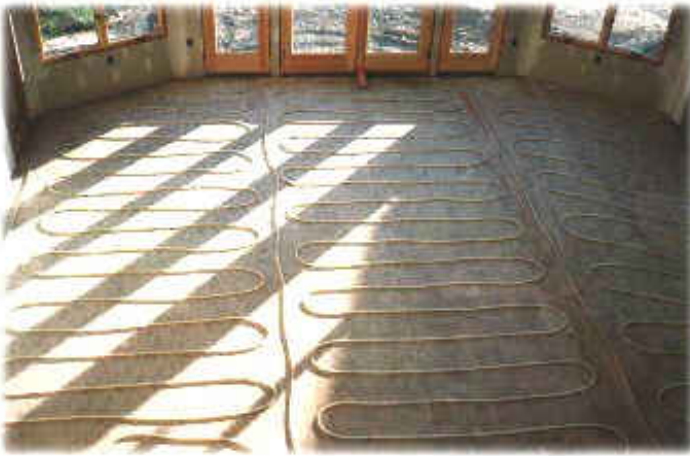
Step 1: The tubing is installed to the sub-floor of the home...
