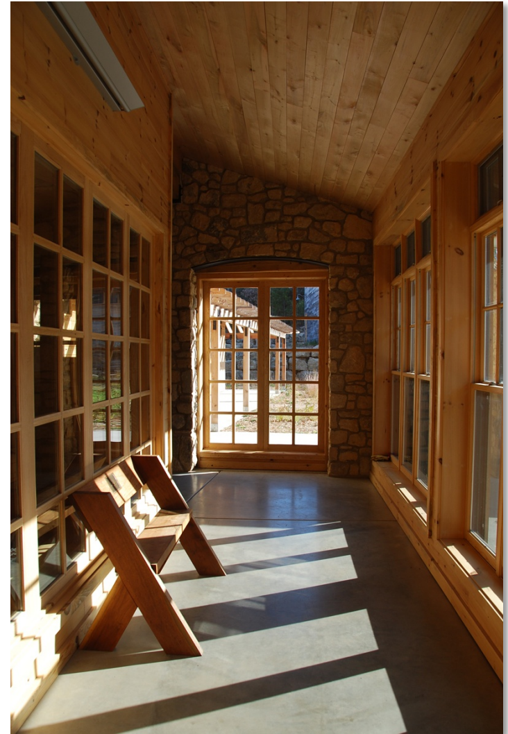
Aldo Leopold Legacy Center: Concrete floors complement the insulative wood walls
