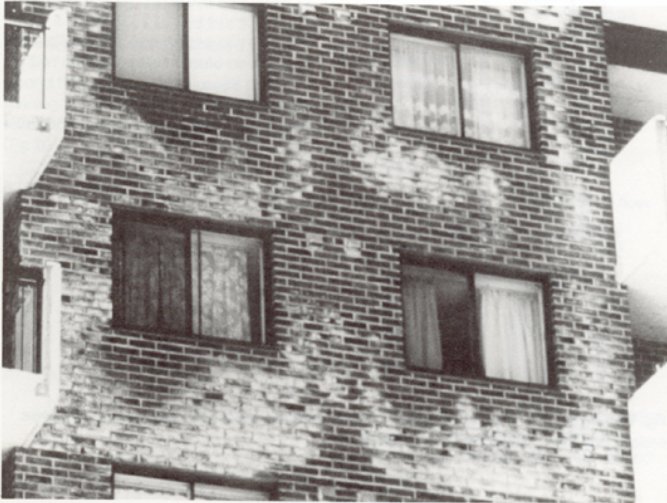
Fig. 16 An example of extensive wetness and efflorescence
