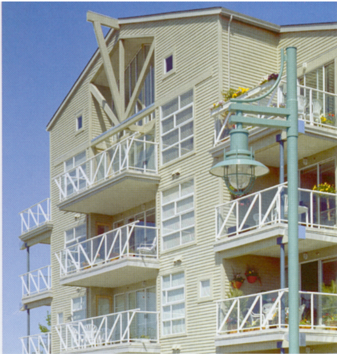
Figure 2 Four Storey Wood Frame Residential Construction
