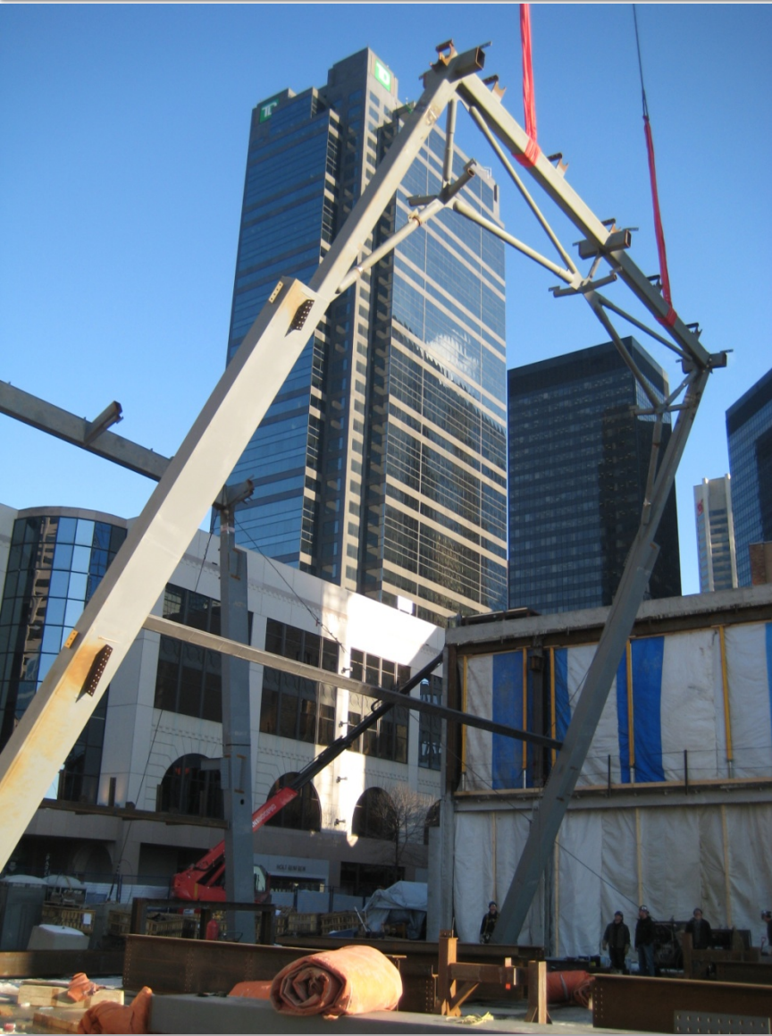
2 nd Arch erection
