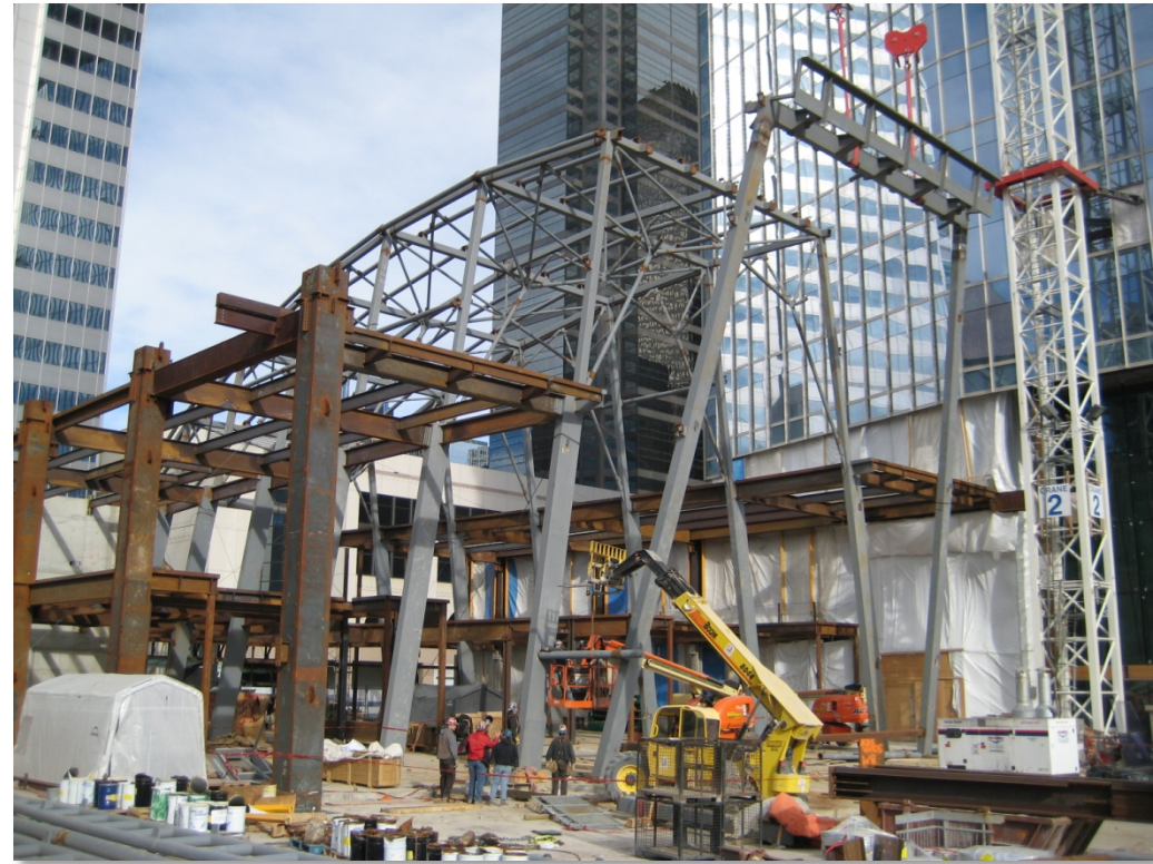
Last Arch erection
