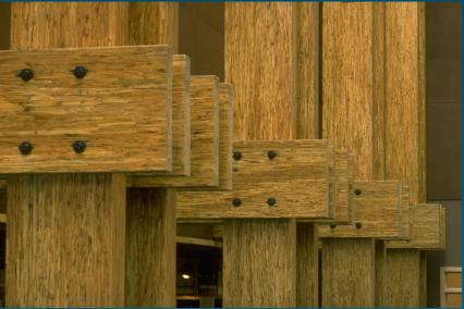
Note that the connectors are highlighted and in steel rather than nails in these connections.
