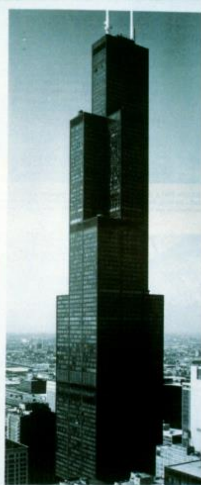
Crystal Palace would have been too heavy for its cast-iron columns; now steel beams make such buildings possible. At right is Skidmore, Owings & Merrill's Sears Tower, built out of stacked modular units.
