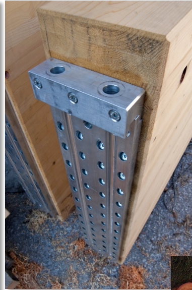
Megant fastener system for beams
