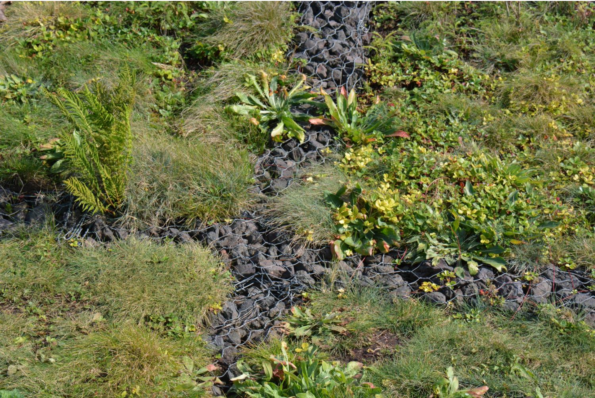
Drainage paths for excess water
