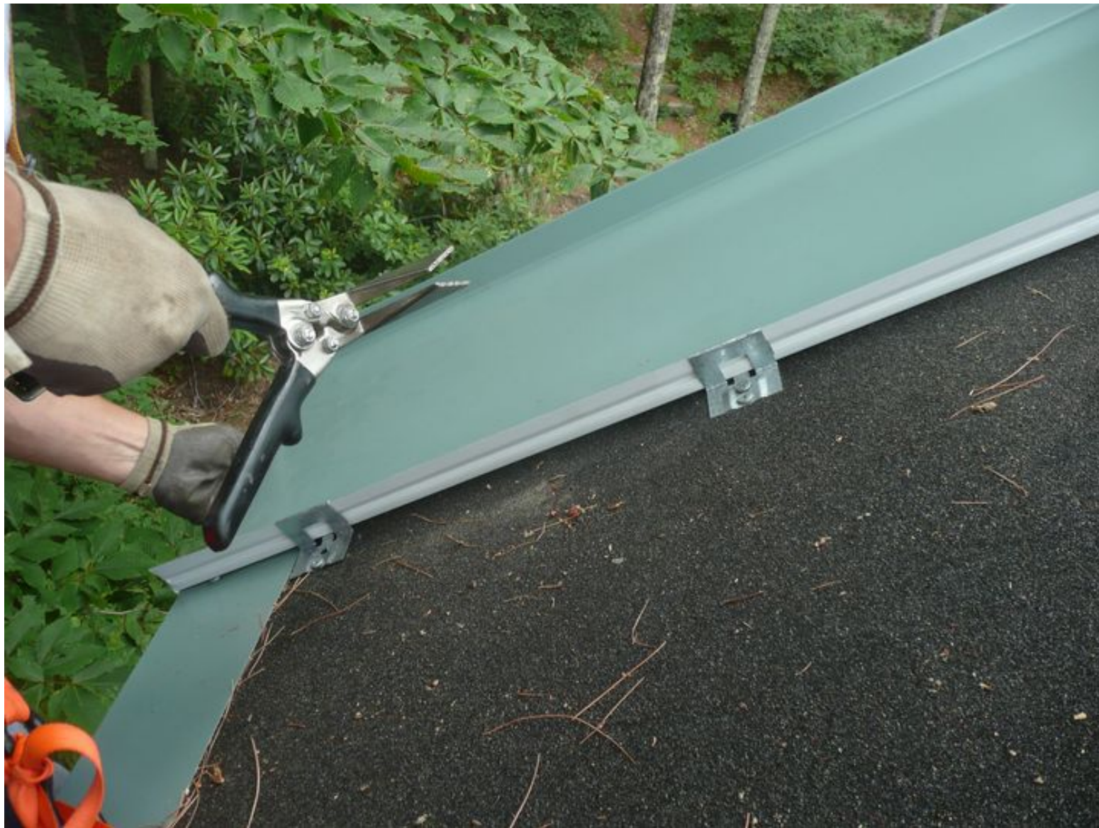
Retrofit of a commercial standing seam roof over an existing roof.
