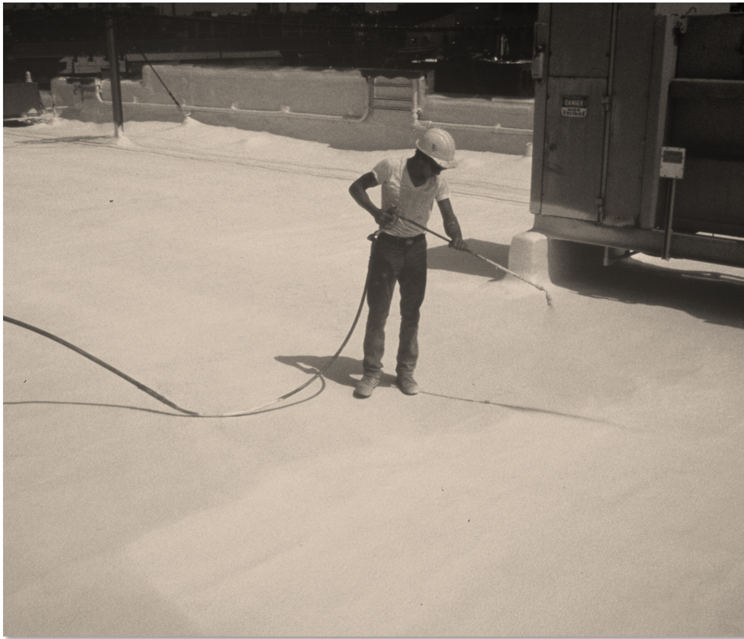
Spray applied elastomeric membrane roofing
