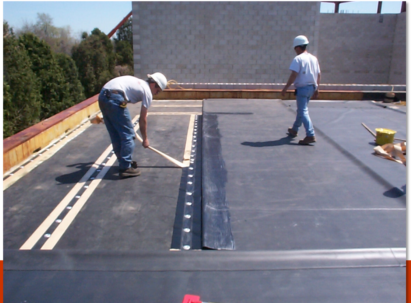
Mechanical fastening strips and an EPDM roof
