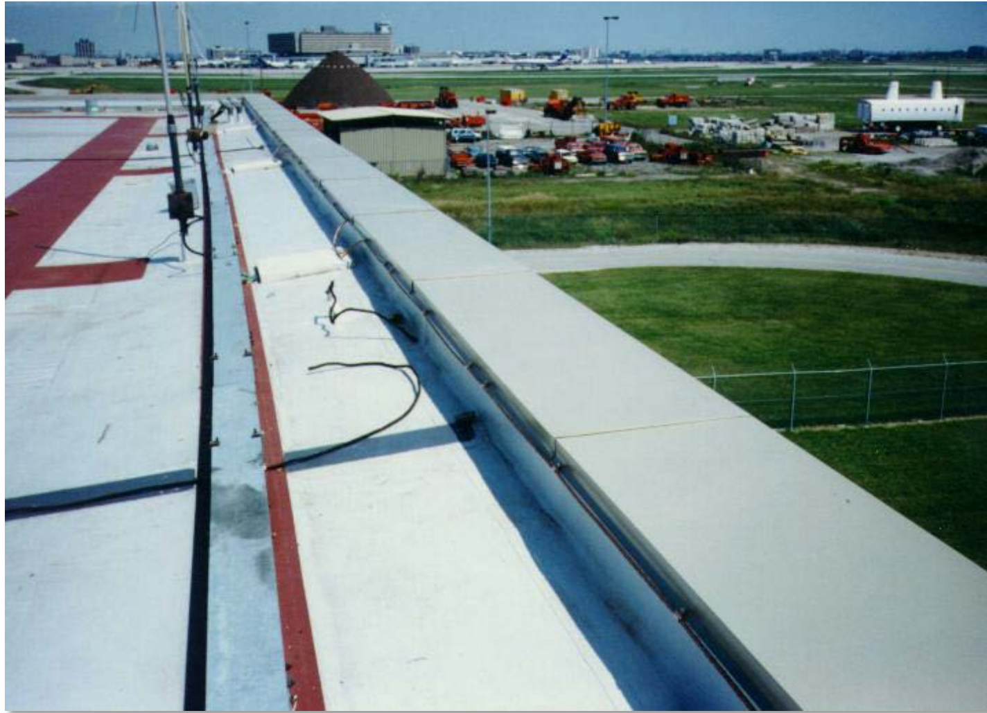
PVC Roof at Pearson International Airport
