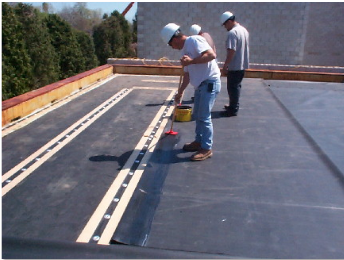
Mechanical fastening strips and an EPDM roof
