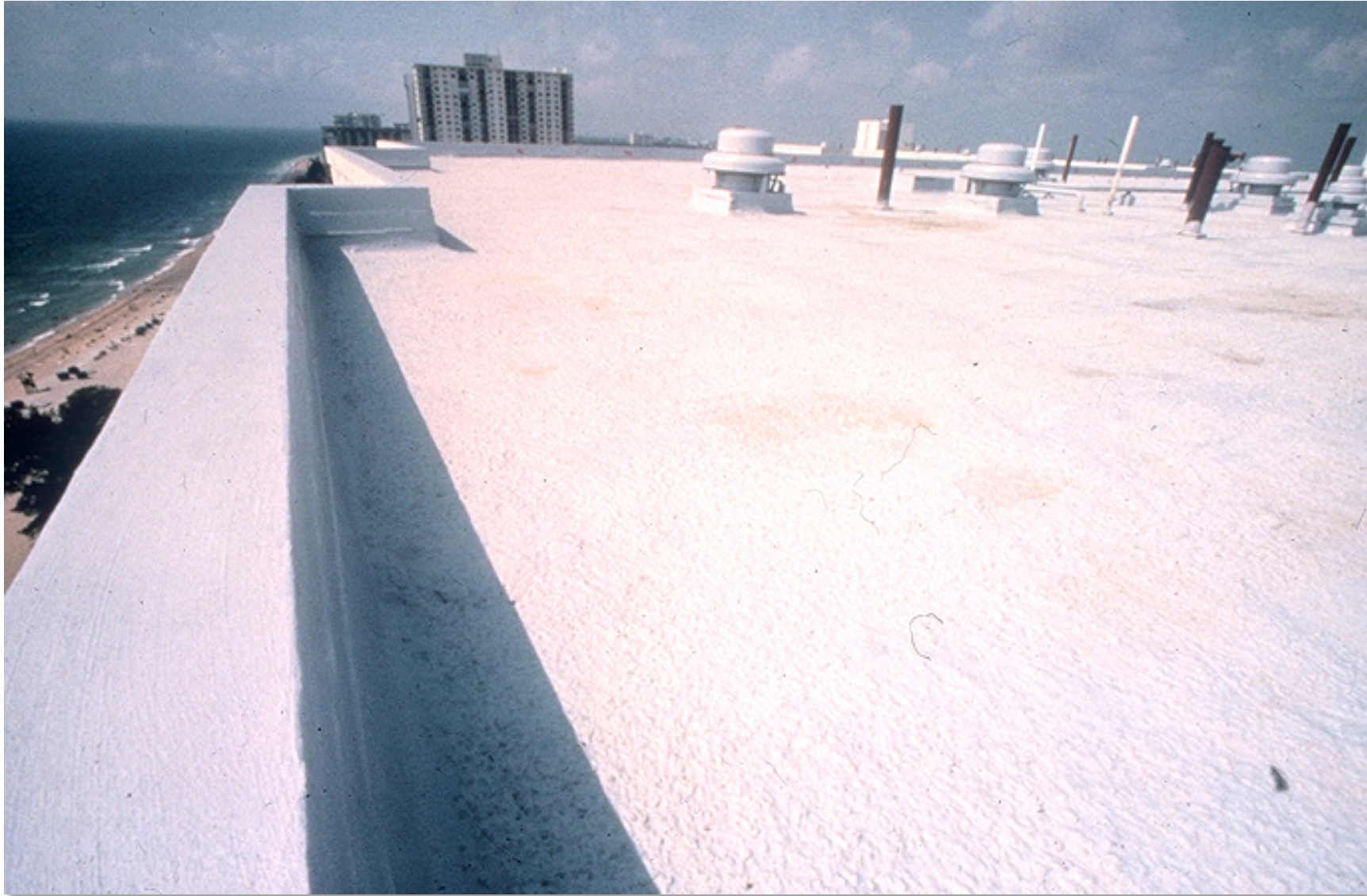
Spray applied elastomeric membrane roofing
