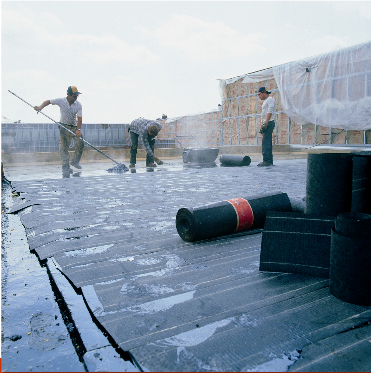
Built up Roof (BUR)
