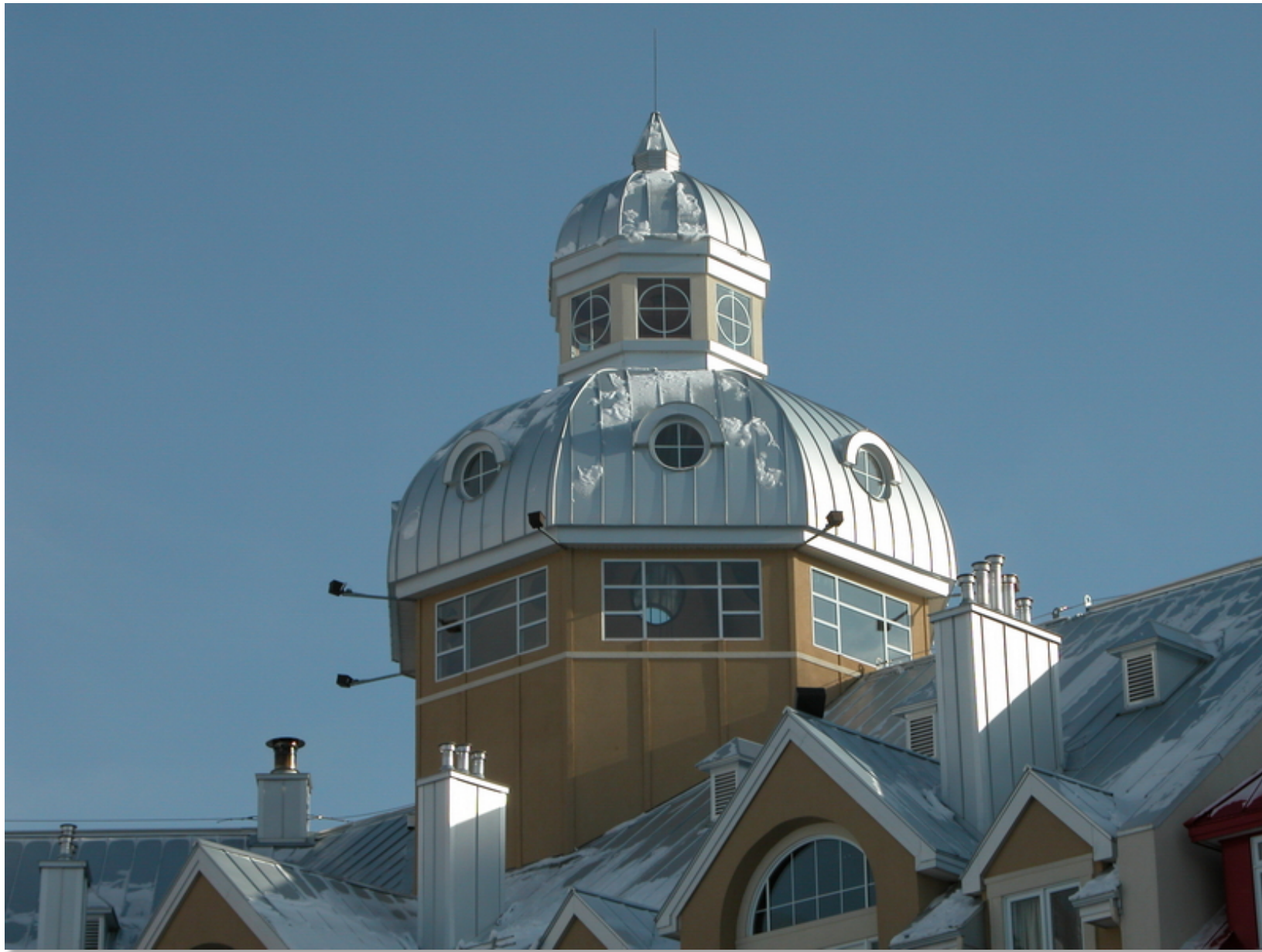
Contemporary terne-look roof in standing seam
