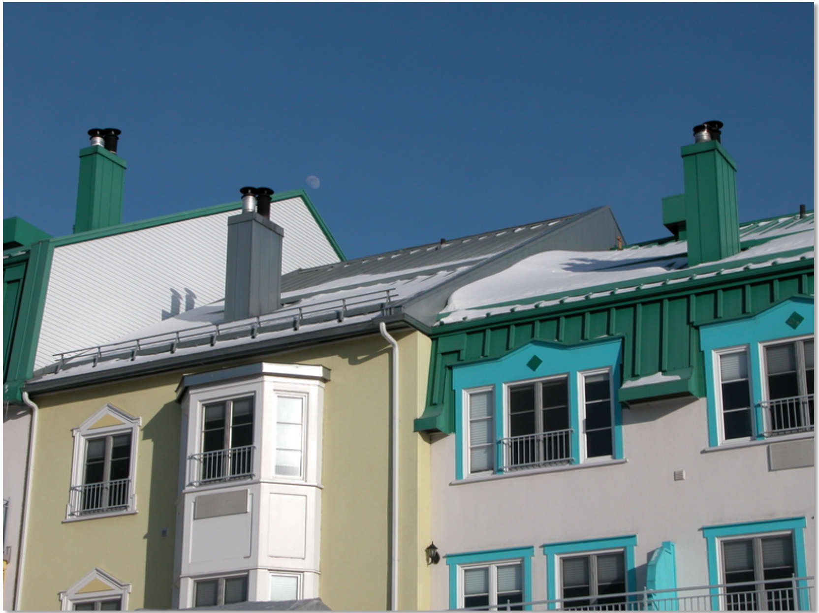
Snow guards at the edge of roofs
