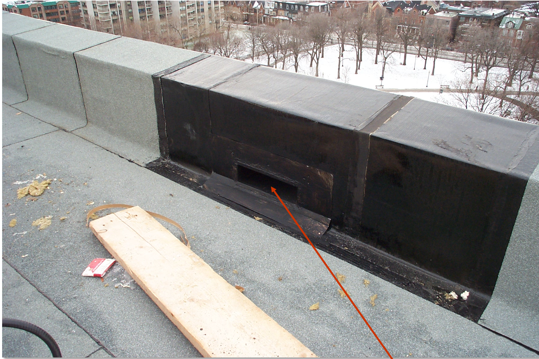
Detail at parapet. Note water overflow opening.
