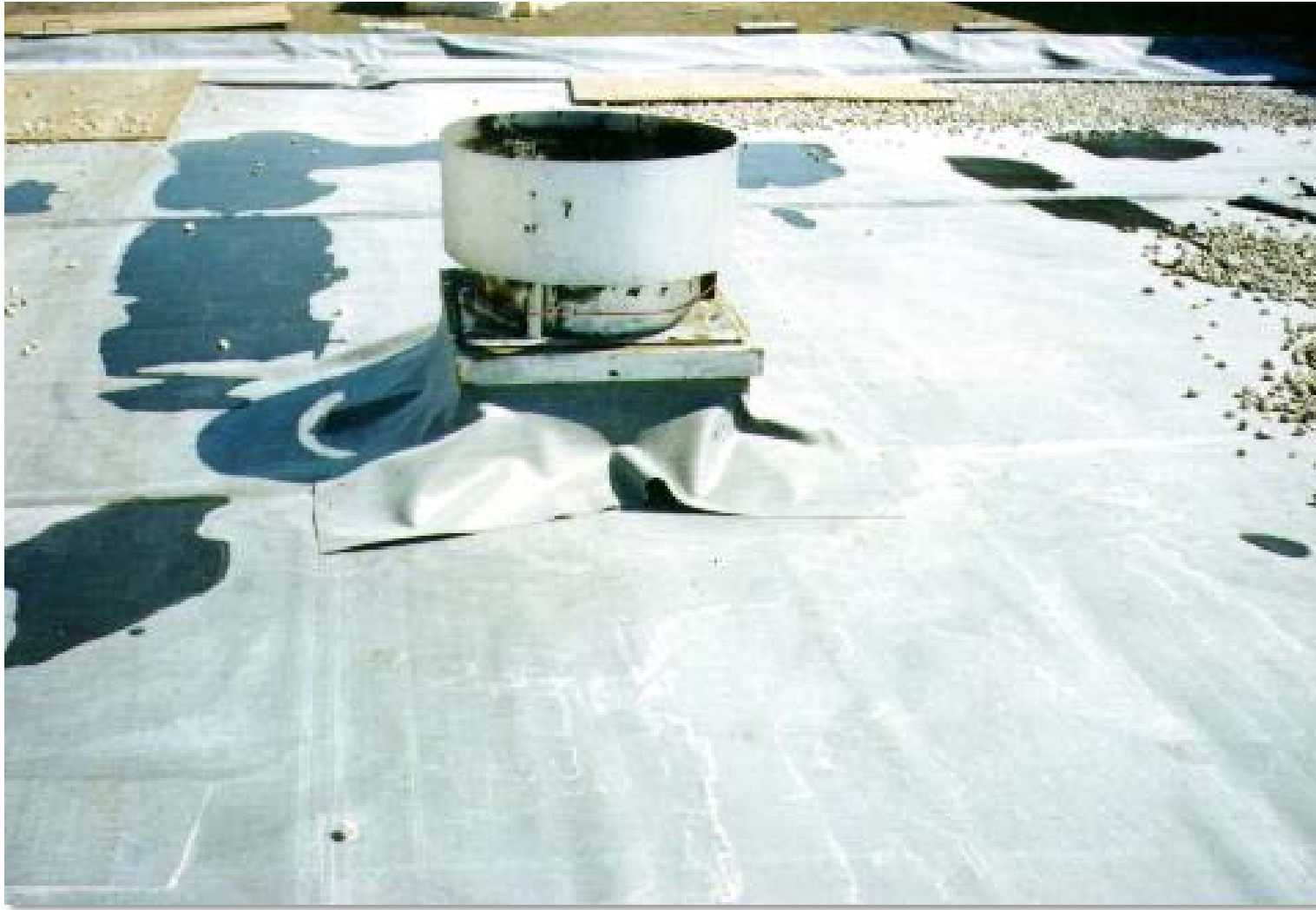
EPDM - loose laid and ballasted
