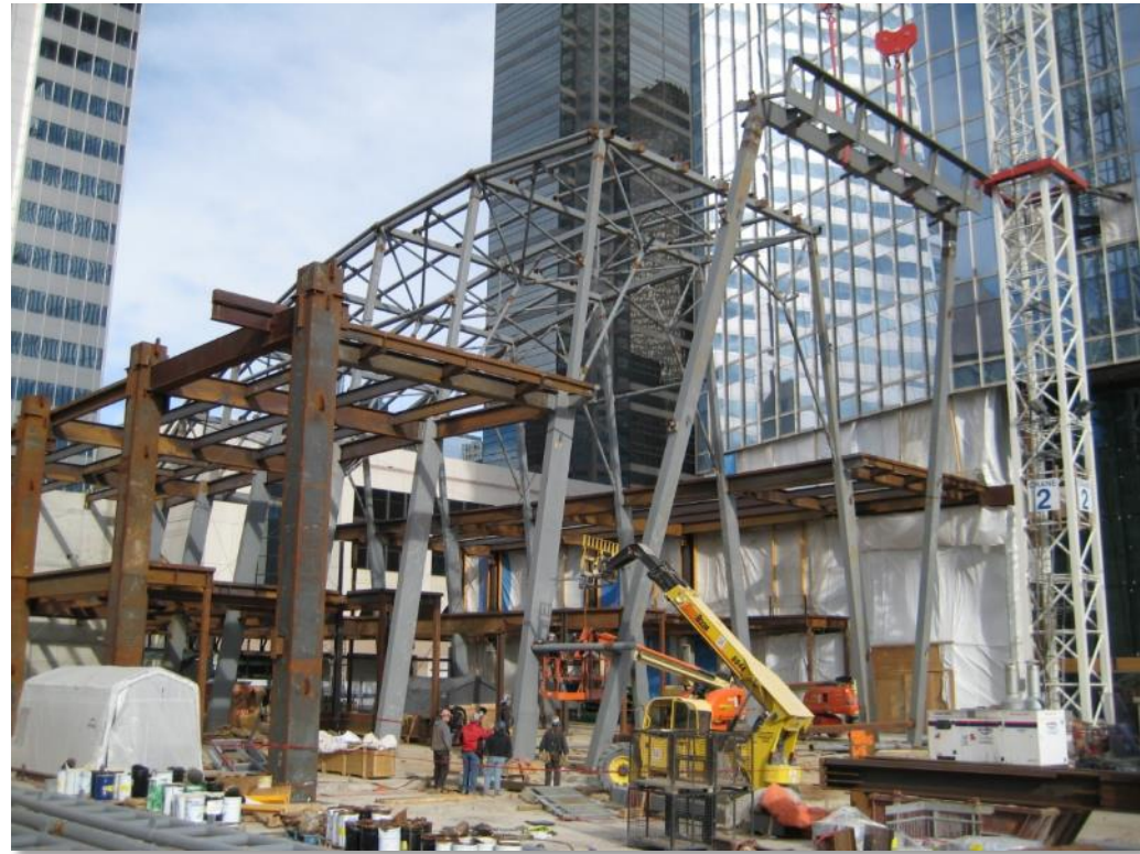
Last Arch erection
