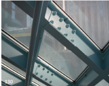
130 This building uses extensive diagrids formed with I sections. These are very simply attached using bolted splice plates on both sides of the flange.
