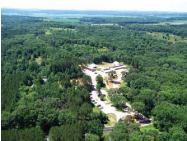
Ariel Image from South
