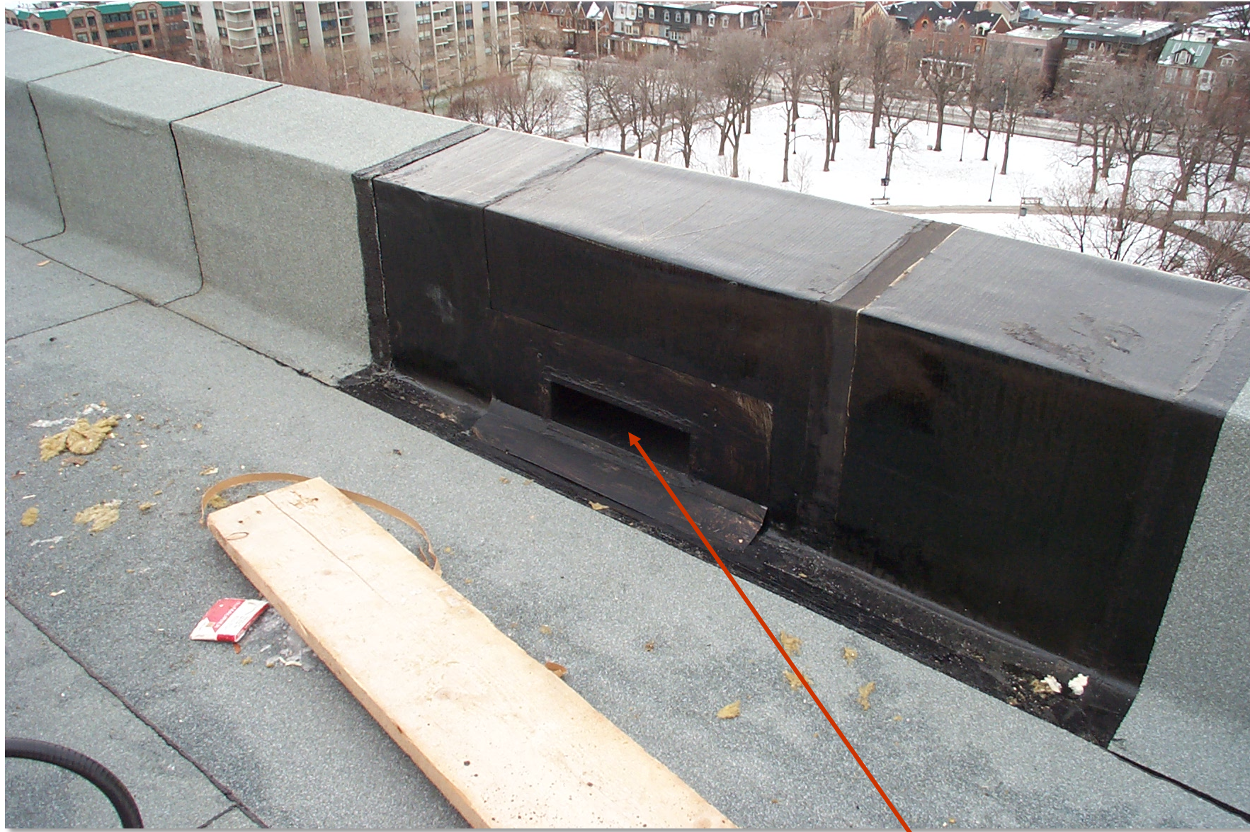
Detail at parapet. Note water overflow opening.
