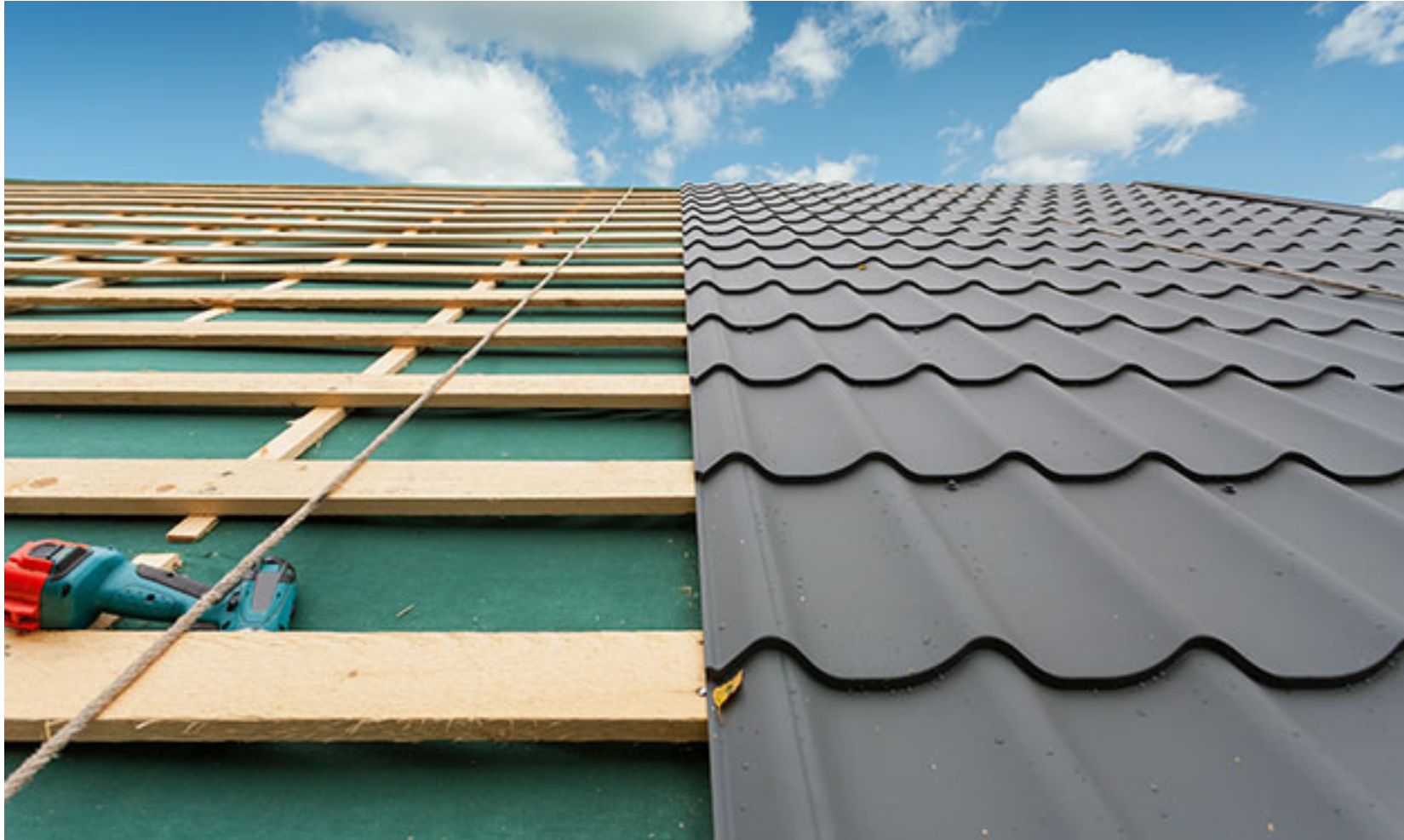
Batten mounted steel roof.
