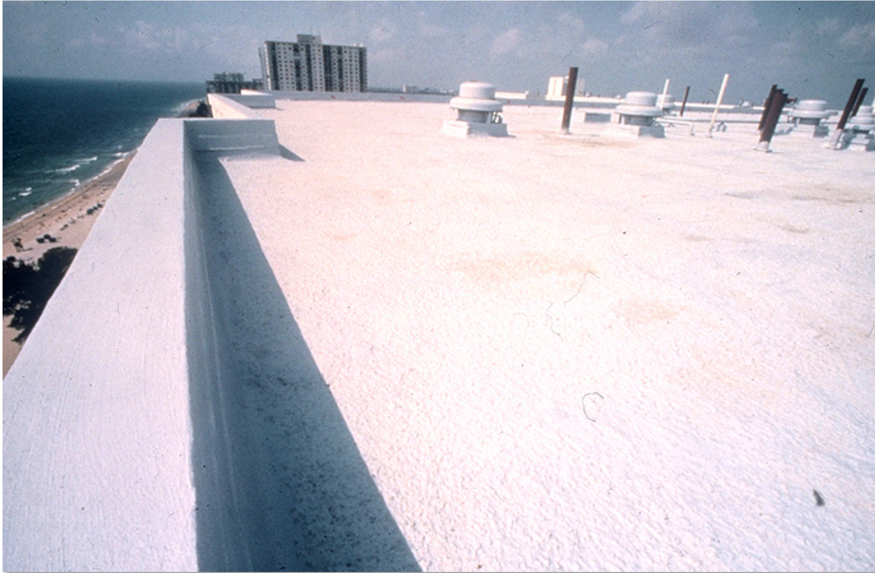
Spray applied elastomeric membrane roofing
