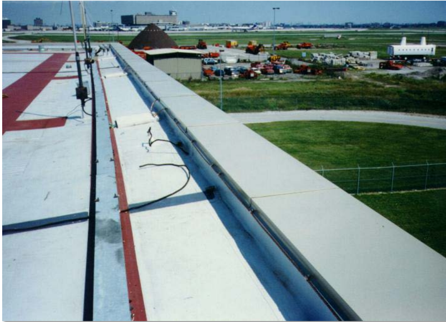
PVC Roof at Pearson International Airport
