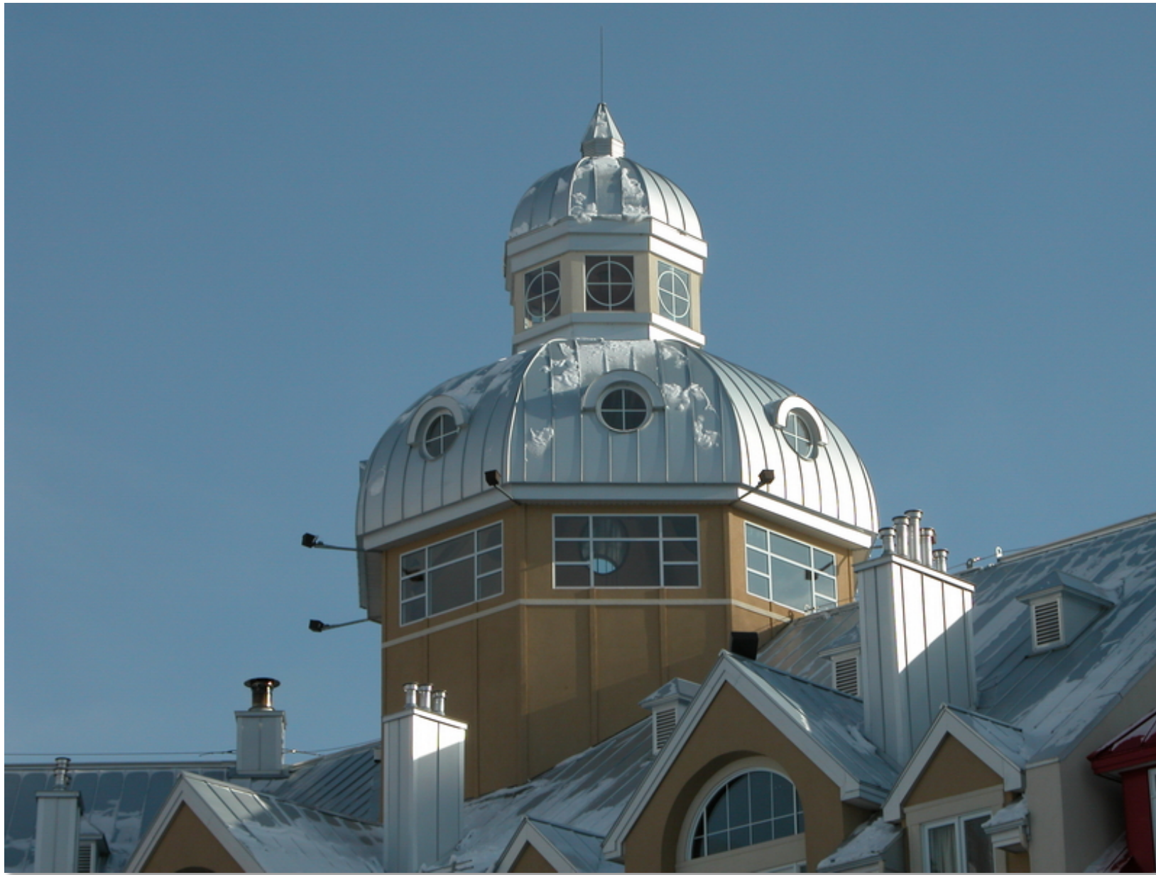
Contemporary terne-look roof in standing seam
