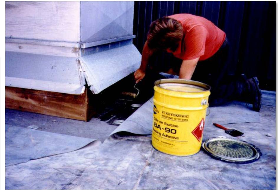
EPDM flashing
