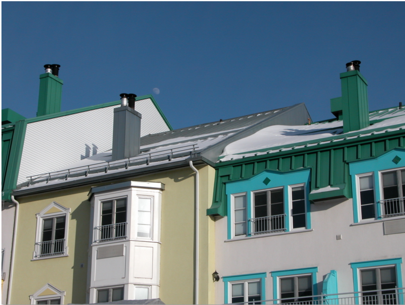
Snow guards at the edge of roofs
