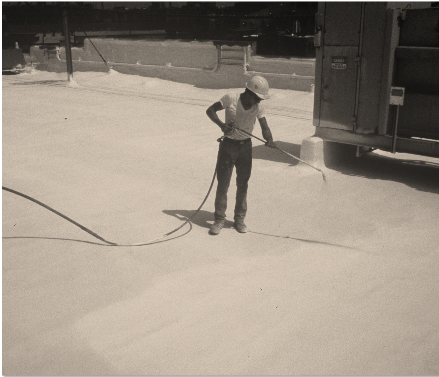
Spray applied elastomeric membrane roofing
