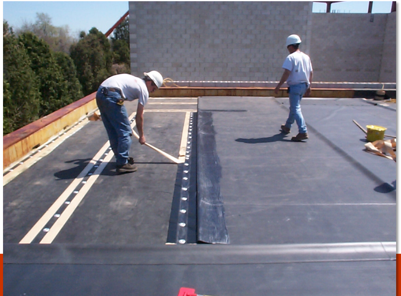
Mechanical fastening strips and an EPDM roof
