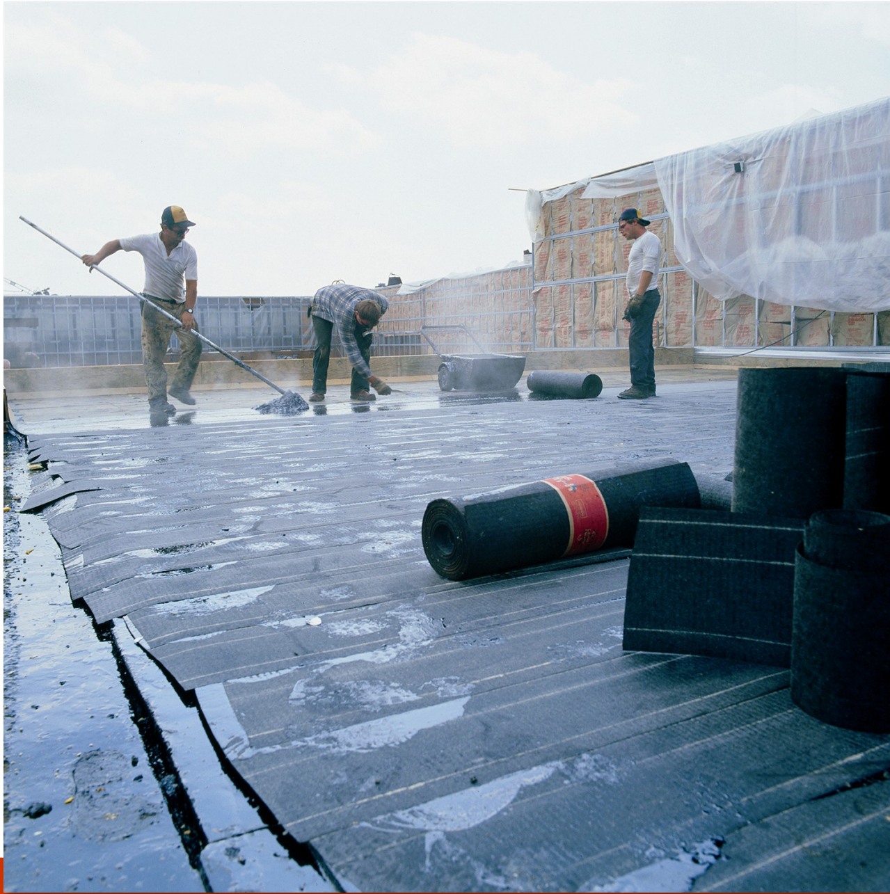
Built up Roof (BUR)
