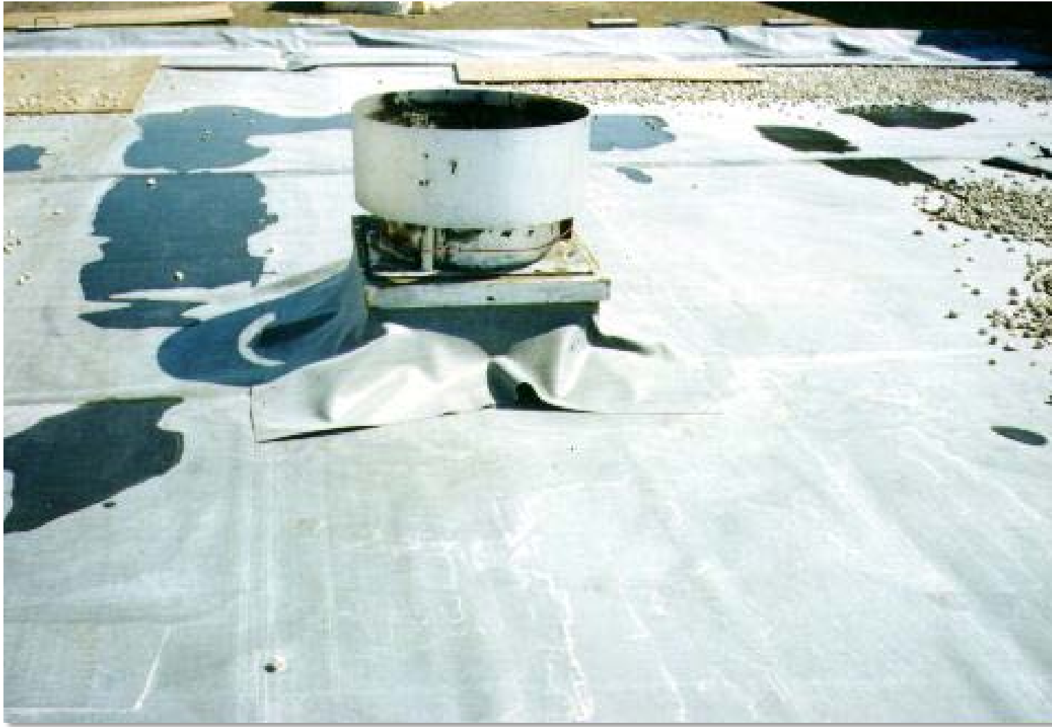
EPDM - loose laid and ballasted
