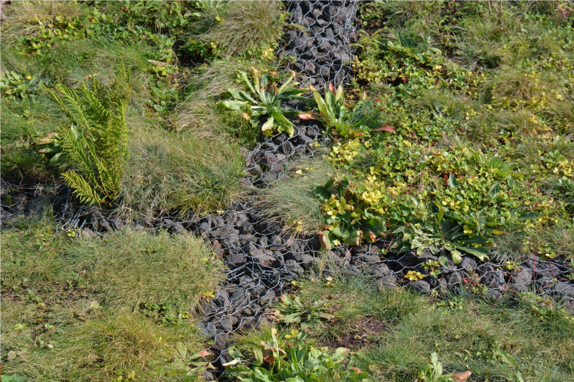
Drainage paths for excess water
