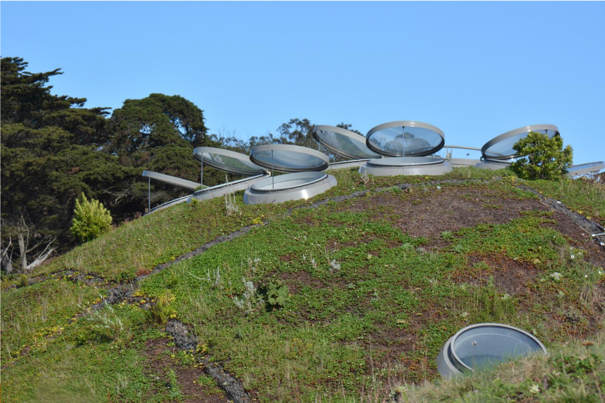
Operable skylights to vent heat from interior
