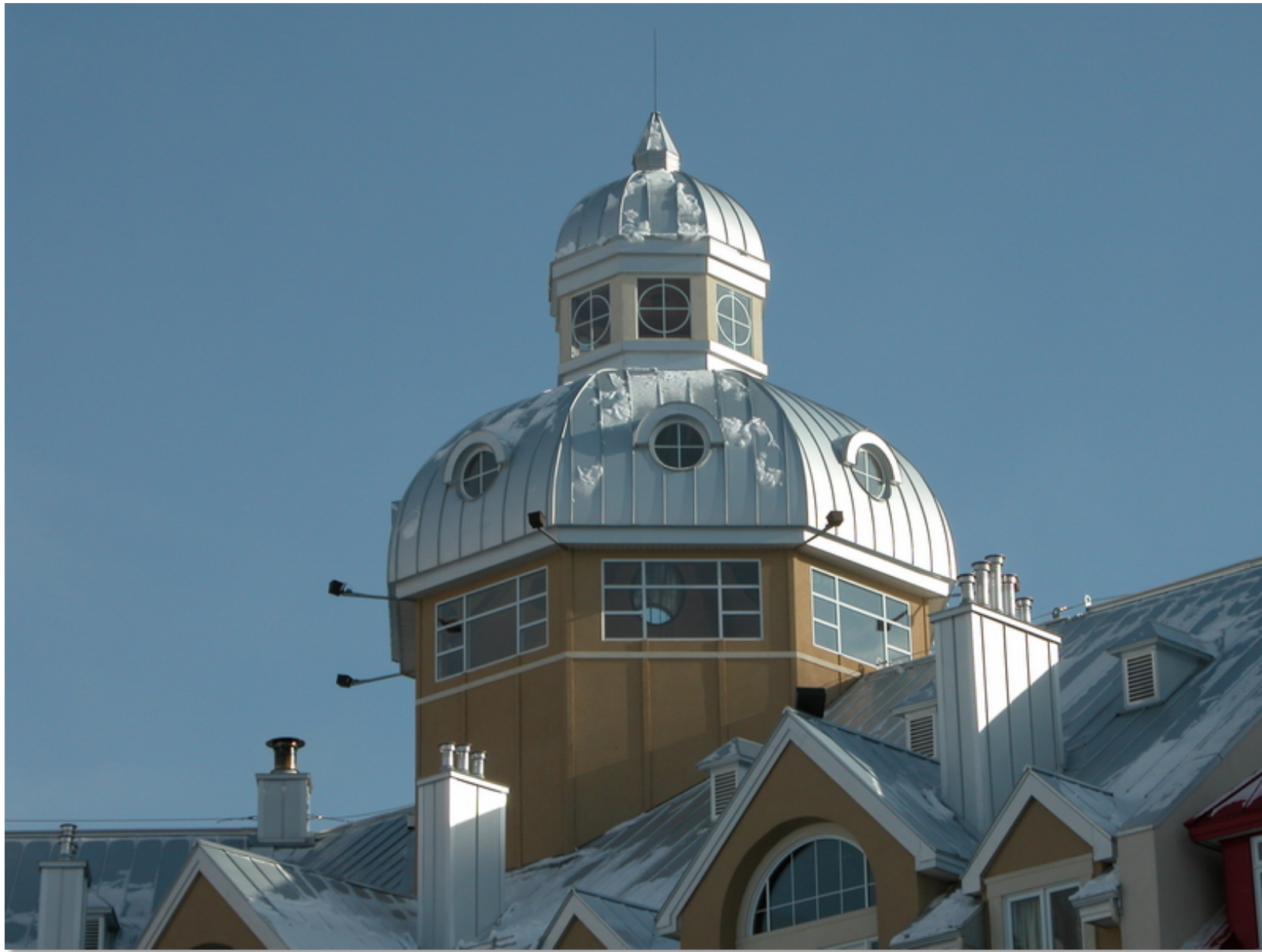
Contemporary terne-look roof in standing seam
