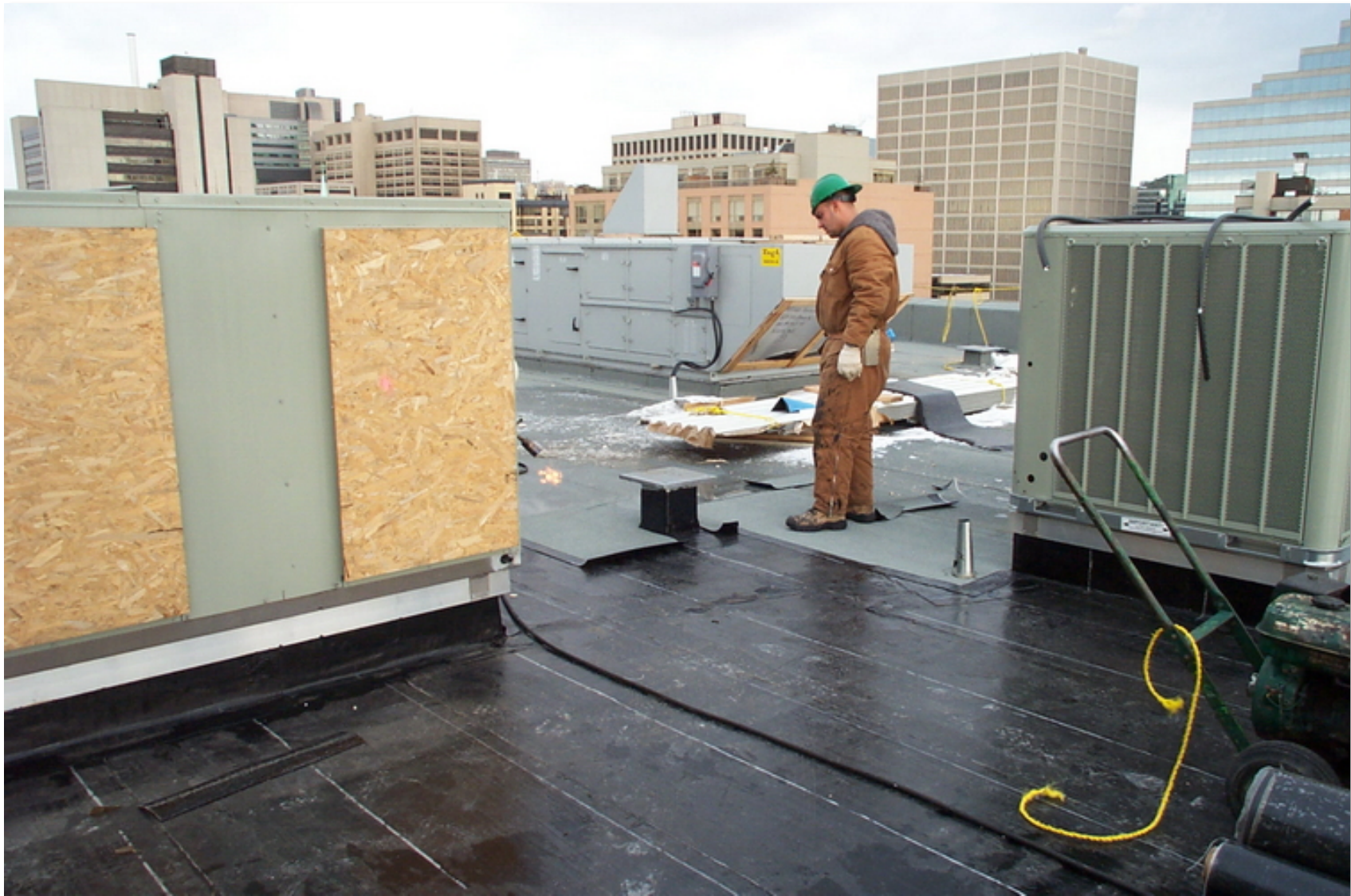
This is the roofing membrane being installed on the top of the new OCAD addition.
