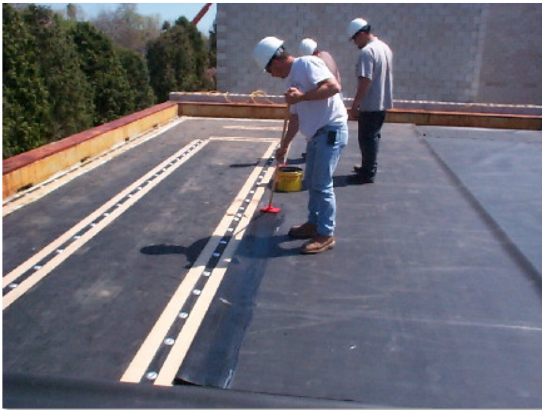
Mechanical fastening strips and an EPDM roof
