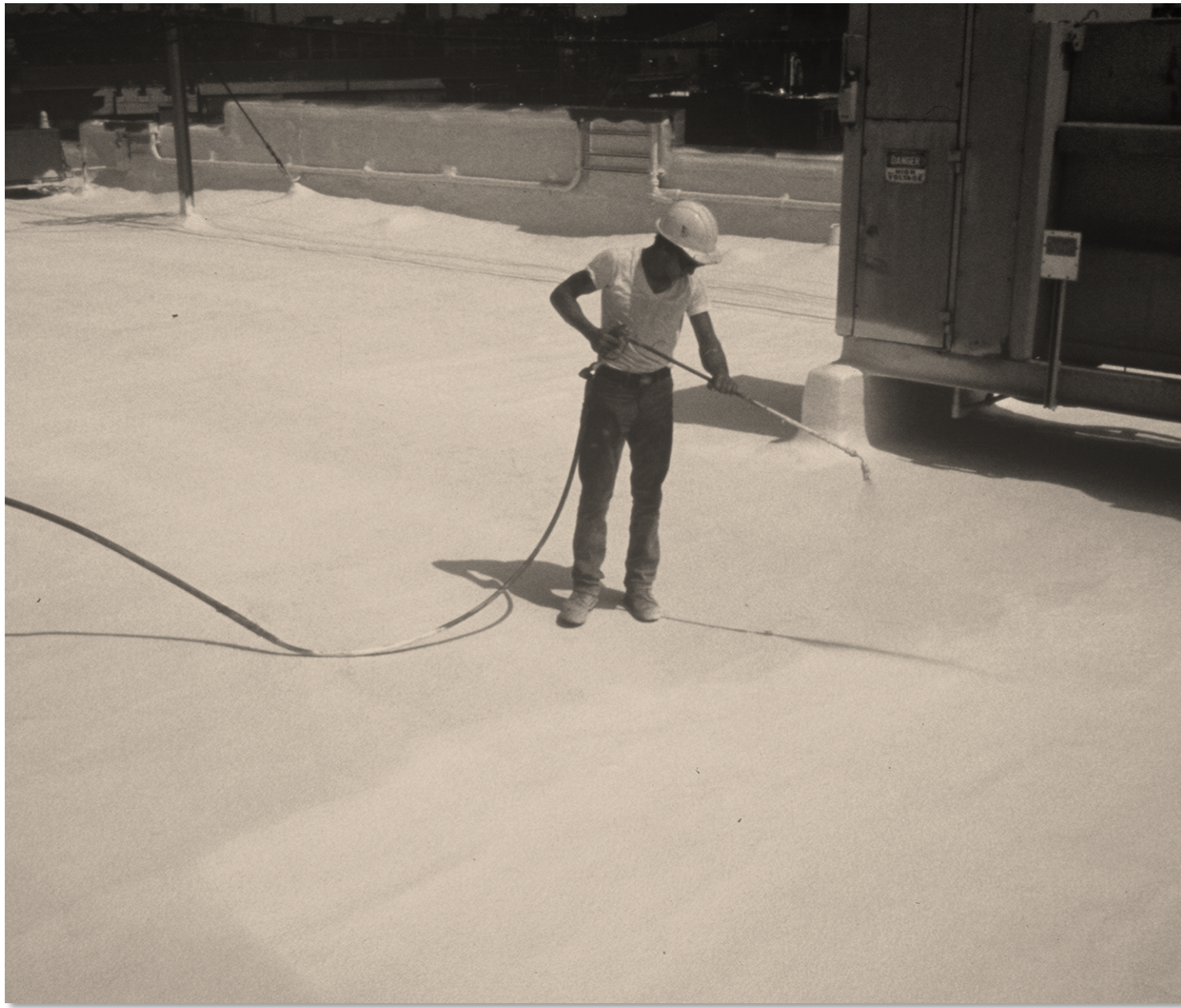
Spray applied elastomeric membrane roofing
