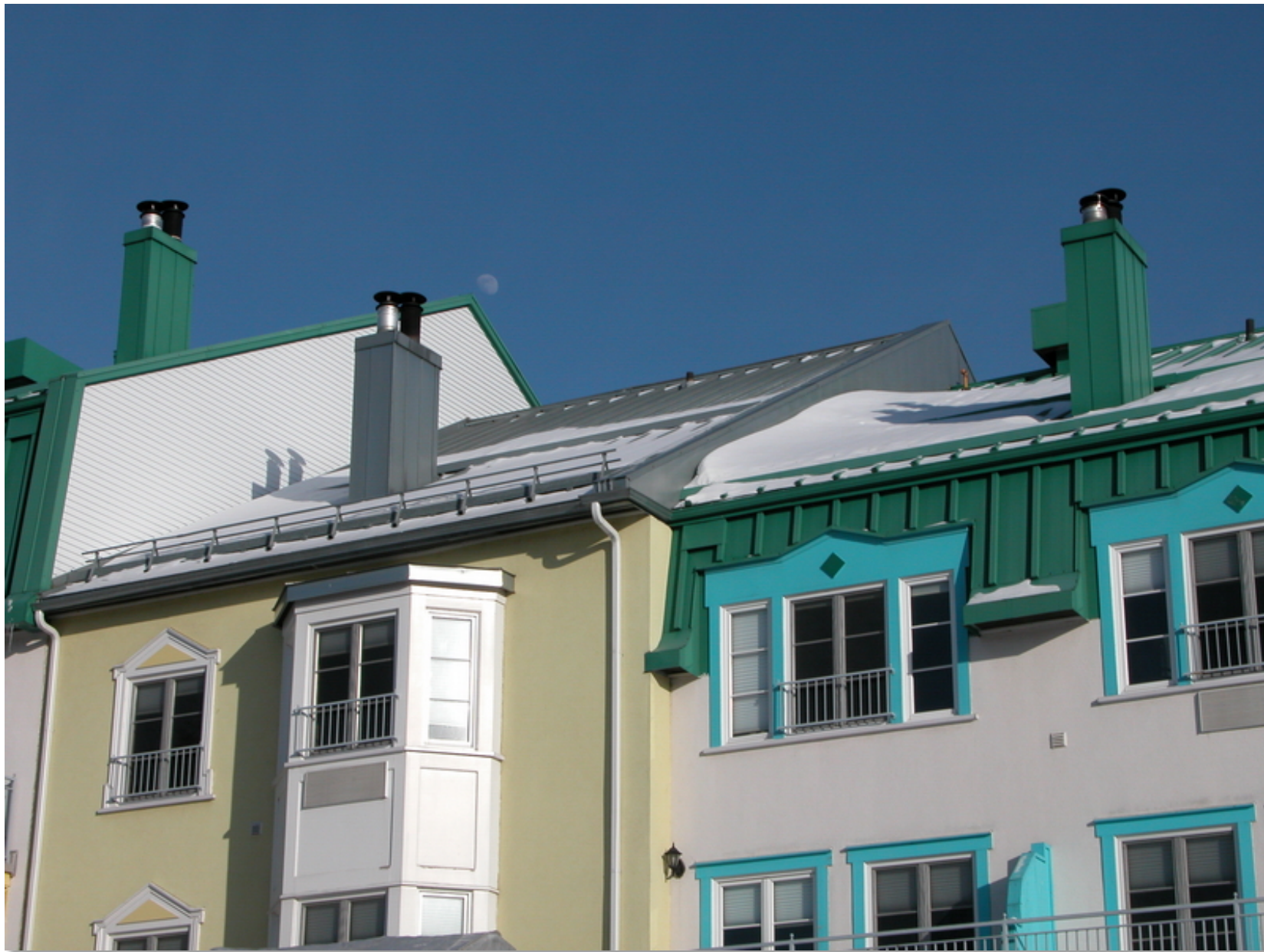
Snow guards at the edge of roofs
