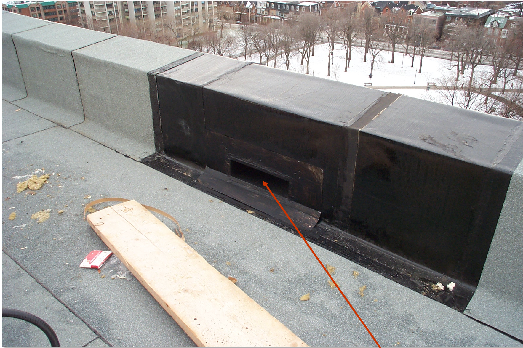
Detail at parapet. Note water overflow opening.
