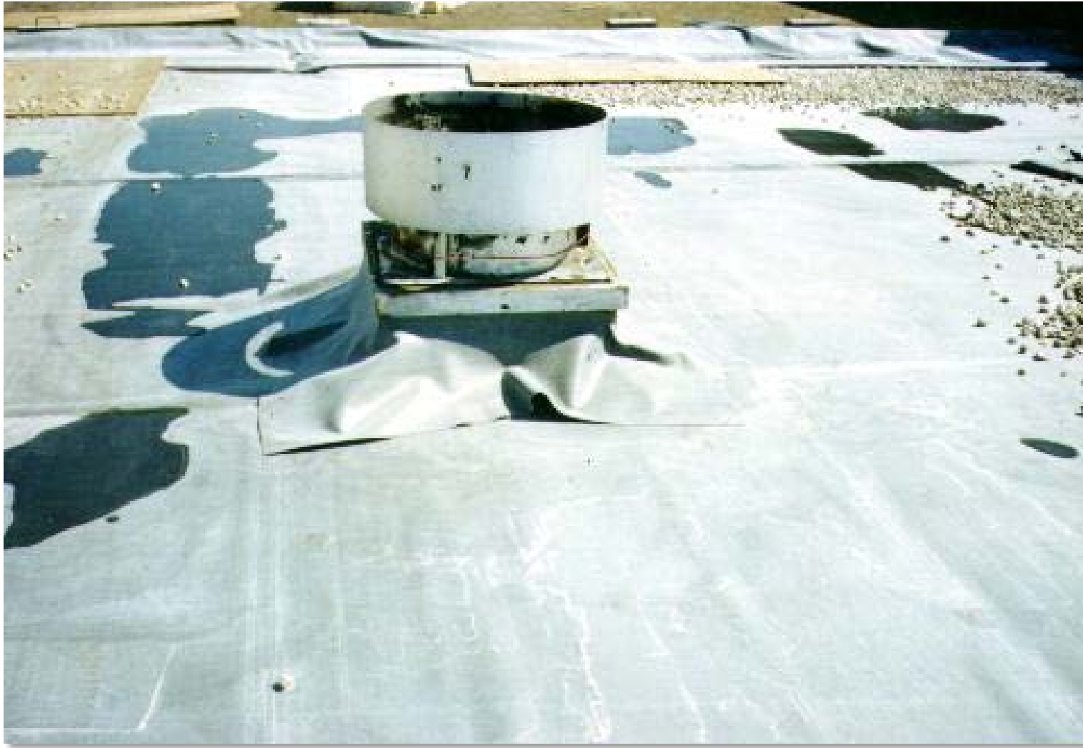
EPDM - loose laid and ballasted
