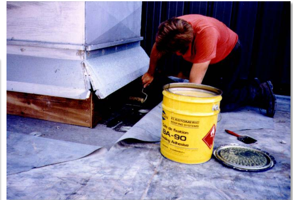
EPDM flashing
