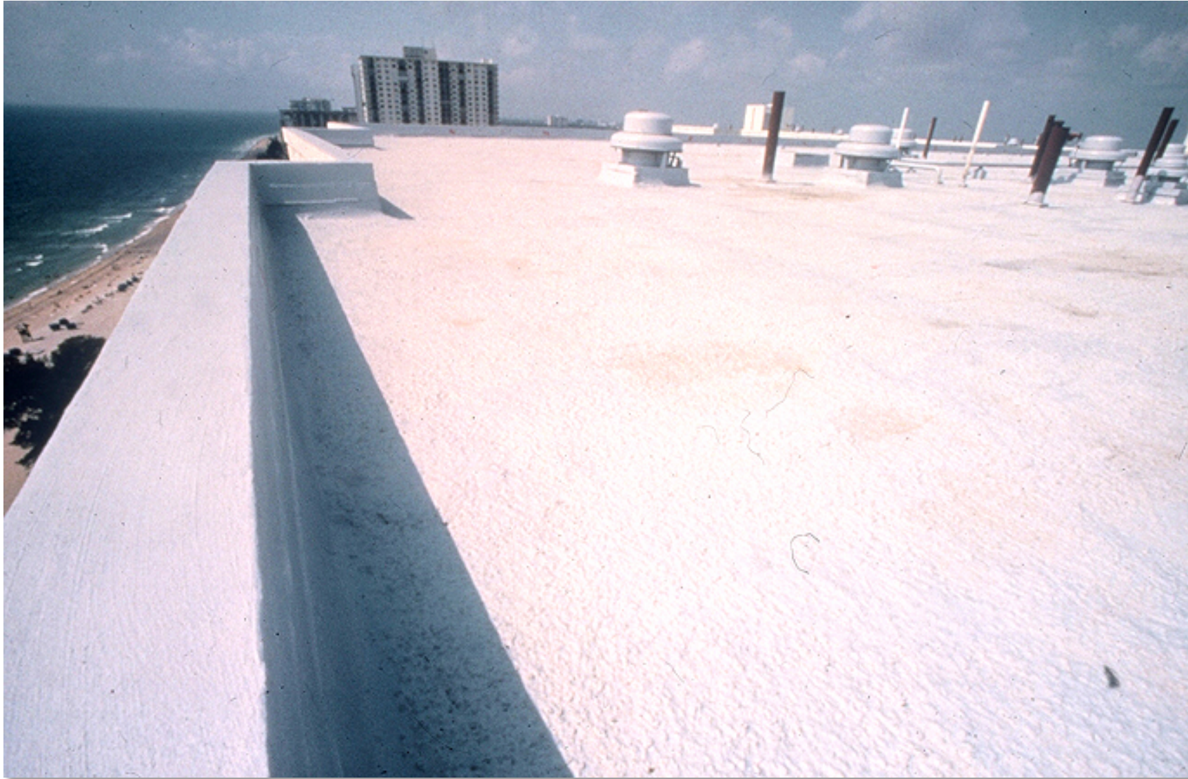
Spray applied elastomeric membrane roofing
