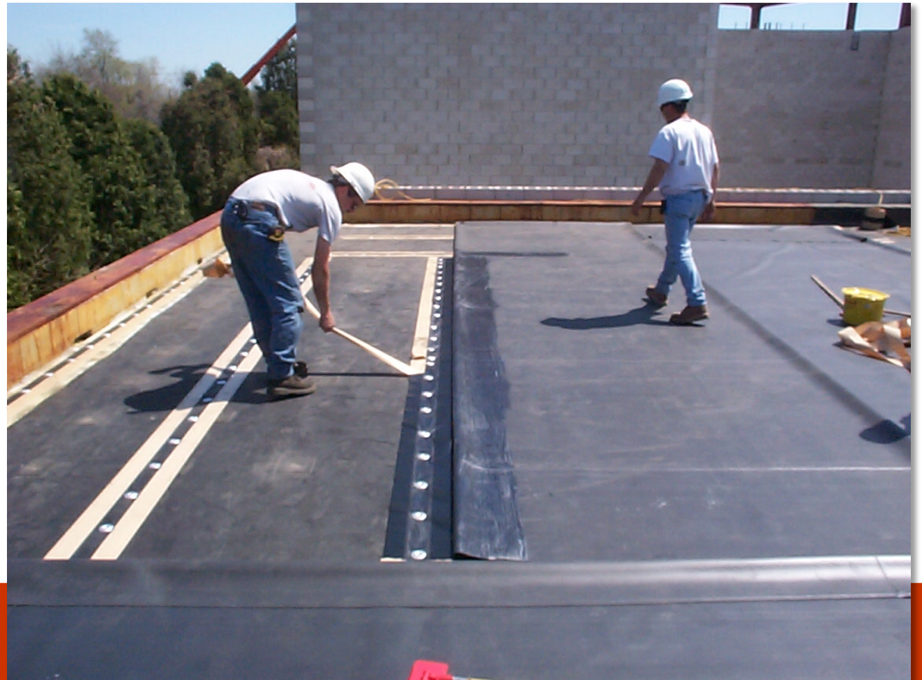
Mechanical fastening strips and an EPDM roof
