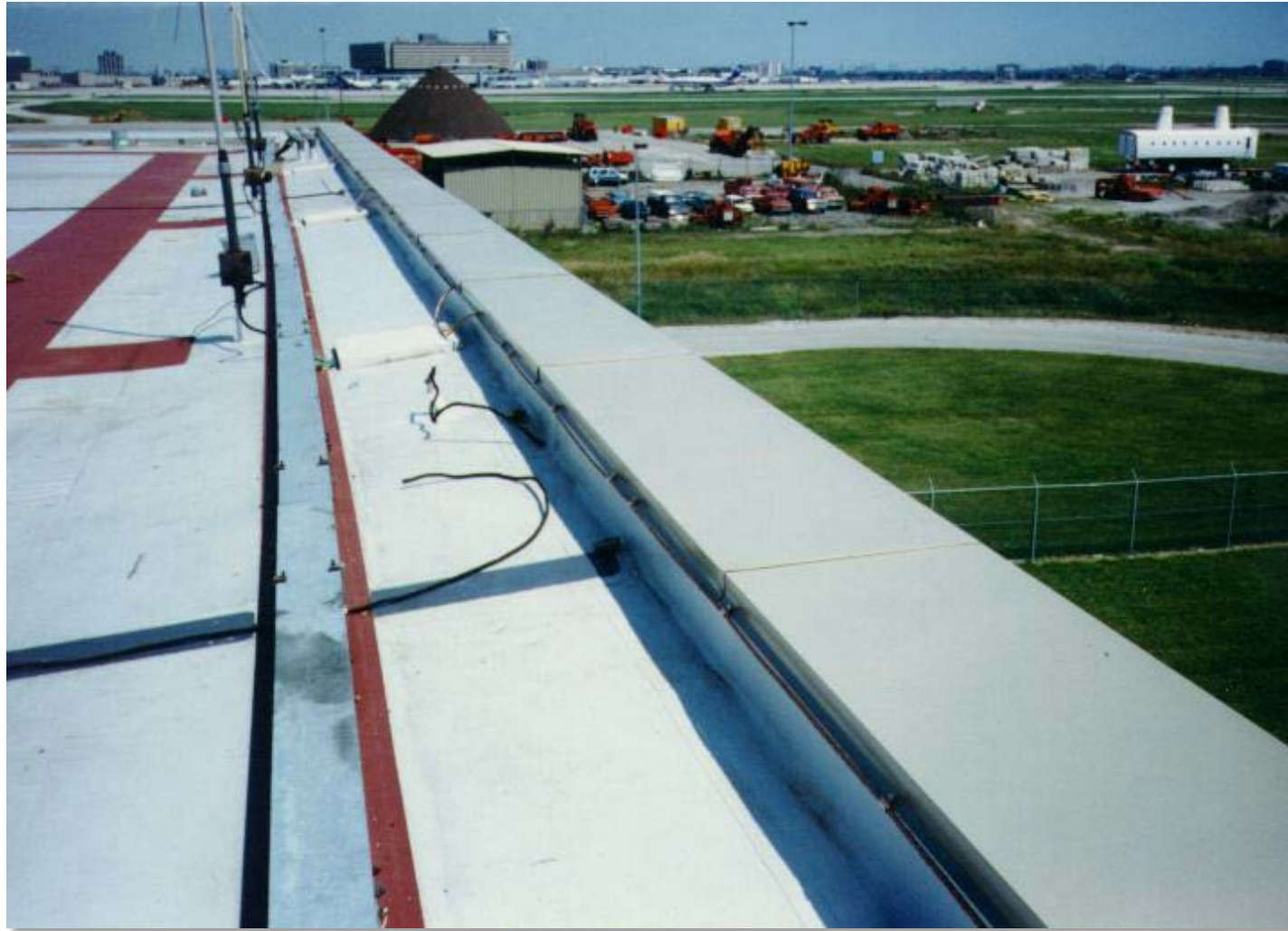
PVC Roof at Pearson International Airport
