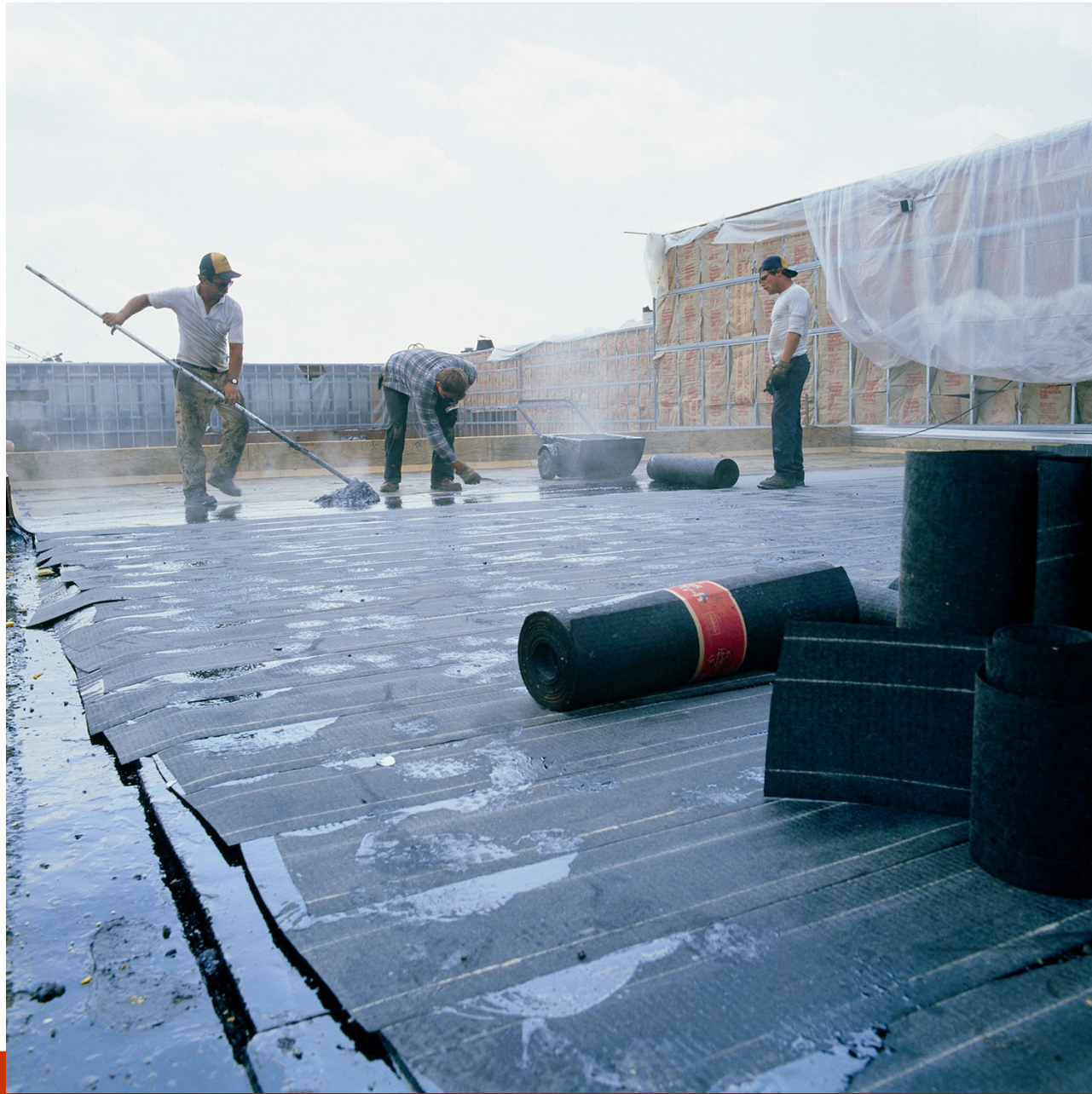
Built up Roof (BUR)
