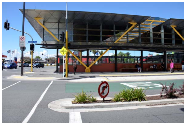
Figure 5: The New Lynn Transit Station in Auckland, New Zealand uses AESS effectively to create Award Winning architecture. The diagonal braces could easily provide the basis for a “seismic aesthetic” if modified for that purpose.
