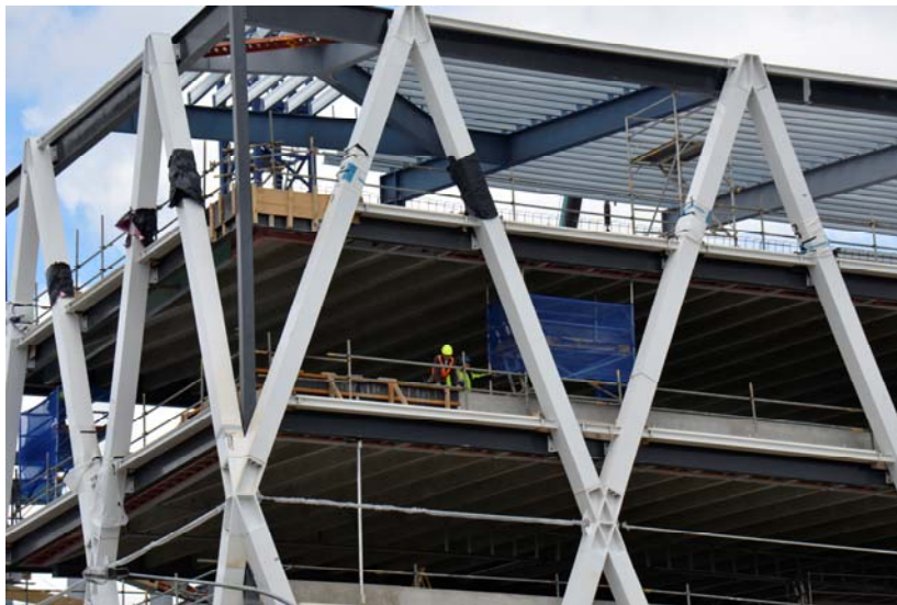
Figure 10: The Manukau Institute of Technology in Auckland, New Zealand designed by Warren and Mahoney Architects uses a perimeter diagrid on its exterior to purposefully express the structure. Note the absence of vertical columns. EBFs are used on the building interior to assist with seismic resistance. These are left exposed.
