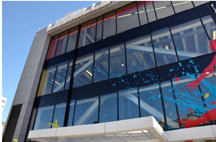
Figure 4: Exposed bracing at the Lesmills Fitness Centre in Christchurch.
