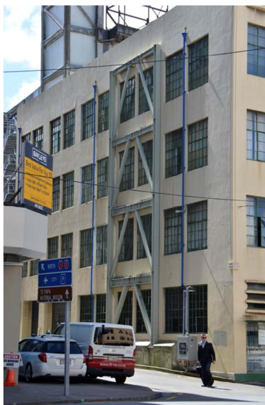
Figure 8: Existing seismic retrofit in Wellington, New Zealand.
