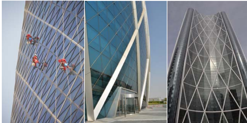
Fig. 4: Capital Gate, Abu Dhabi (left) has a small module and uses a triangular window system that accommodates operable windows. Aldar HQ, Abu Dhabi (center) has a larger module and also employs a triangular system. Bow Encana, Calgary (right) has the largest module and the faceting of the structure allows for the use of a rectilinear glazing system.
