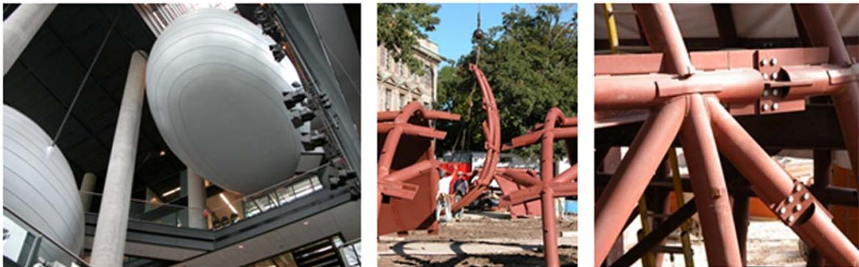
Figure 3. (clockwise from top left): Classic connection, detail from F. Ching of a type of tube to W connection, detail of tube to tube connection with plate on the Leslie Dan School of Pharmacy, crane lifting pod segment for placement, and finished building – pods clad in gypsum board with painted finish
