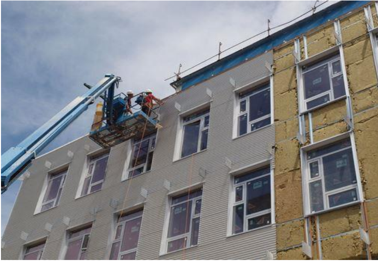
Figure 9: Insulation, Brick Work
