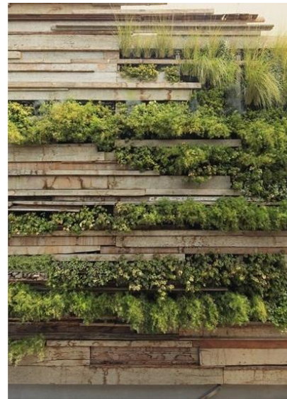
Figure 12: Living Retaining Wall, Lima
