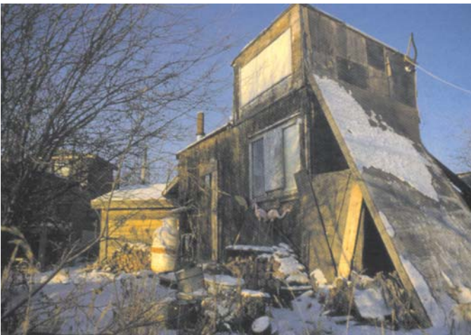
Shack located in 'the woodyard' Old Town. image from Yellowknife Diamond in the Rough p31
