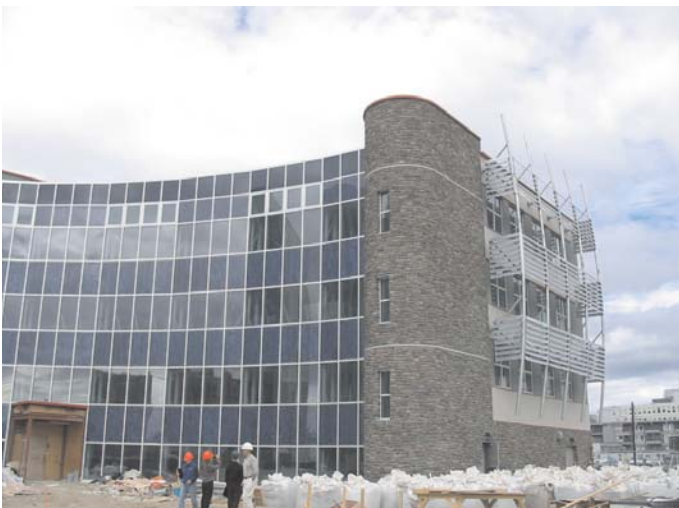
New federal government building located downtown Yellowknife. Note photovoltaic panels and sun shading device. Expected to receive LEED silver. Architect: Manasc Issac image: author
