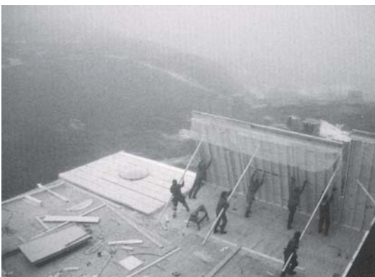
Platform framing in Rankin Inlet Image from Bare Poles p 124
