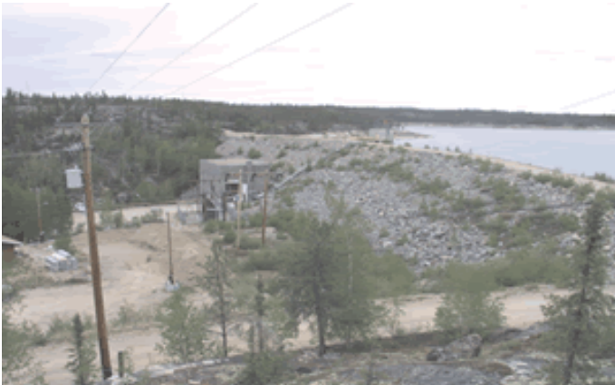
Snare Hydro Project image from http://www.ntpc.com/grey/supply/hydro.html
