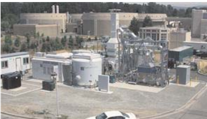
Four large digester tanks sit behind the fuel cell power plant at the wastewater treatment plant in Renton, Wash. image from: http://www.msnbc.msn.com/id/5335635
