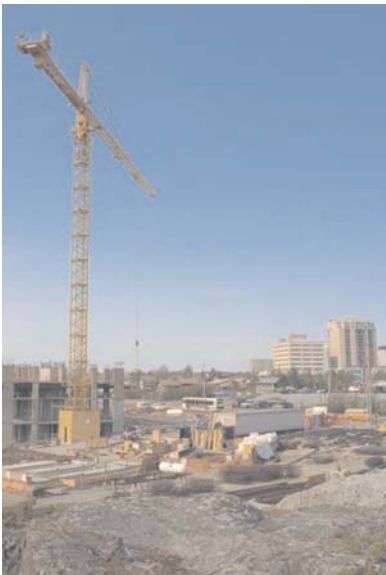
Polar Developments residential tower under construction image: http://www.yellowknife.ca/__shared/assets/Blue_Book5.pdf
