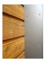
avoid heat dispersal. The total wall thickness is 12 cm. The internal part of the perimeter wall is covered with plywood, resistant to impact and to the external *sollicitations*, to humidity, and it is fire proof. Moreover it could be personalized choosing between one immense applicable finish range: to tempera, enamels, wall paper, according to one's taste. The external part is covered with nailed steel sheets.
