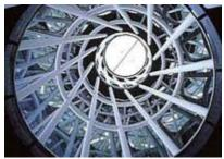
These buildings also carry certain sustainable aspects. In Sendai Mediatheque, the voids created by the circular placement of the tubular columns serve to provide ventilation throughout the building, as well as provide natural lighting into the space. (IMAGE)
