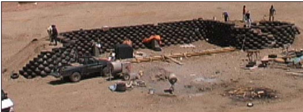
Earthships primarily use recycled and waste materials in their construction. Automobile tires, pop bottles, aluminum cans are just some of the components used in creating the structure of the Earthship. The finishing materials used in the house are made of recycled and reused materials. The carpet is made of
