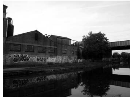
Site from canal
