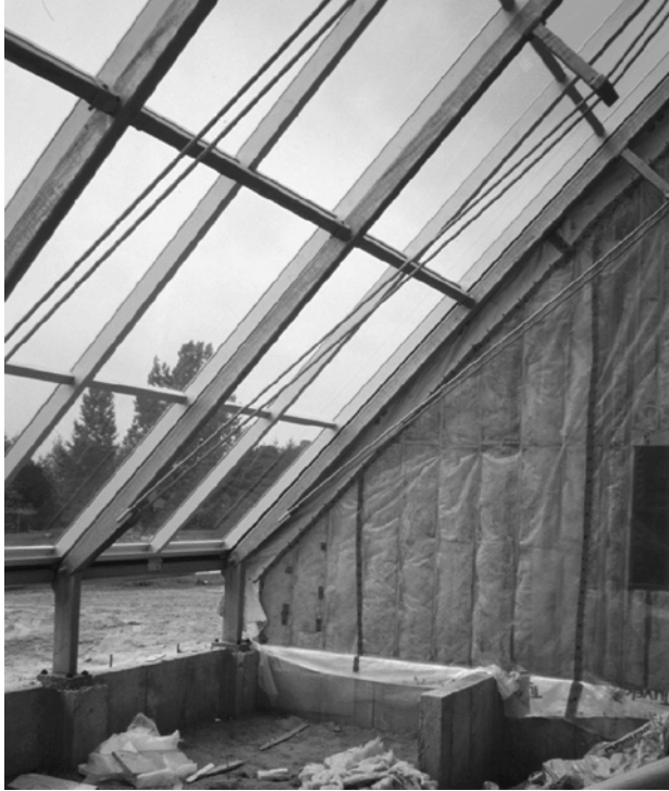
Fig. 4 The Day Center, interior under construction showing triple glazed greenhouse, high insulation levels (6" fiberglass batt inside + 2" rigid polystyrene outside), mass thermal storage in concrete floor
