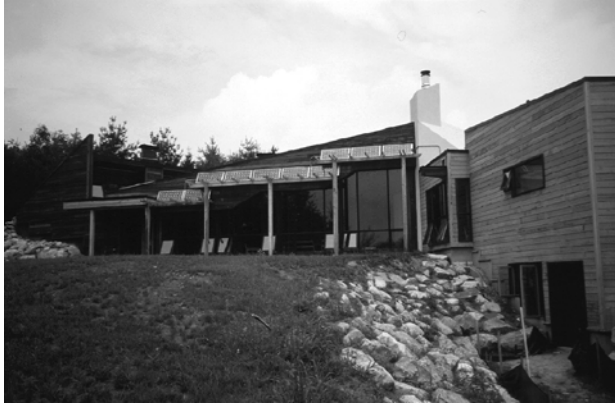
Fig. 1 The Earth Residence, south facade, with trellis sun shades/with PV collectors atop
