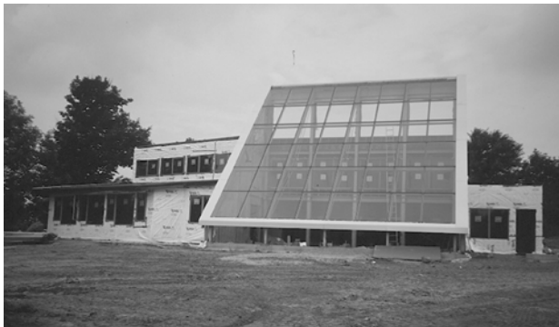
Fig. 3 The Day Center, south elevation
