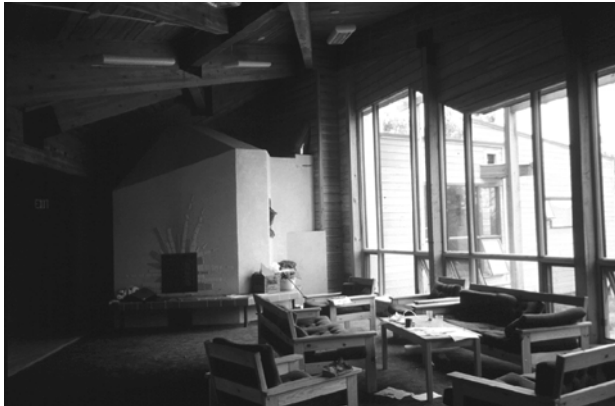
Fig. 2 The Earth Residence, masonry heater which supplements solar heat during the winter months
