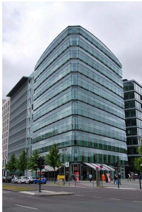
Fig 6: Double façade office building in Berlin, Germany. The exterior glass skin is not sealed and allows for migration of ventilating air to the interior while buffering noise.
