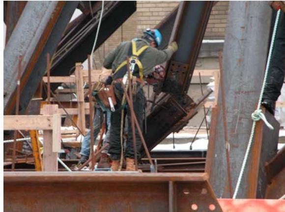
Figure 7: Ironworkers attempt to connect a sloped assemblage of the diagrid
