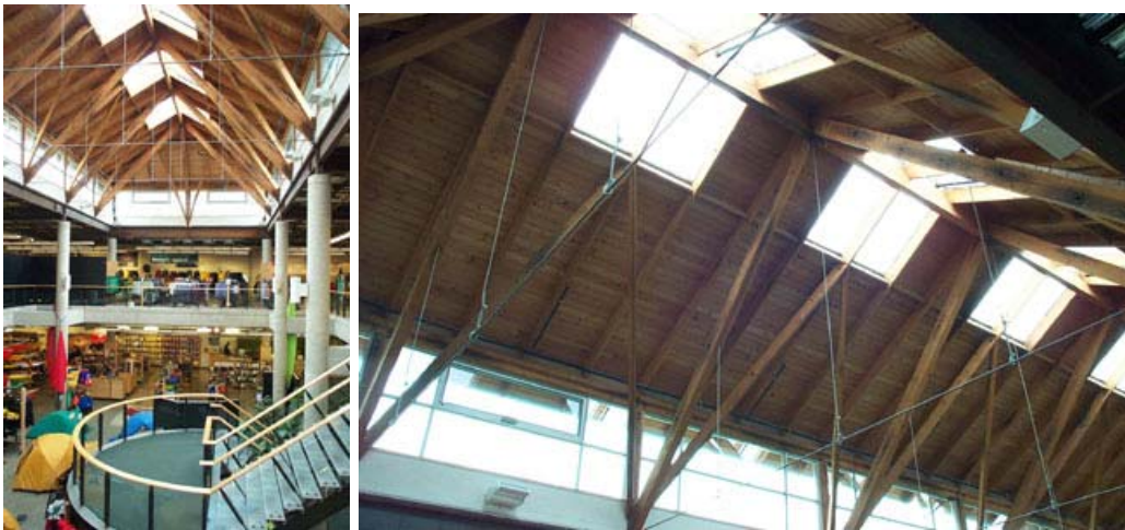
Figure 8: Mountain Equipment Coop, Toronto, Stone Kohn and Vogt Architects Indoor Environmental Quality: Credit 8 Daylighting – use of glazing to daylight the space can increase heat loss (winter) or heat gain (summer) if not properly detailed and specified
