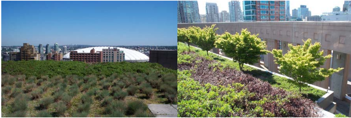
Figure 2: Vancouver Public Library. Moshe Safdie and Associates with Downs Archambault and Partners. Sustainable Sites: Credit 7.2 Landscape & Exterior Design to Reduce Heat Islands (roof)
