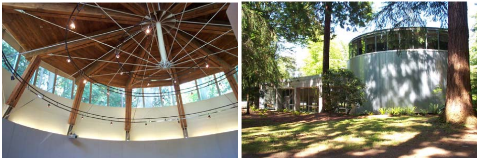
Figure 6: Liu Centre for Asian Studies, UBC, Architectura Materials and Resources: Credit 4 Recycled Content – timber framing. The building also uses flyash in its concrete – a waste product of the steel industry.
