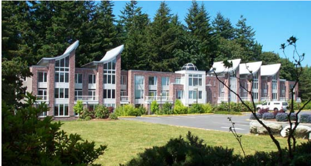
Figure 7: C.K. Choi Institute for Asian Studies, UBC, Matsuaki Wright Architects Materials and Resources: Credit 4 Recycled Content (both the timber frame and brick veneer cladding) Reuse of brick for cladding can bring concerns regarding the “life left” of the product from the point of view of durability and weathering.
