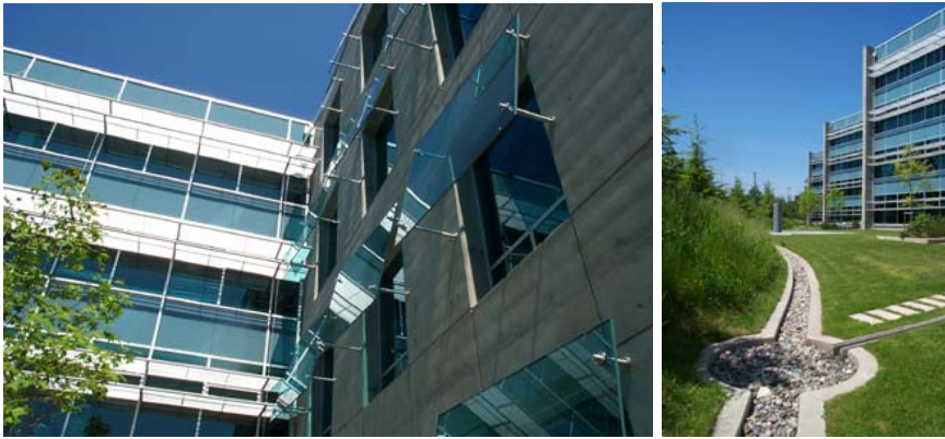
Figure 5: BC Gas (Terasan Gas) Musson, Cattell Mackey Partnership Energy Efficiency: Prereq 2: Minimum Energy Performance: Solar shading to reduce energy consumption. Differentiated façade strategies as a function of orientation.
