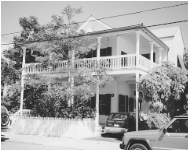
Fig. 4 Eaves and porches Roof overhangs have long been used to keep buildings cool in warm climates. The trees help, also.
