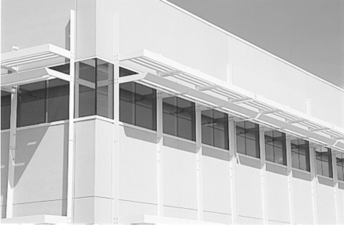
Fig. 8 Shadow pattern of horizontal louvers These are working well, except at the corner. We infer that the wall at right faces in a southerly direction. A double row of louvers is used to reduce the outward distance required. The louvers are attached to vertical stringers, which are bolted to the wall.
