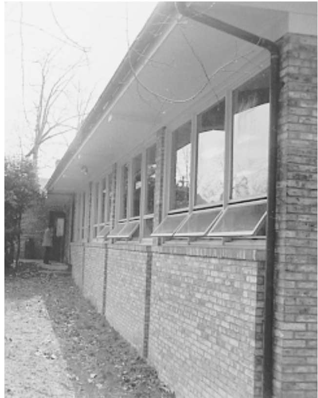
Fig. 5 Roof overhang The shadow pattern shows that the roof overhang of this library is effective in keeping direct sunlight out of the windows. The open windows show that natural ventilation is cooling the building, assuming that the air conditioning has been turned off.
