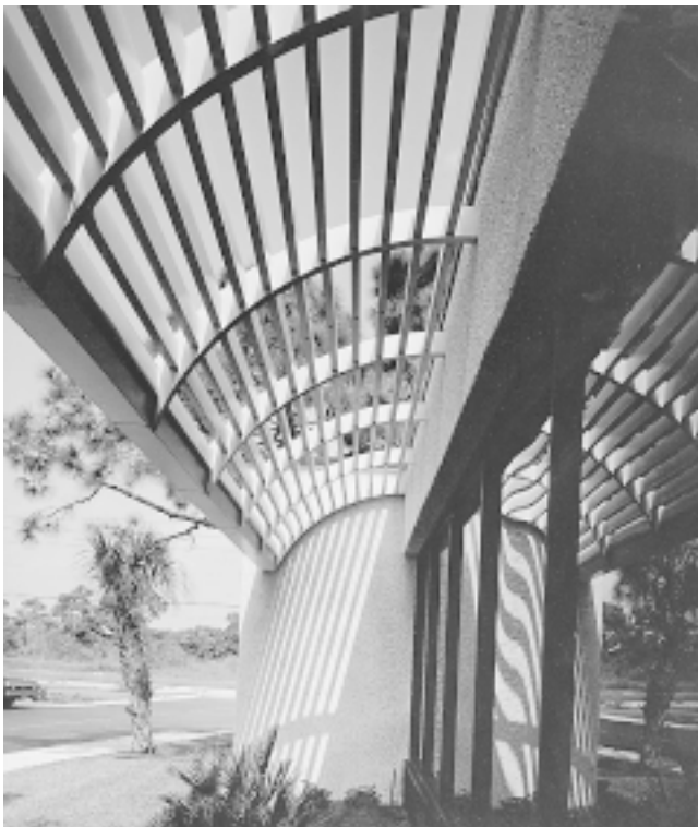
Fig. 13 Louvers arranged in a curved array The curvature is strictly for appearance. The designer has to work a little harder to figure out the louver dimensions that keep direct sunlight from striking the window.
