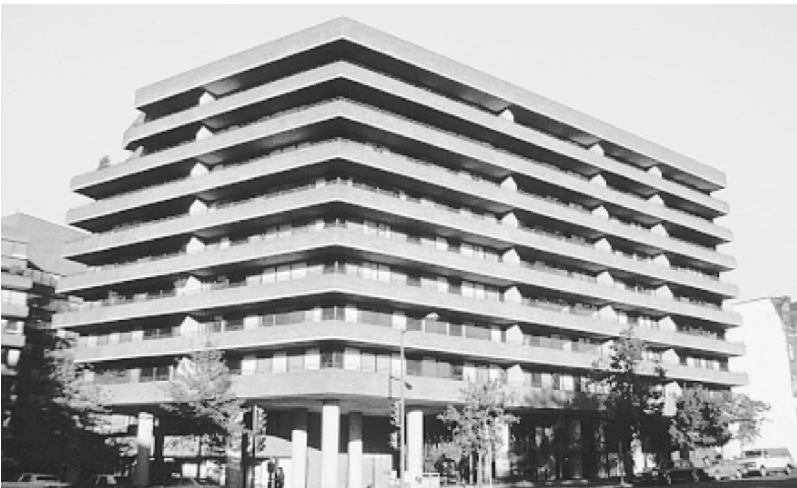
Fig. 1 Horizontal shelves These can be every effective for reducing cooling load on the south side of a building. As seen here, sunlight gets under the shelves on other orientations. These also serve as balconies, a nice touch that is rare in office buildings. They make window washing much easier, protect the glazing, and protect the surroundings from falling glass.
