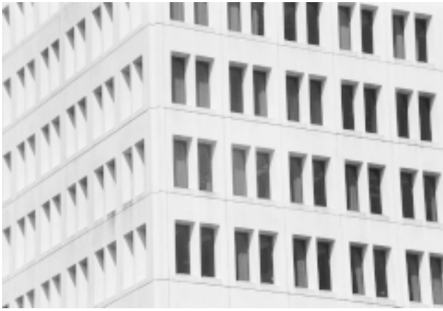
Fig. 6 Inset windows The shadow patterns show that deeply inset windows reduces solar heat gain. However, it cannot create satisfactory daylighting by itself.
