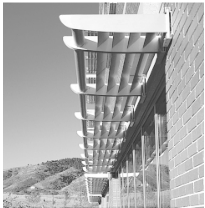
Fig. 14 Shading louvers attached to wall by brackets
