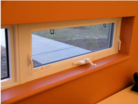
Credit 1.1: Optimize energy Performance - Thermally broken windows with fiberglass frames
