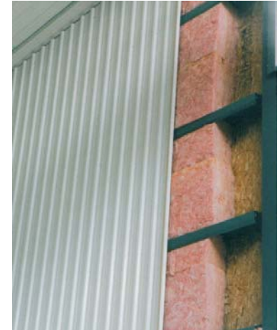
Credit 1.1: Optimize energy Performance - EIFS system combined with batt insulation to reduce thermal bridging
