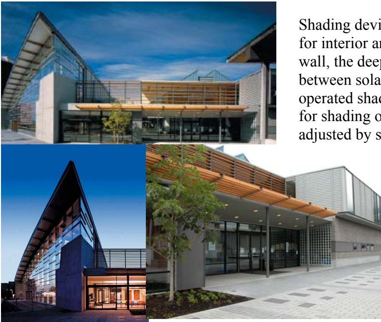
Southeast and East Shading Devices
