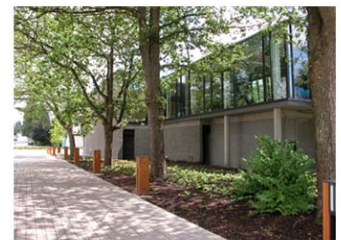
View to existing mature trees
