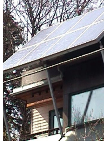
Figures 4, 5 and 6: Details of the photovoltaic panels that shade both the exterior balconies and south facade of the building from excess solar gain in the summer.
