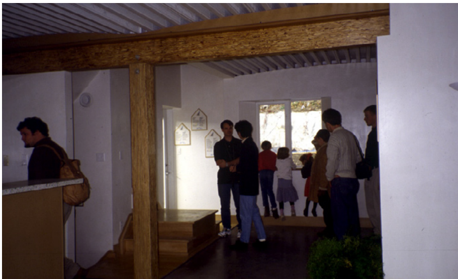
Figure 23: Interior finishes are kept to a minimum, leaving all finishes exposed.
