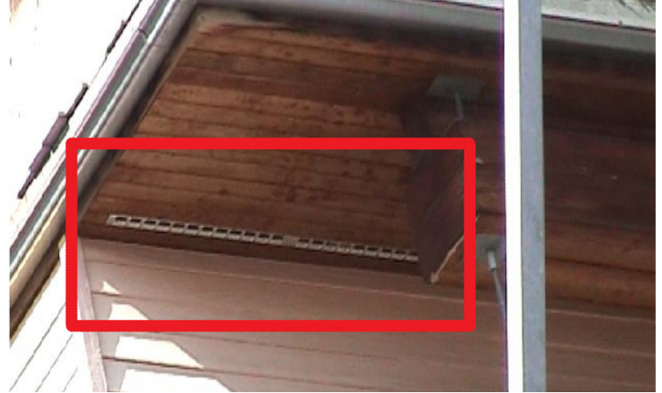
Figure 8 (Above): Aside from operable windows, vents subtly located in soffits and along wall faces. Figure 9 (Below): Living spaces are filled with natural daylight.
