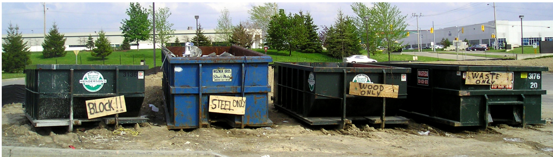
Figure 16 (Below): View of the recycling system implemented during construction.
