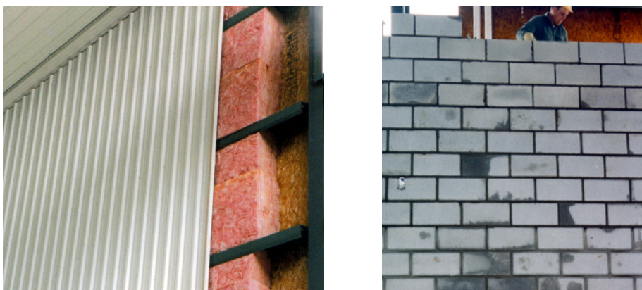
Figure 21 (Above Left): View of wall system in garage area. Figure 22 (Above Right): A concrete block wall is the fire separation between the two halves of the building. Figure 23 (Below): Section of the added insulation at the EIFS portion of the wall.
