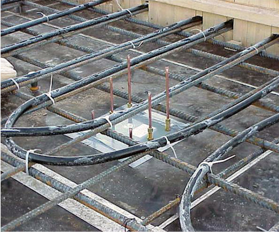
Above: Details of pipes being attached to the concrete reinforcing. Right: Zone valve controls. Below: Conceptual schematic of pipe placement in slab.
