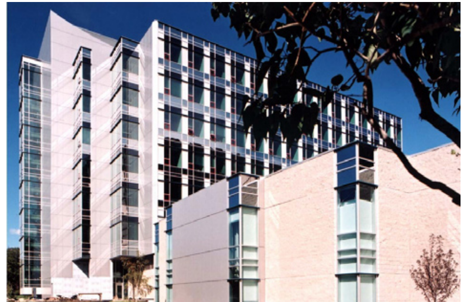
North-west corner of the University of Calgary ICT Building
