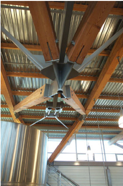
Figures 27, 28, and 29 (Above Left, Above Right, and Below Left, respectively): Details of the steel and glulam trusses. Figure 30 (Below Right): Detail of barrel cellar.
