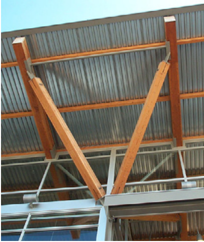
Figures 27, 28, and 29 (Above Left, Above Right, and Below Left, respectively): Details of the steel and glulam trusses. Figure 30 (Below Right): Detail of barrel cellar.
