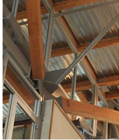
Figures 27, 28, and 29 (Above Left, Above Right, and Below Left, respectively): Details of the steel and glulam trusses. Figure 30 (Below Right): Detail of barrel cellar.
