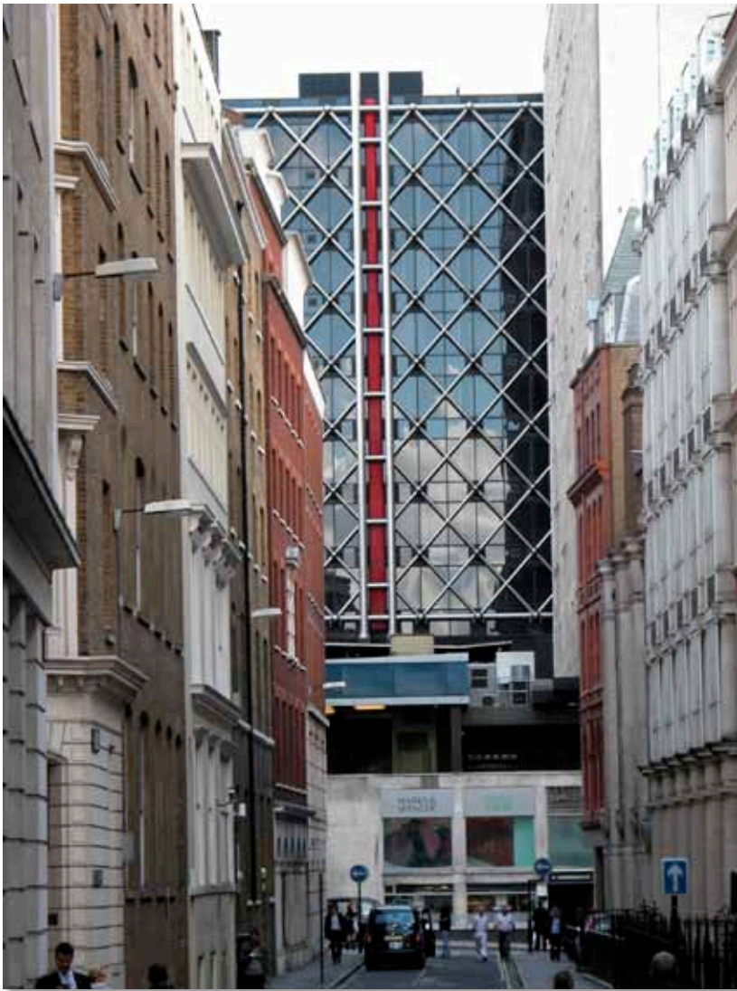
Bush Lane House, London: stainless steel exterior tube structure filled with water
